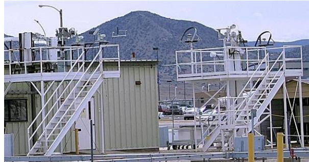
Fig. 1. Weather station at Sandia's PSEL
