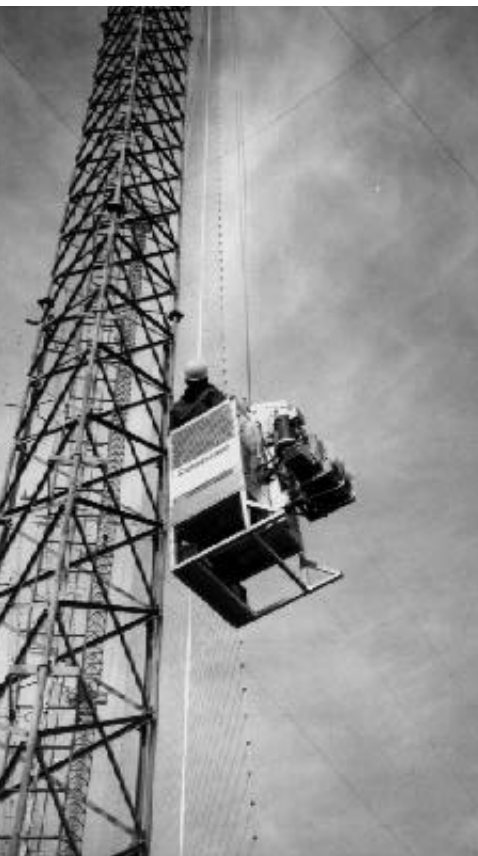
Rigger maintains shortwave antenna using an IBB-designed cage.
