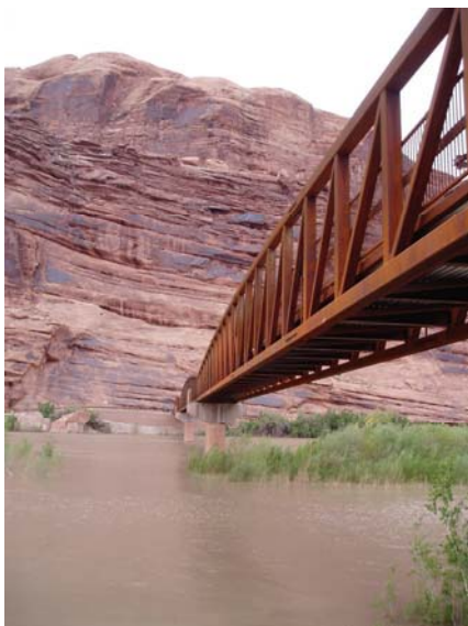
Figure 36: Colorado River Bicycle/Pedestrian Bridge.
