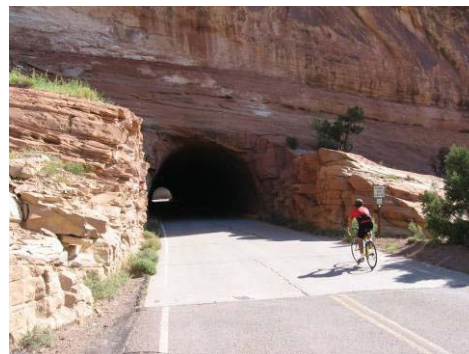
Tunnel at Colorado National Monument (Photo courtesy Phil Akers.)
