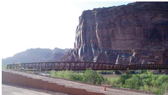
Figure 26: Colorado River Bicycle/Pedestrian Bridge. (Photo courtesy Rebecca Gleason.)
