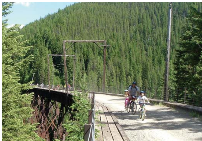
Figure 23: Route of the Hiawatha Railroad Trestle. (Photo courtesy Kate Ciari.)
