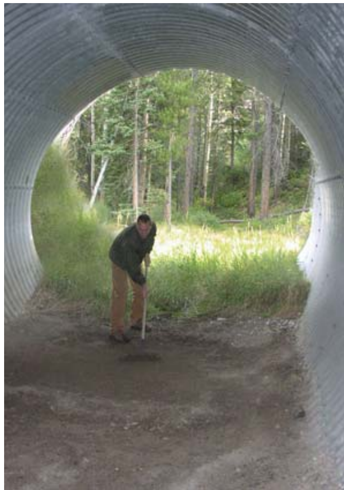
Figure 76. Photo. Raking of track bed in culvert Banff National Park, Alberta (Credit: Tony Clevenger/WTI).
