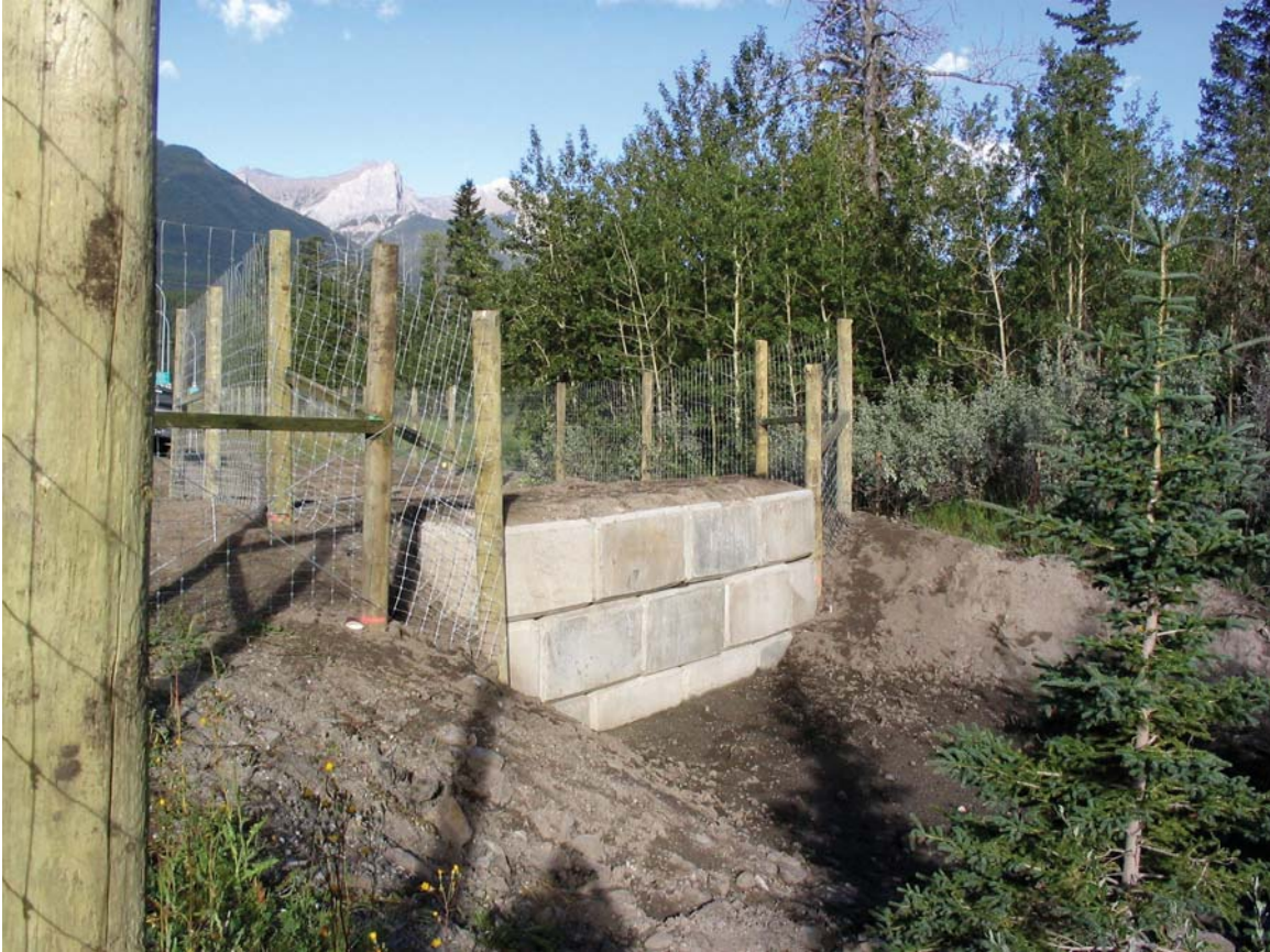
Figure 71. Photo. Escape ramp (jump-out) for wildlife trapped inside highway right-of-way (Credit: Tony Clevenger).
