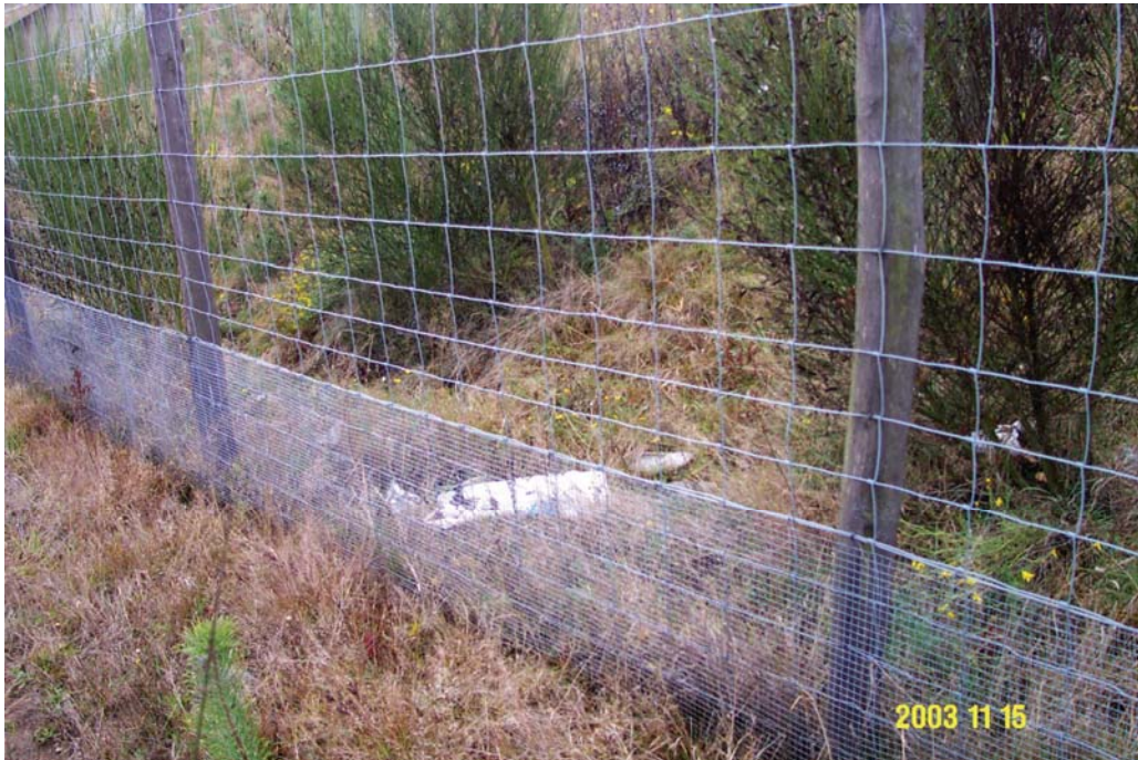
Figure 70. Photo. Small and medium-sized mammal fence material spliced to large mammal fence material (Credit: Nancy Newhouse).
