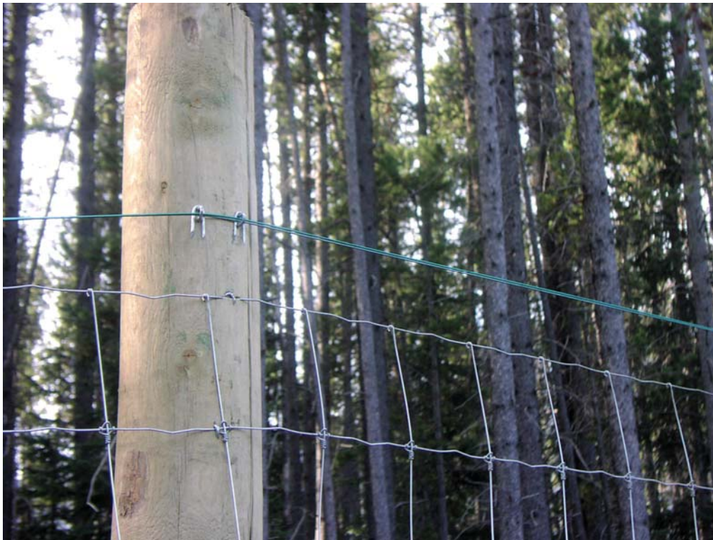
Figure 67. Photo. High tensile cable designed to break fall of trees onto fence material (Credit: Tony Clevenger).
