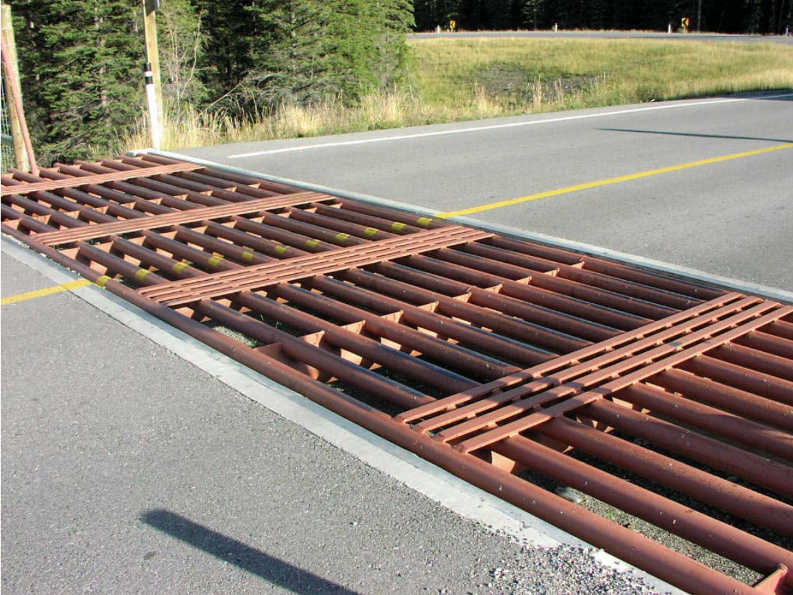
Figure 63. Photo. Cattle guard (Texas gate) in road (Credit: Tony Clevenger).
