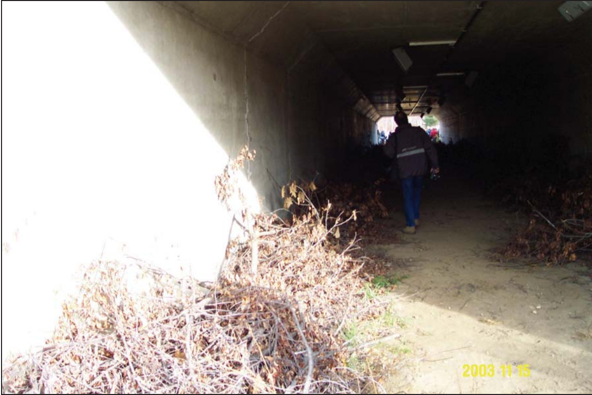
Figure 44. Photo. Brush and root wads placed along underpass wall to provide cover for mammals (Credit: Nancy Newhouse).
