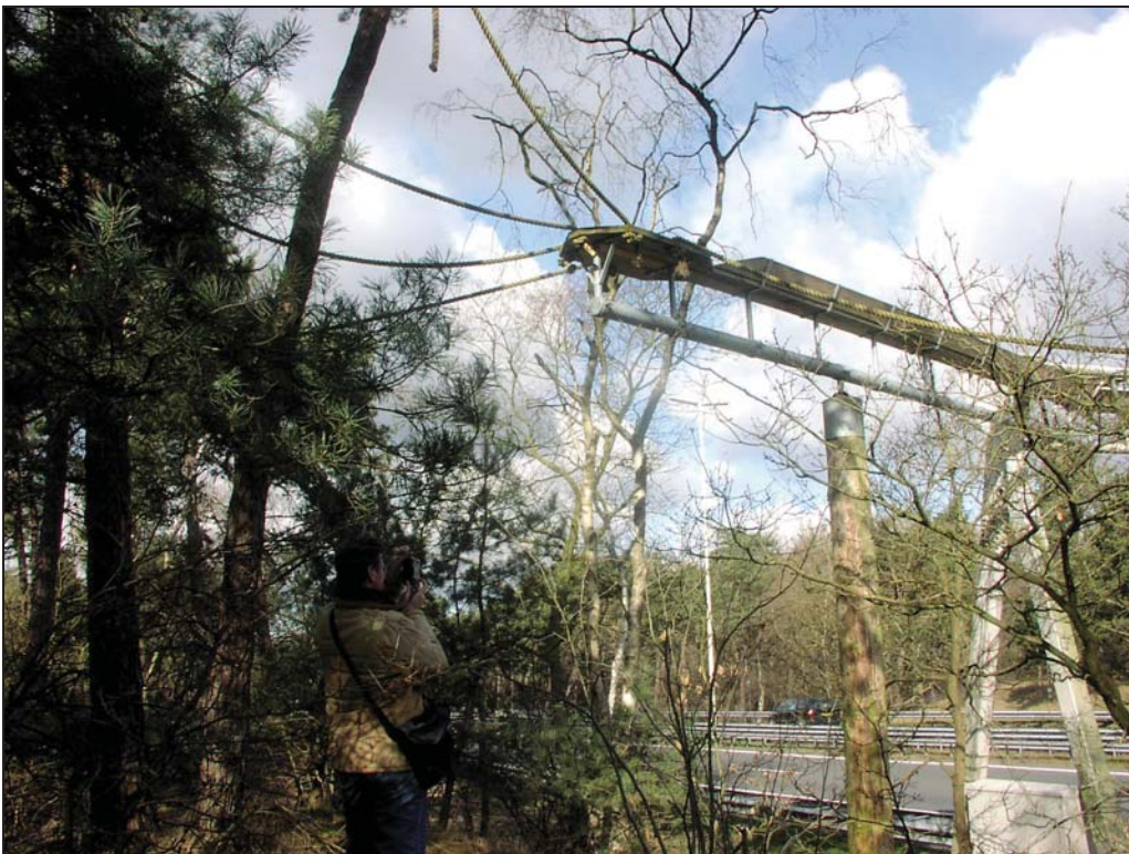
Figure 38. Photo. Ropes extending out from canopy crossing to forest canopy (Credit: Tony Clevenger).
