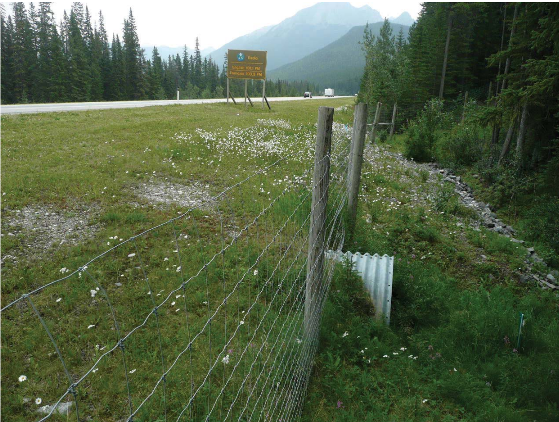
Figure 62. Photo. Wildlife exclusion fencing and culvert design wildlife underpass (Credit: Tony Clevenger).
