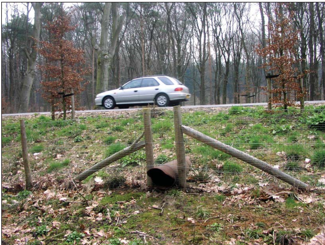
Figure 52. Photo. Badger tunnel in The Netherlands (Credit: Tony Clevenger).
