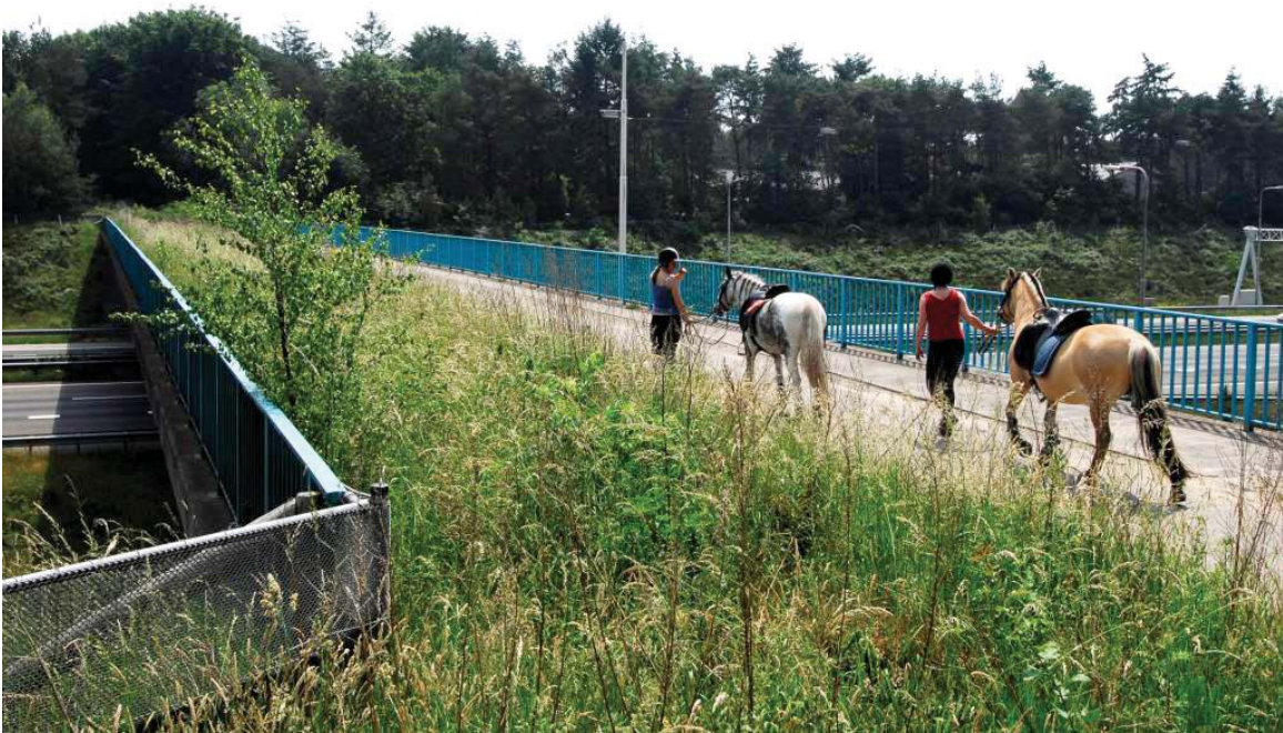
Figure 36. Photo. Human use lane and vegetated strip on multi-use overpass (Credit: Marcel Huijser).
