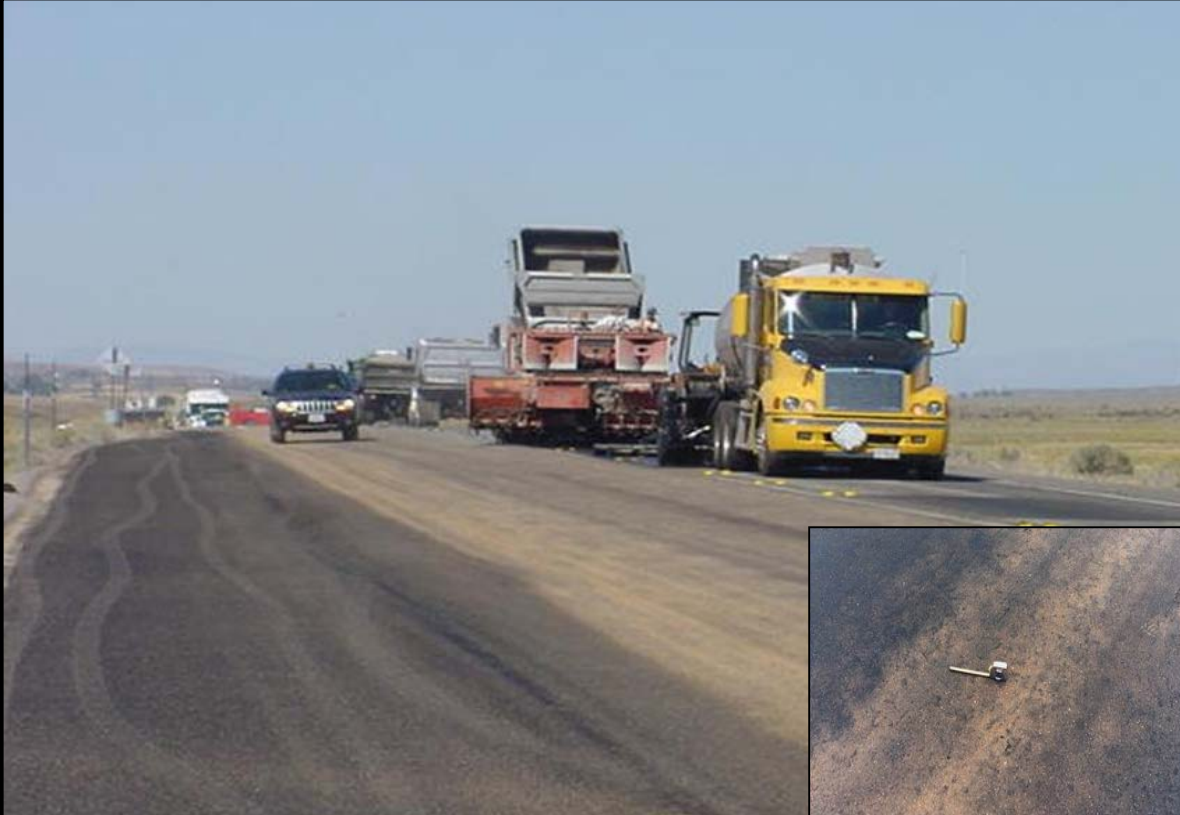
Sand seal construction.
