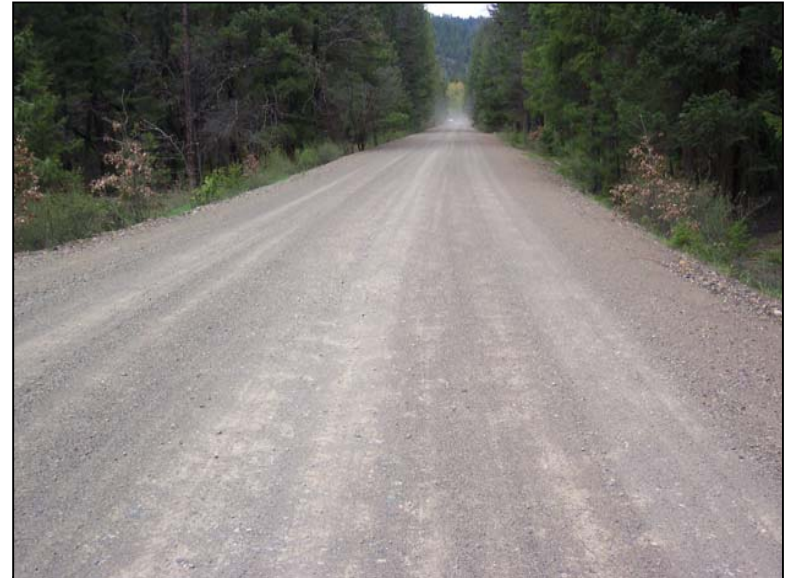
Unbound crushed gravel surfacing.
