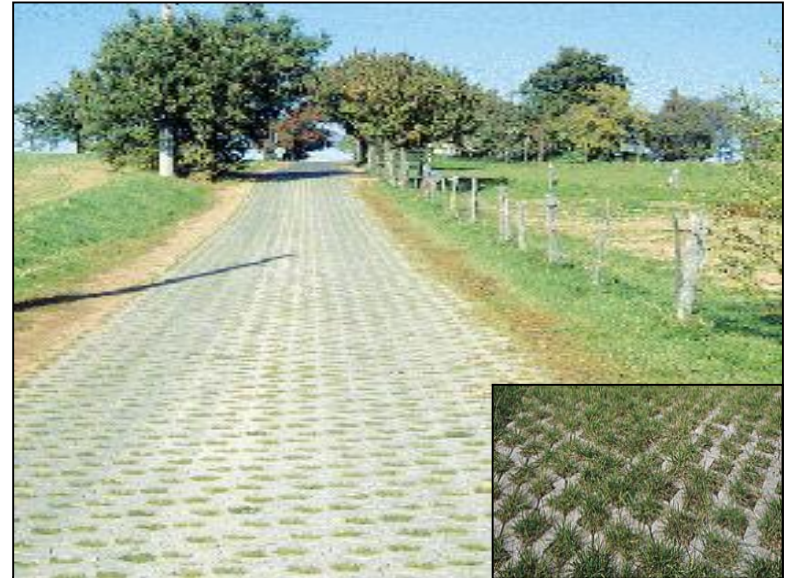
Porous unit paver surfacing.
