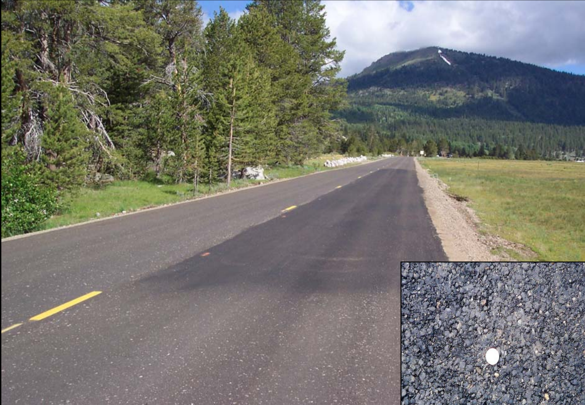
Cold in-place recycled material.
