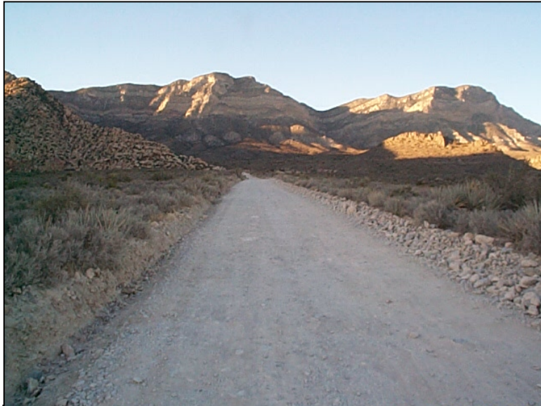
Unbound crushed gravel surfacing.
