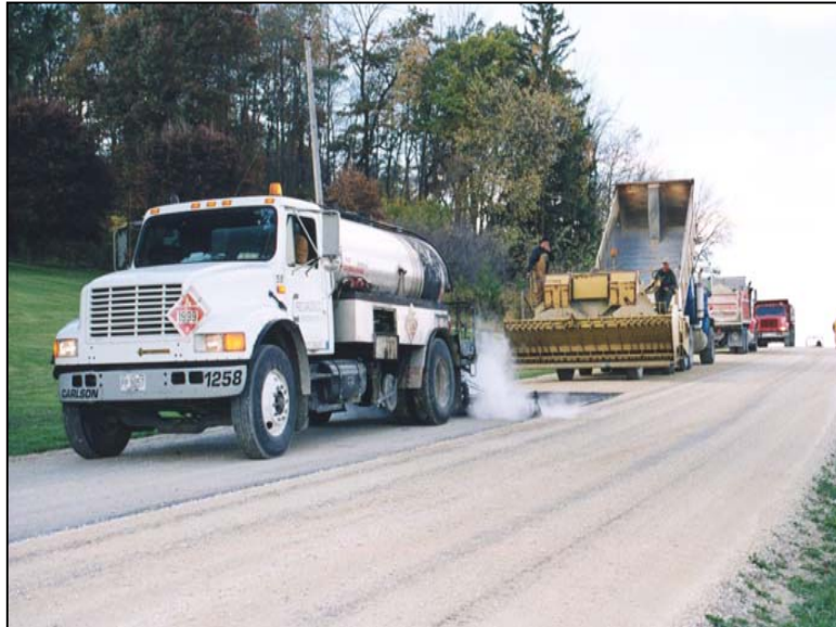
Otta seal construction.
