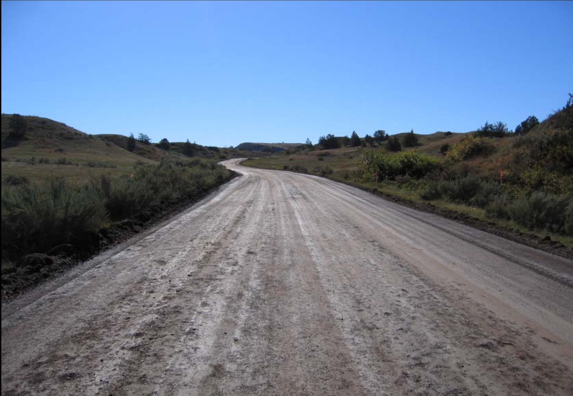
FDR with cementitious stabilization additive.
