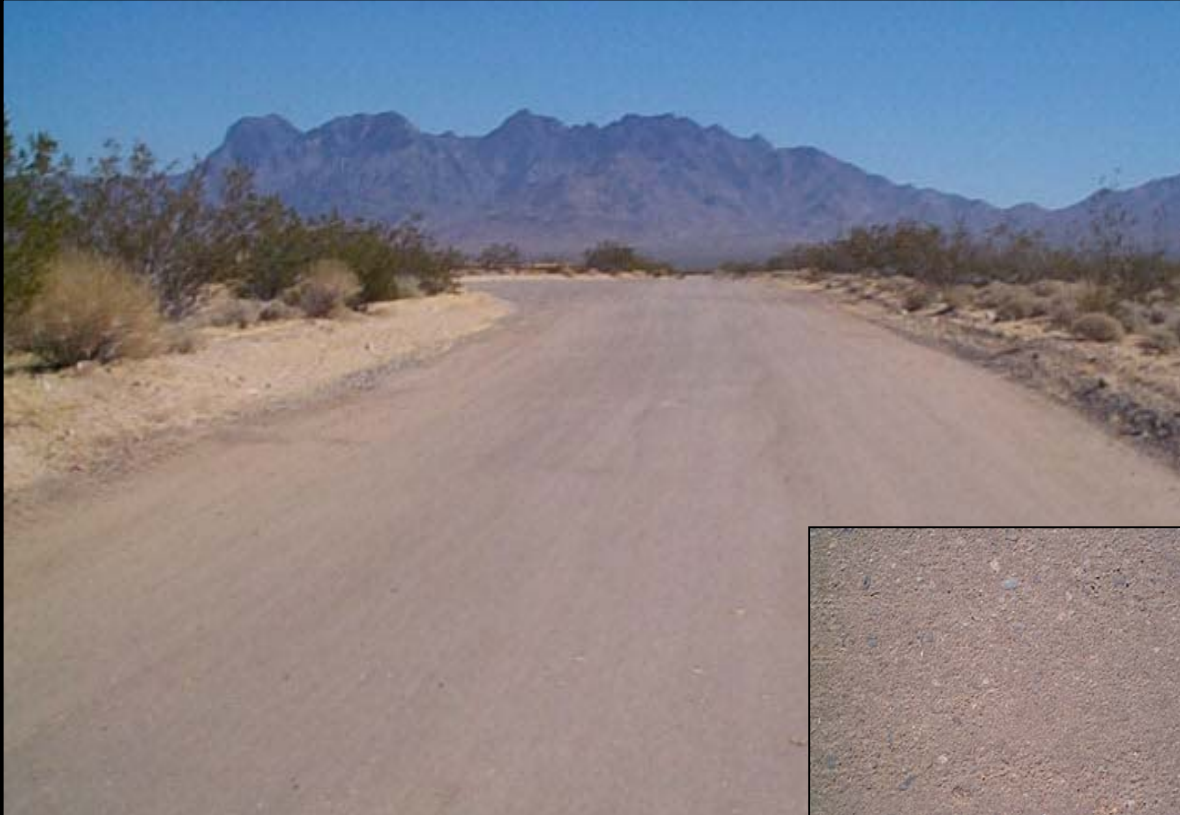
Synthetic polymer emulsion stabilized roadway.
