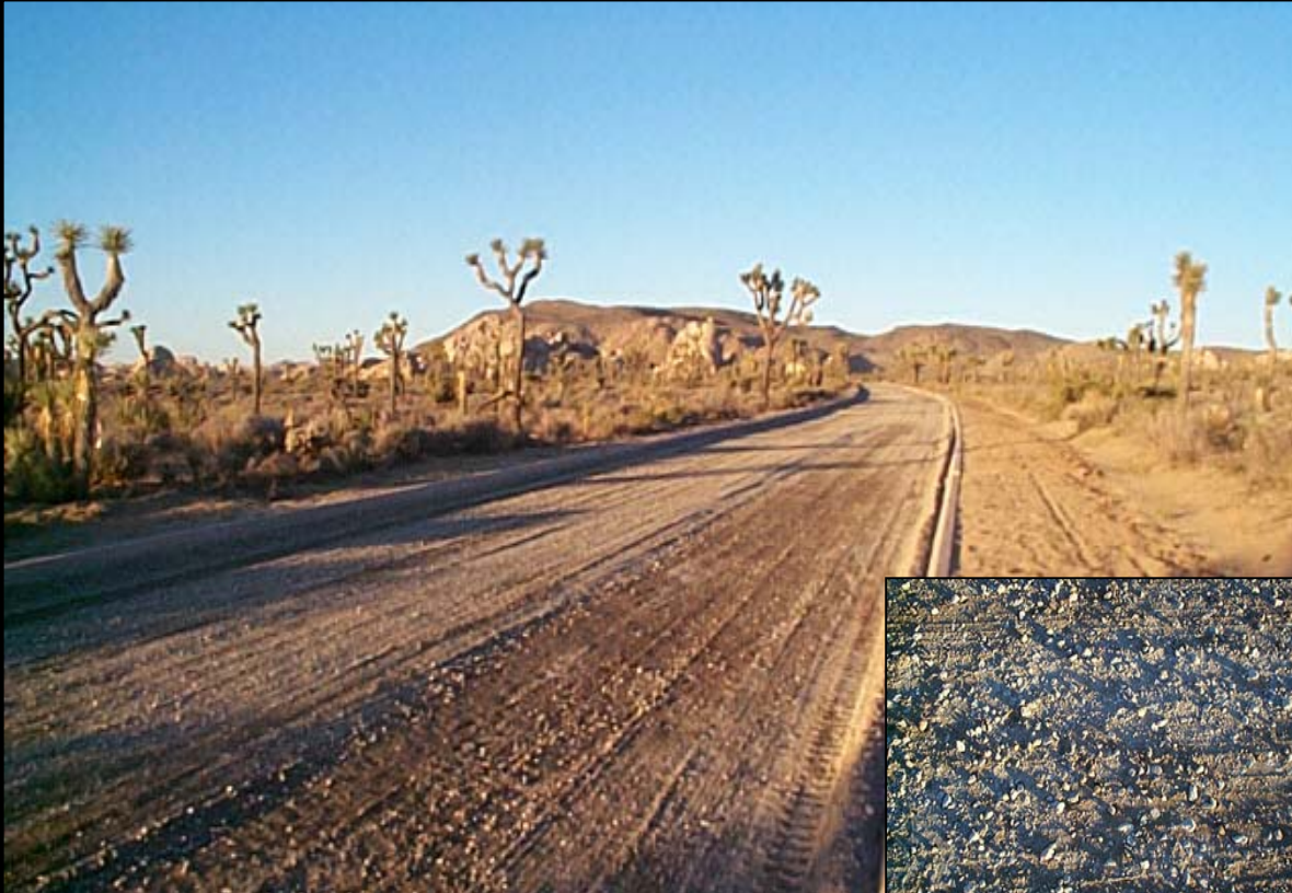
Portland cement stabilized base material.
