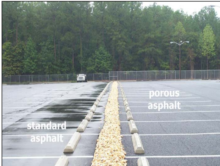
Porous HACP parking lot.
