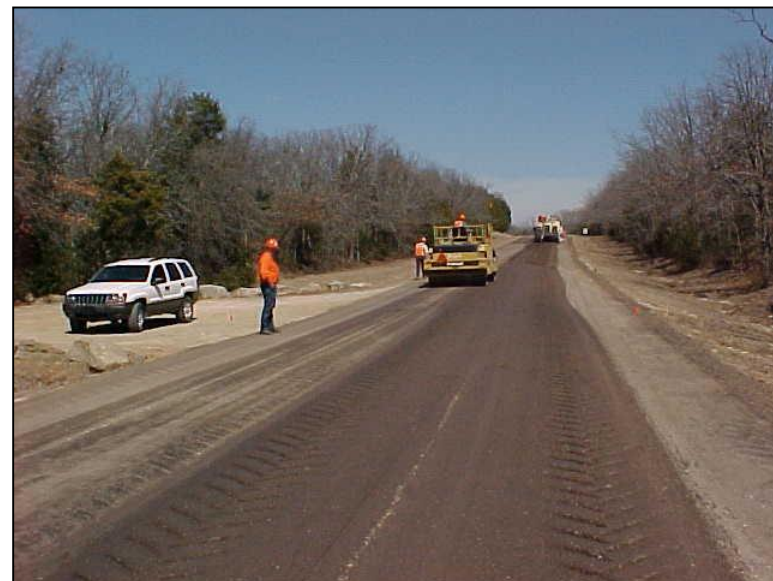
Compaction of FDR-emulsified asphalt material.
