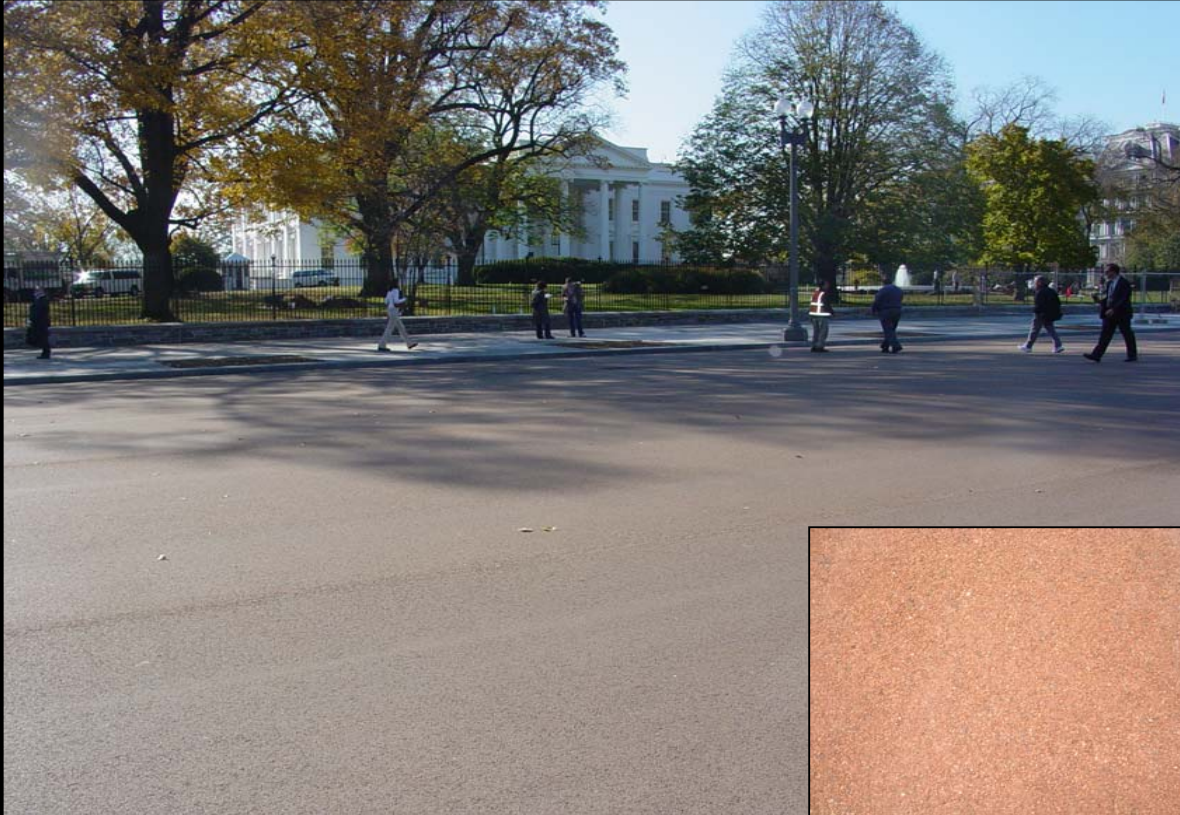
Synthetic binder concrete pavement roadway surfacing.
