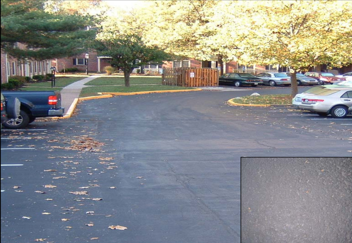
Fog seal surfacing.
