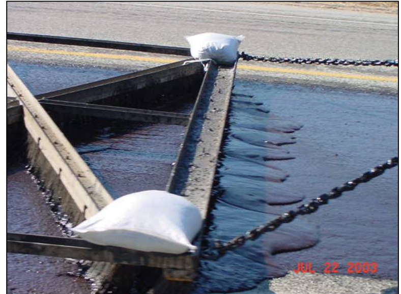
Scrub broom used in construction process.
