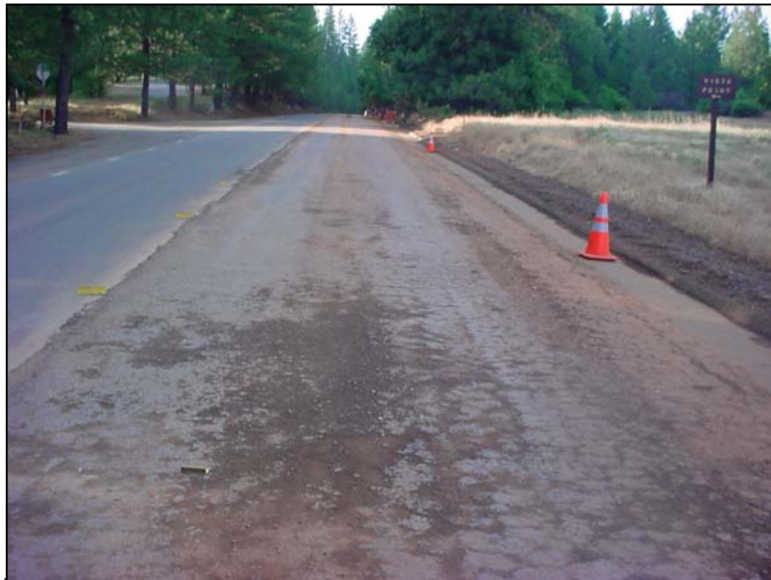
Foamed asphalt material in right lane.
