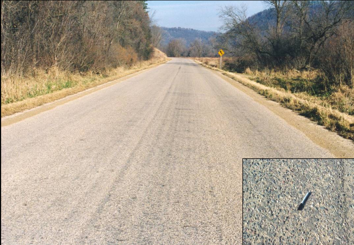
Otta seal roadway surfacing.
