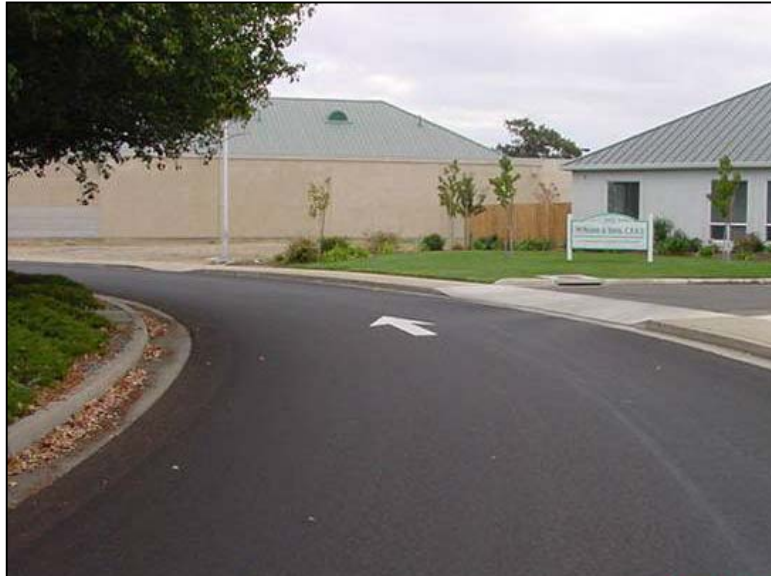
Cape seal surfacing.
