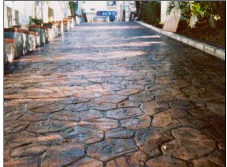
Stamped PCCP surfacing.
