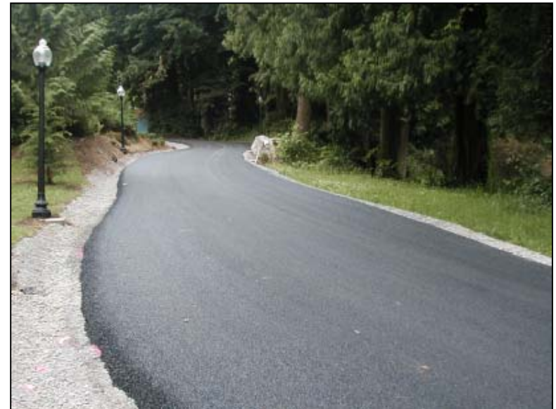
Porous HACP roadway.
