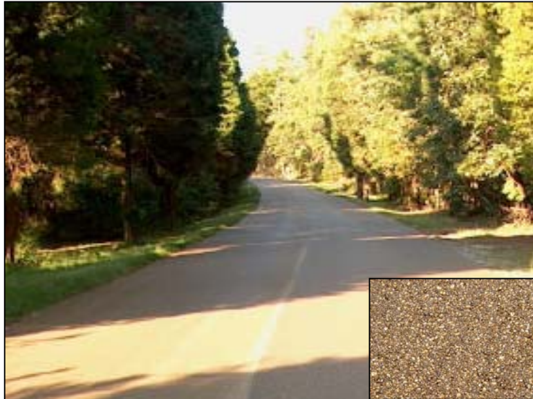
Synthetic binder concrete pavement surfacing.
