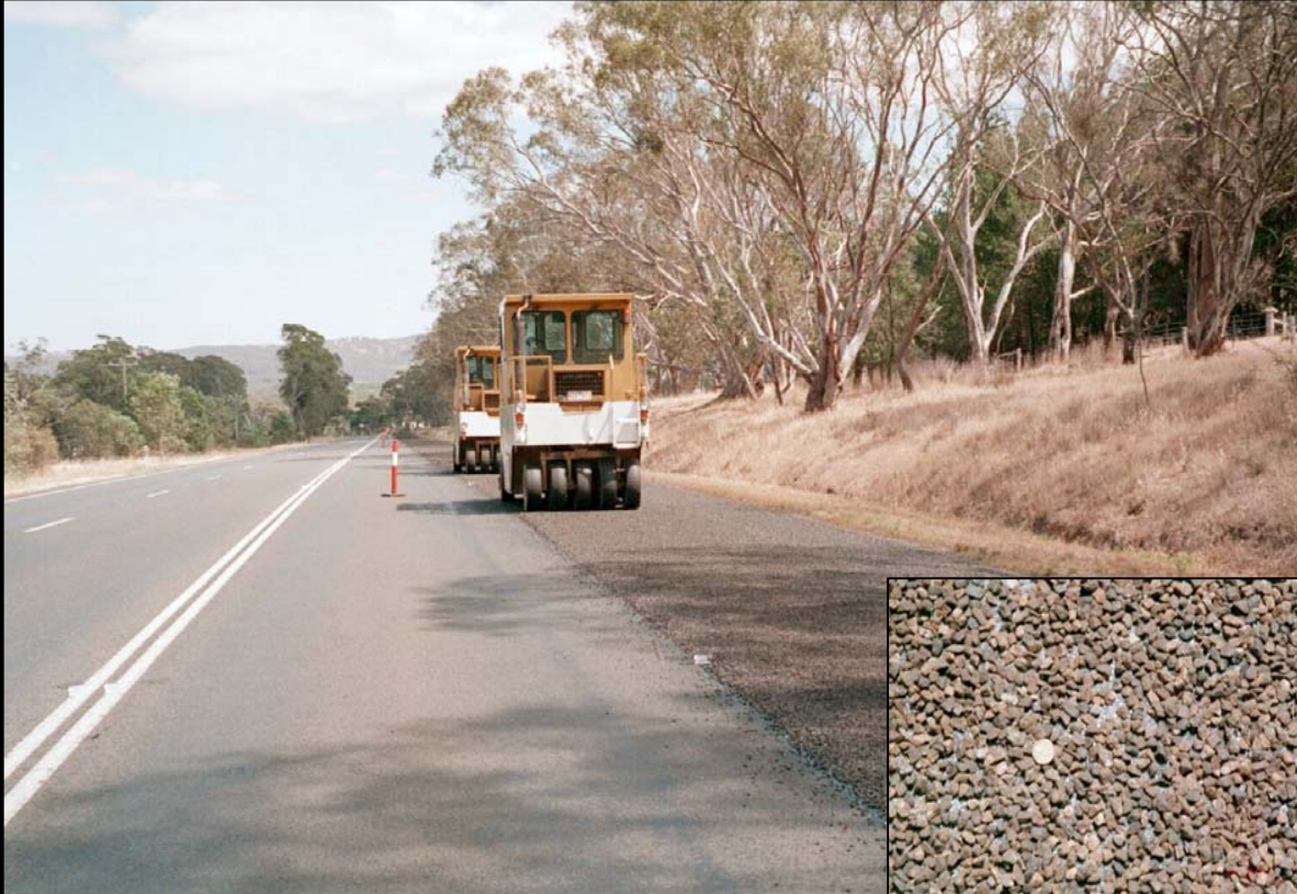
Chip seal over geotextile construction.
