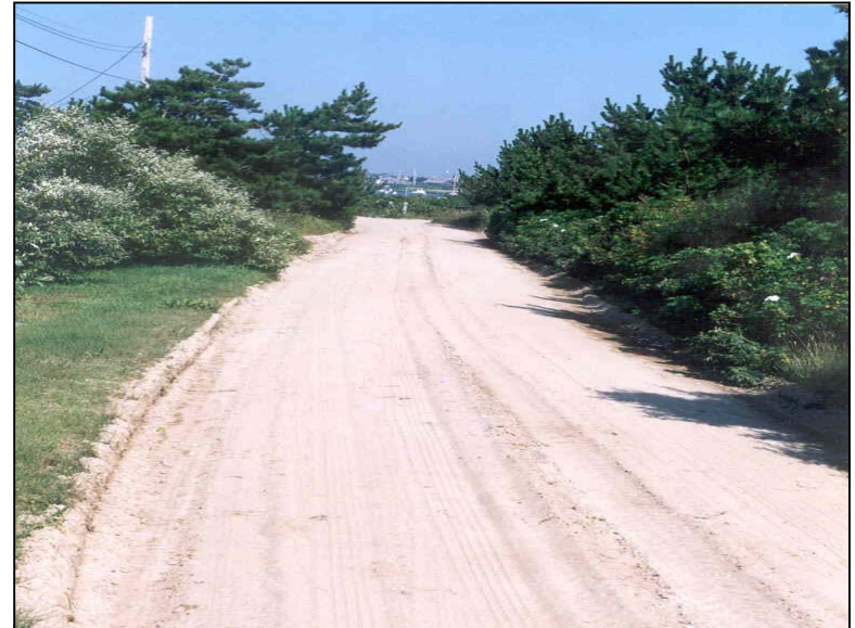
Sand roadway surfacing.
