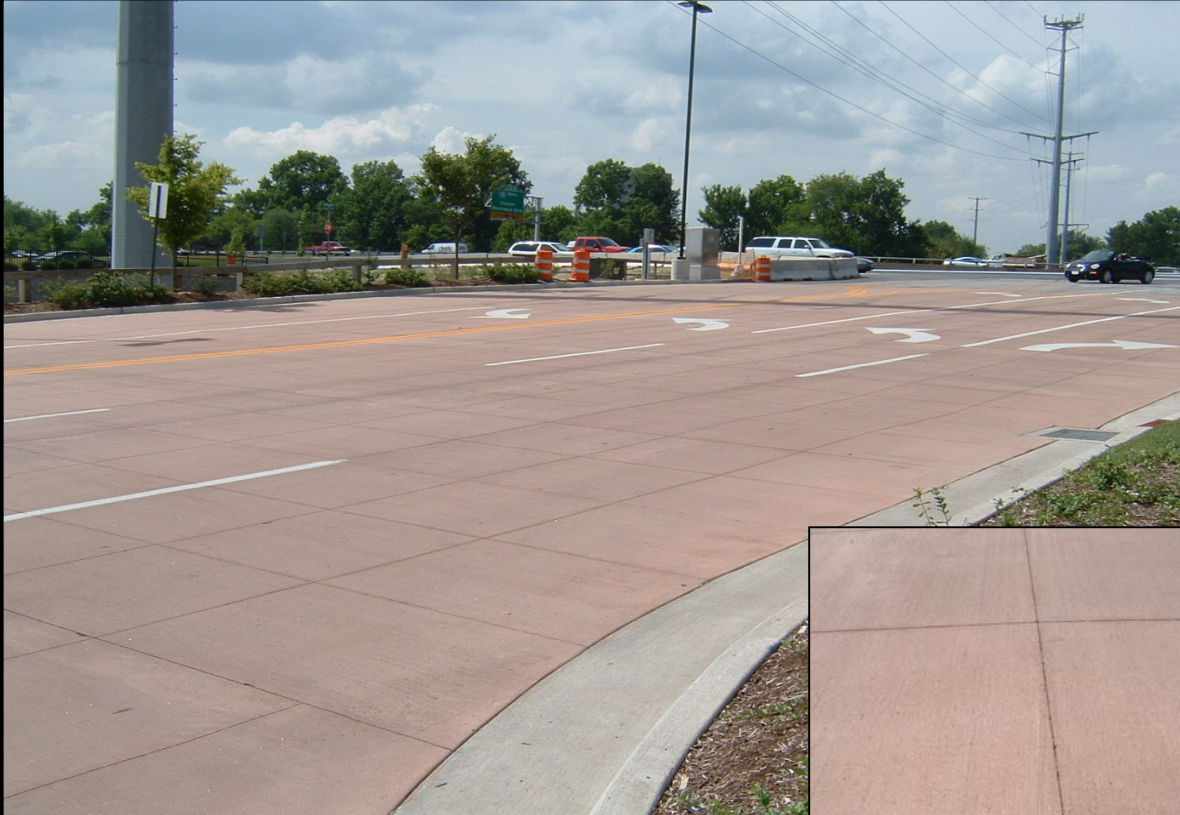
Portland cement concrete pavement roadway.
