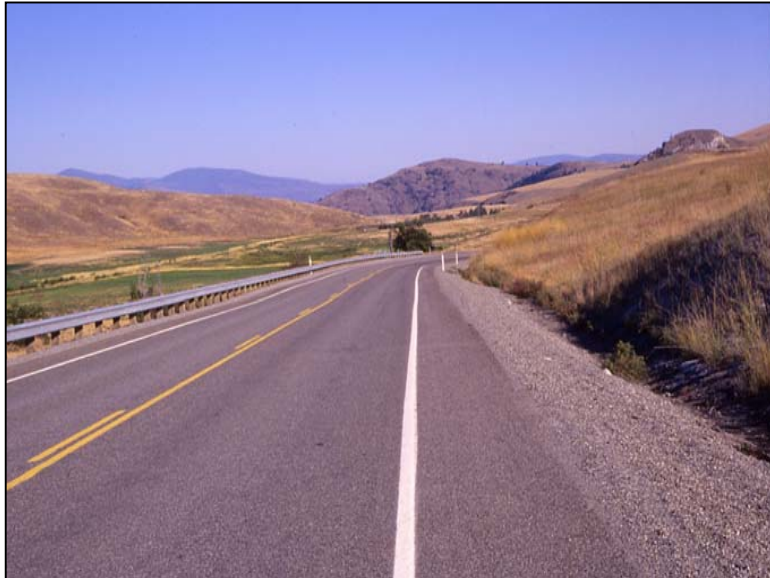
Triple chip seal surfacing.
