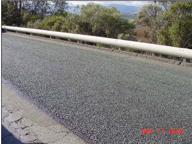
Scrub seal surfacing.
