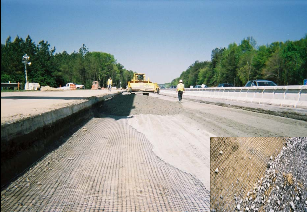
Spreading aggregate base over geogrid layer.
