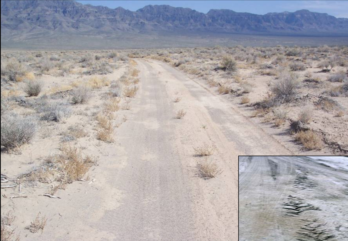
Sand roadway surfacing.
