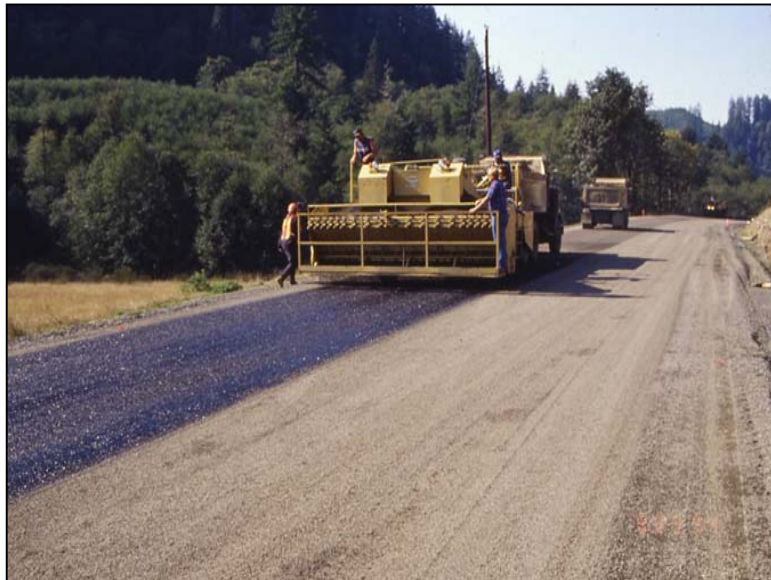
Chip seal construction.
