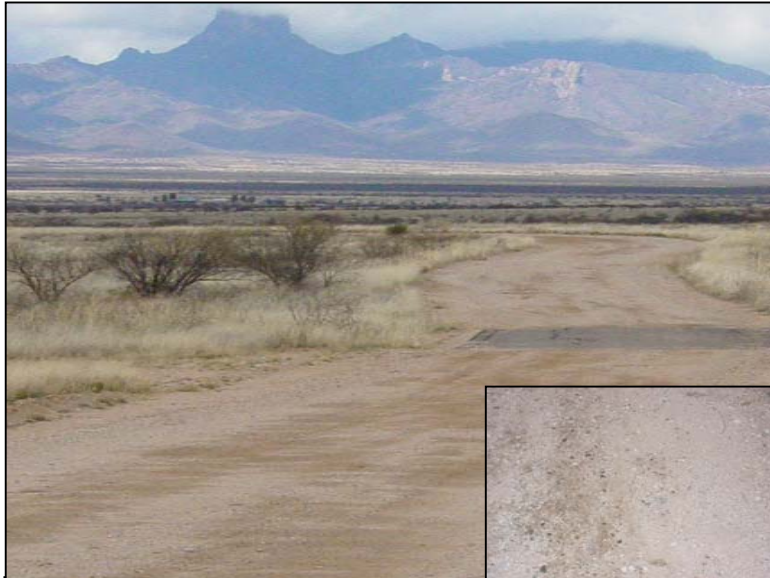
Gravel surfacing treated with MgCl.
