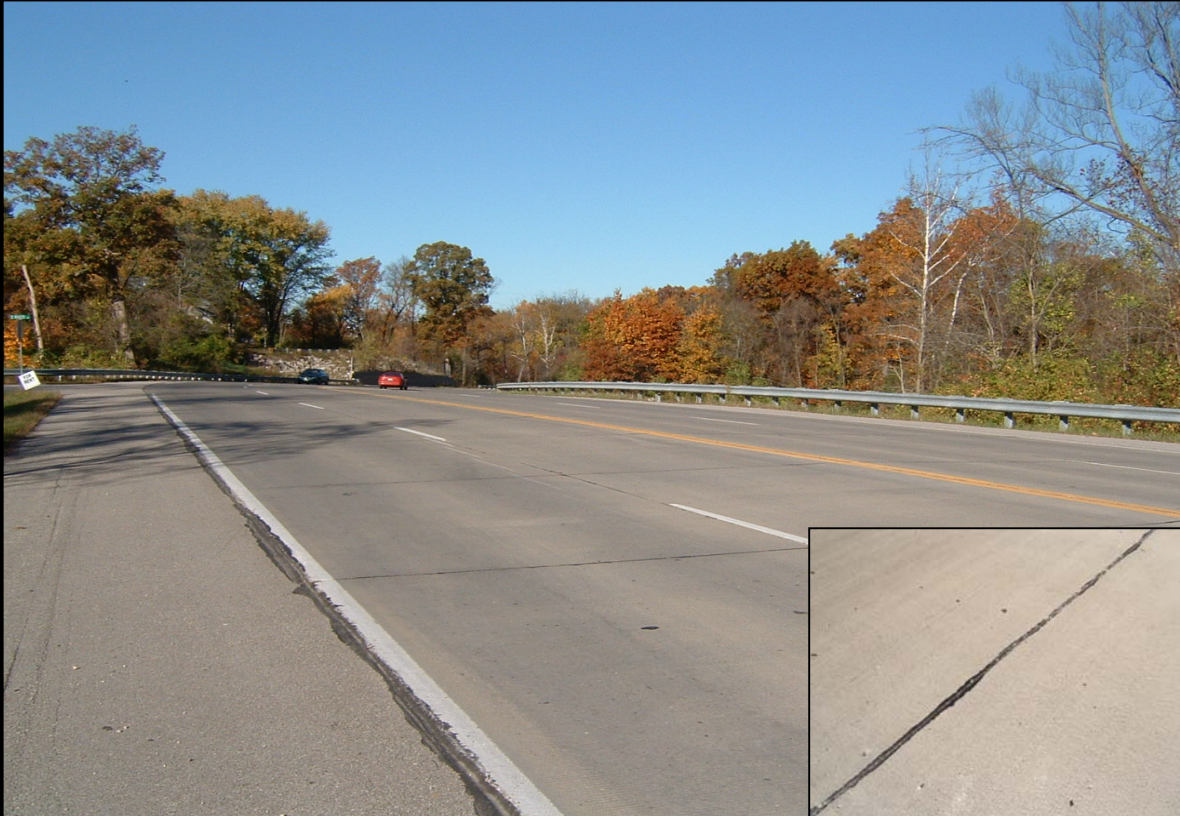
Portland cement concrete pavement roadway.
