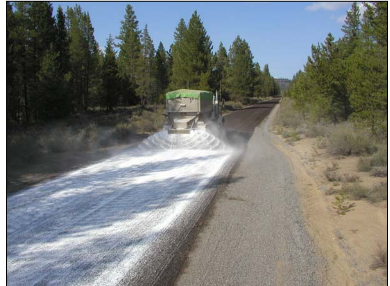
Application of chloride treatment.
