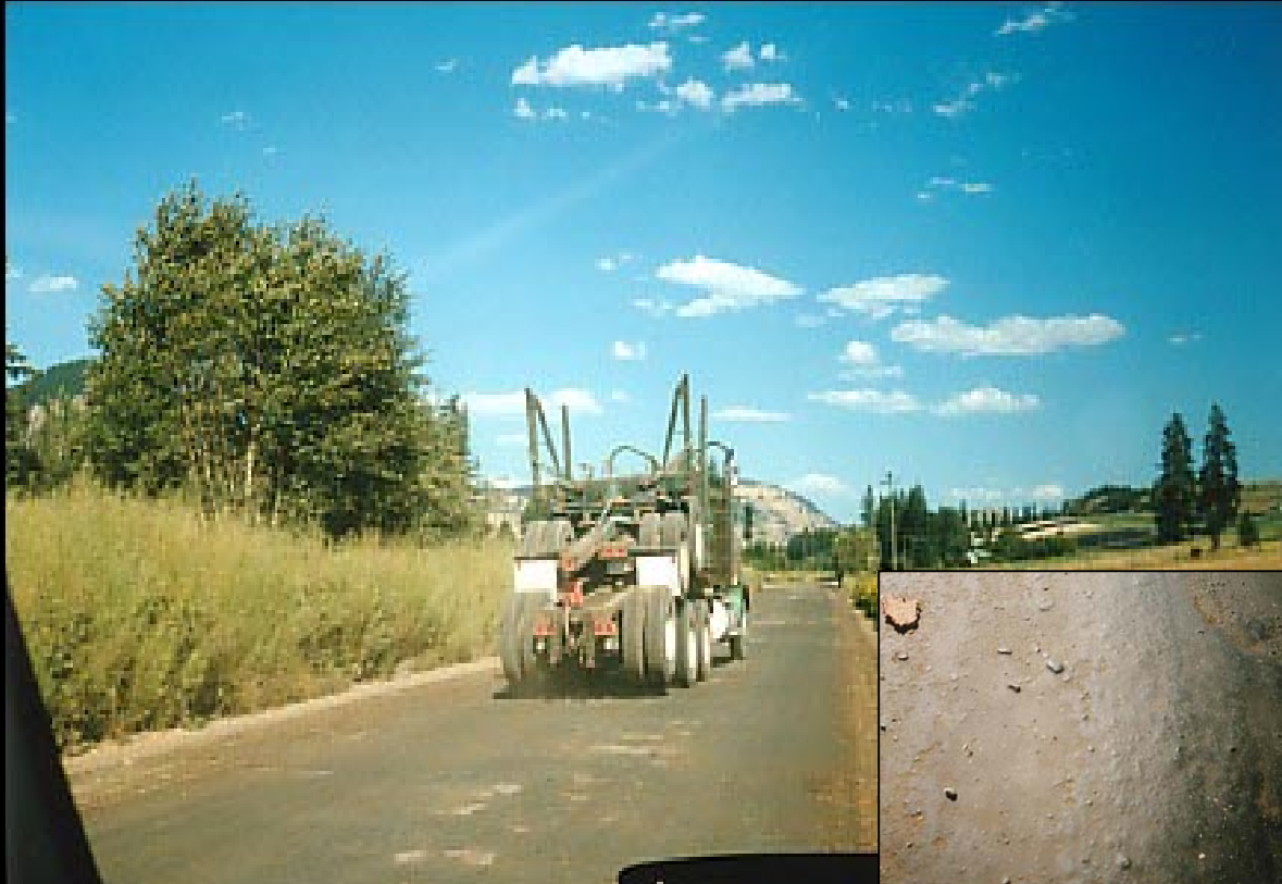
Organic petroleum emulsion stabilized surfacing.
