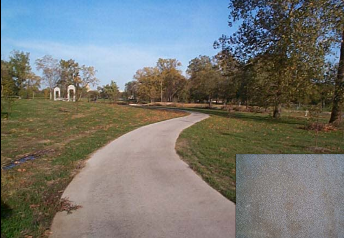
Tree resin emulsion stabilized gravel.
