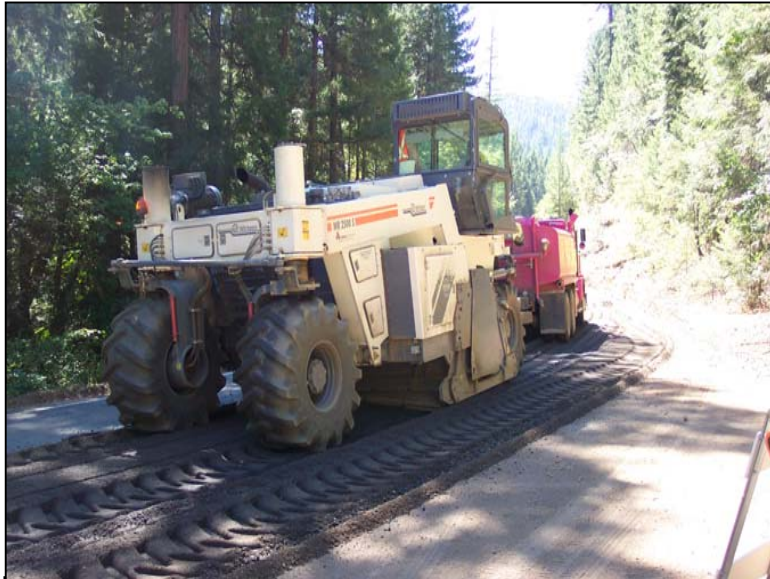
Pulverization process.
