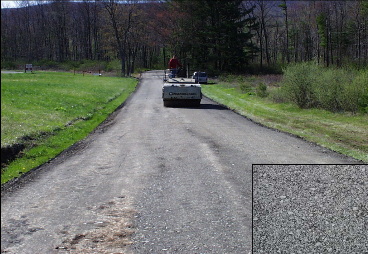
Compacted FDR-emulsified asphalt material.
