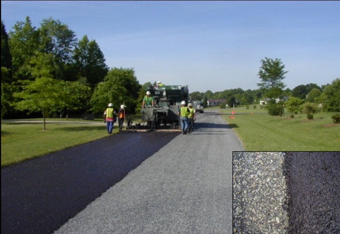
Cape seal construction.
