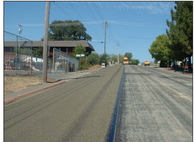
Finished chip seal over geotextile surfacing on left lane
