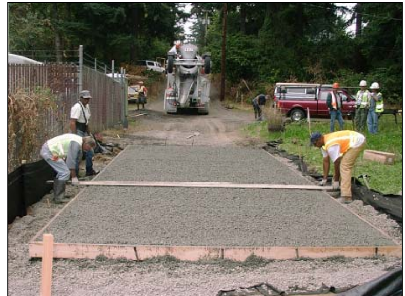
Porous PCCP construction.
