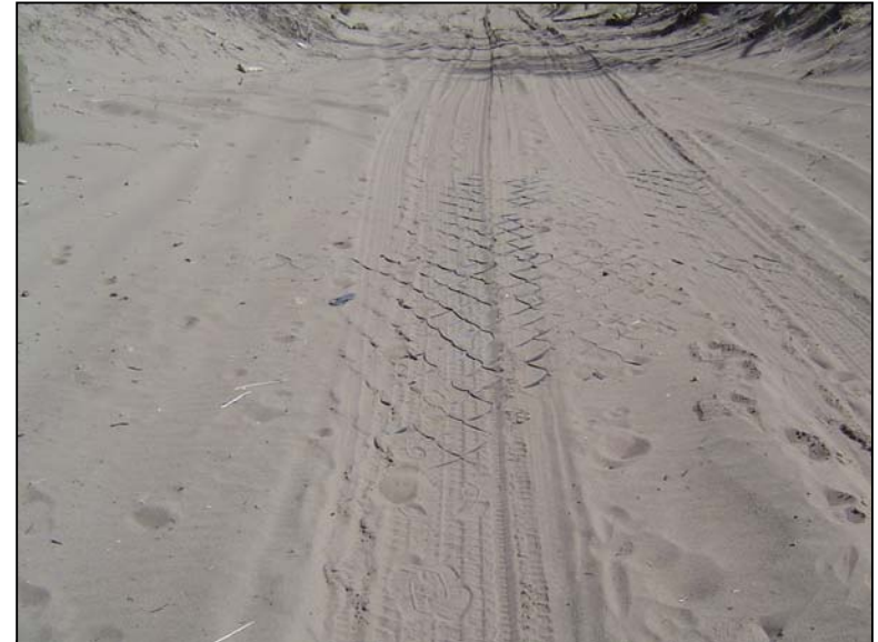
Cellular confined sand surfacing.
