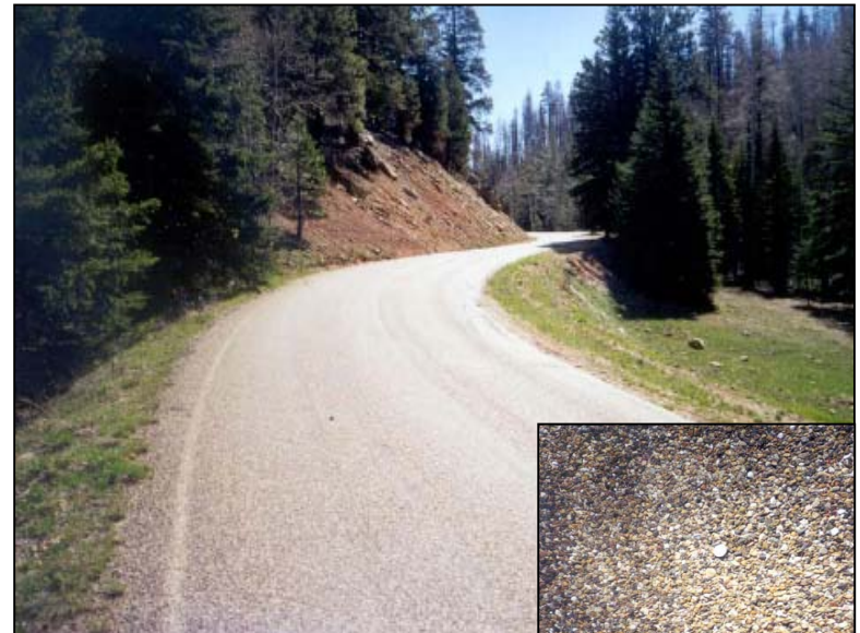
Chip seal surfacing.
