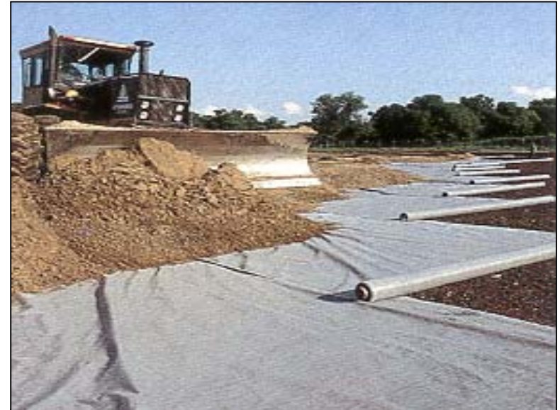
Geotextile for subgrade stabilization.
