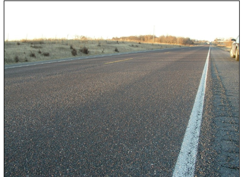
Double chip seal surfacing.
