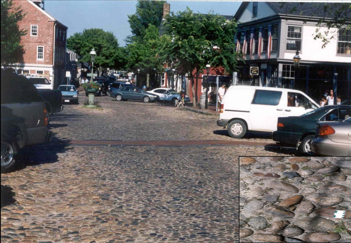
Natural stone paver surfacing.
