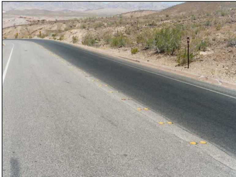
Fog seal on right lane of roadway.
