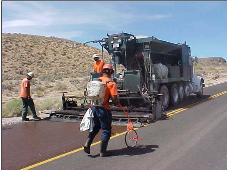
Microsurfacing placement.
