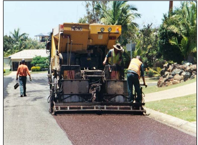
Slurry seal placement.
