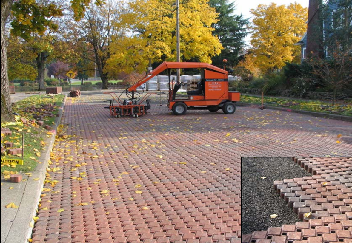
Porous unit paver surfacing.
