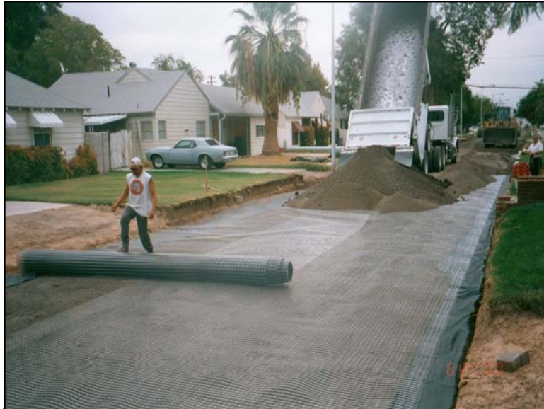
Geogrid placement for base reinforcement.
