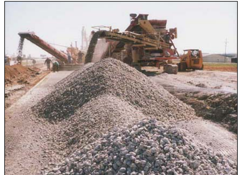
Concrete aggregate reclamation process.
