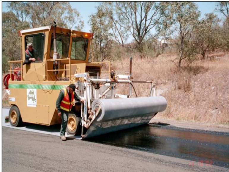
Geotextile placement.
