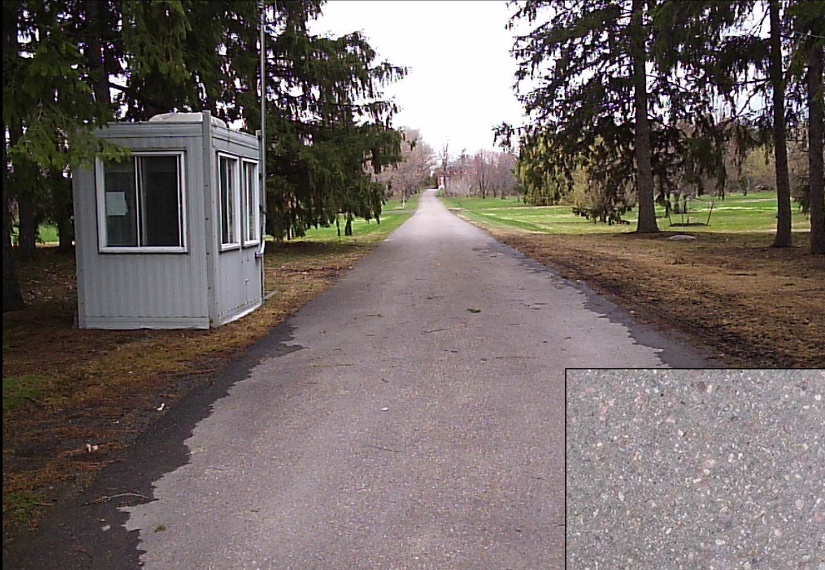
Exposed Aggregate HACP surfacing.
