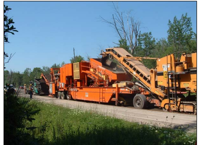
Foamed asphalt equipment train.
