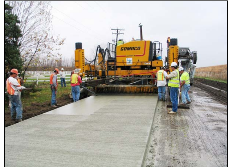
PCCP construction: concrete paving.
