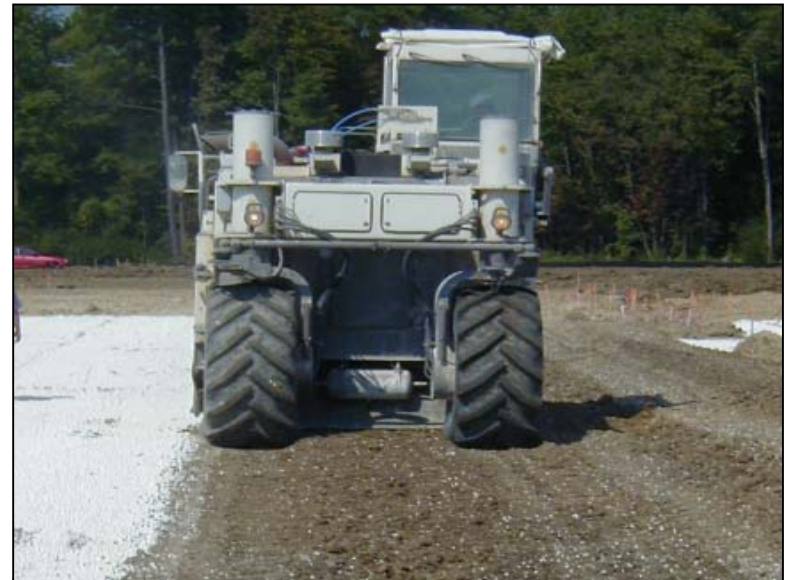
Mixing lime into subgrade material.
