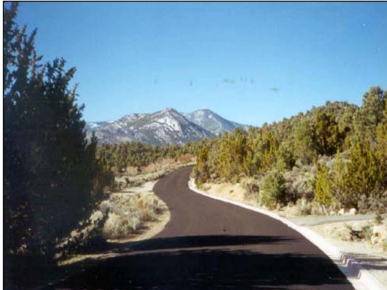
Slurry seal surfacing.
