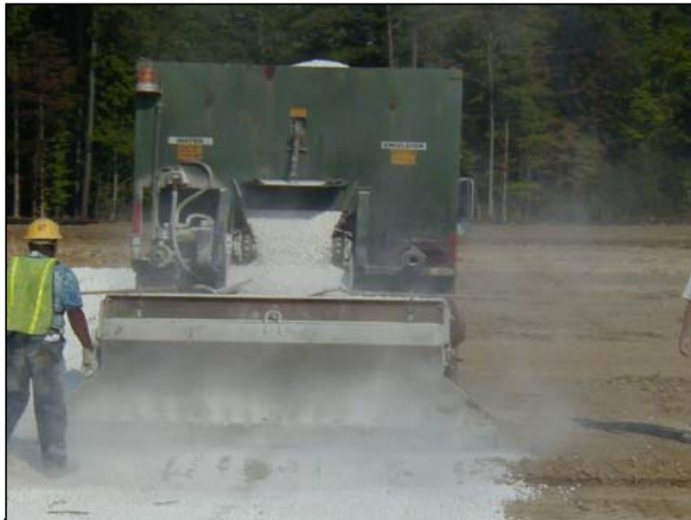
Spreading lime treatment on subgrade.
