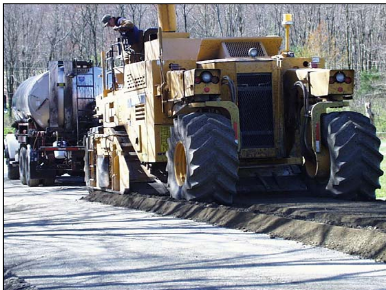
FDR-emulsified asphalt construction.
