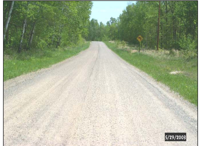
Otta seal surfacing.
