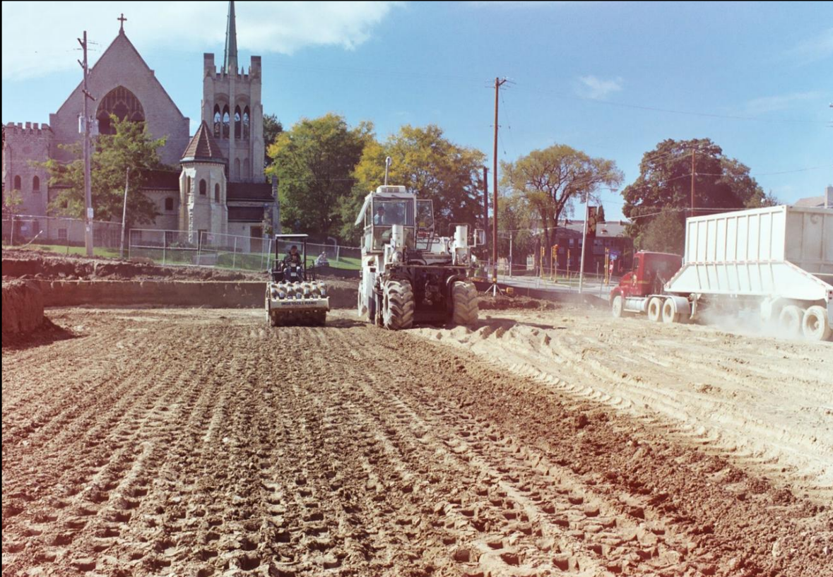
Spreading fly ash for soil treatment.
