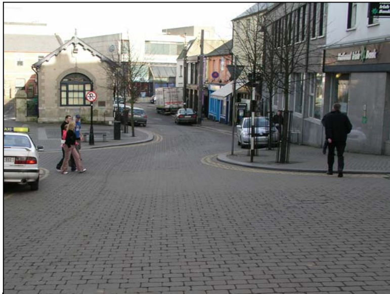
PCC paver surfacing.
