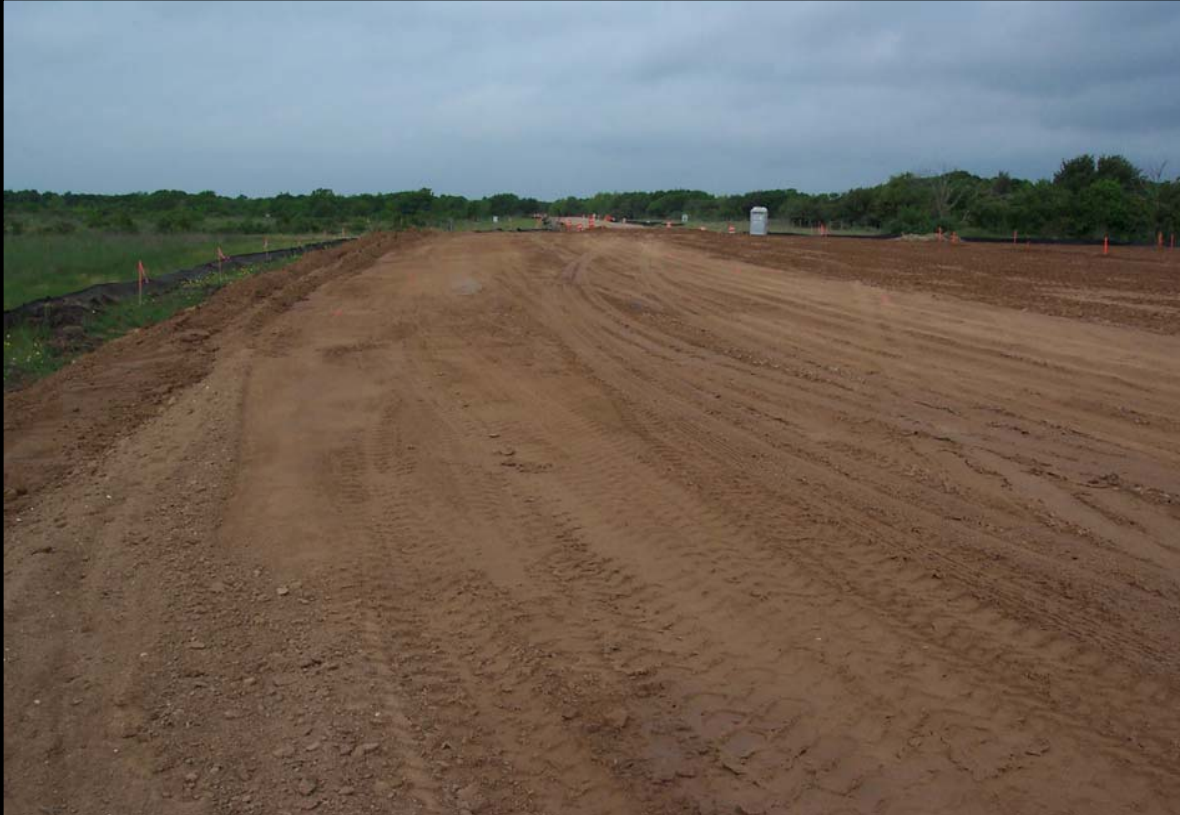
Lime stabilized subgrade material.
