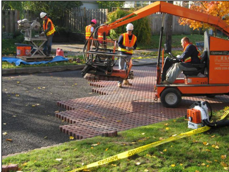
Porous concrete unit paver placement.
