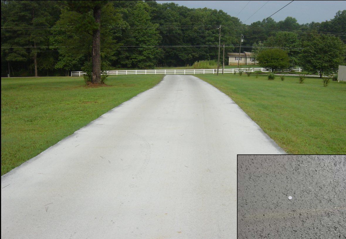
Roller compacted concrete roadway surfacing.
