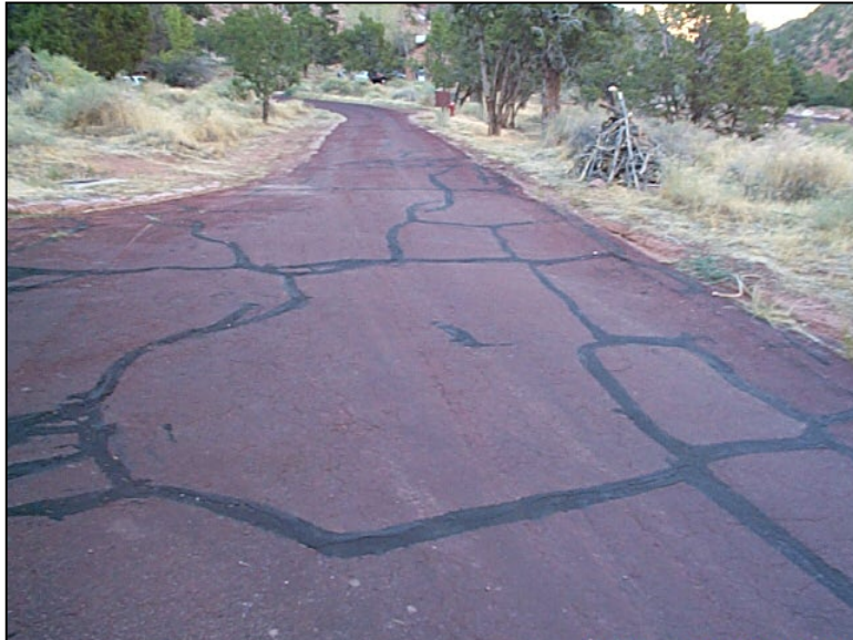
Chip seal crack sealing.
