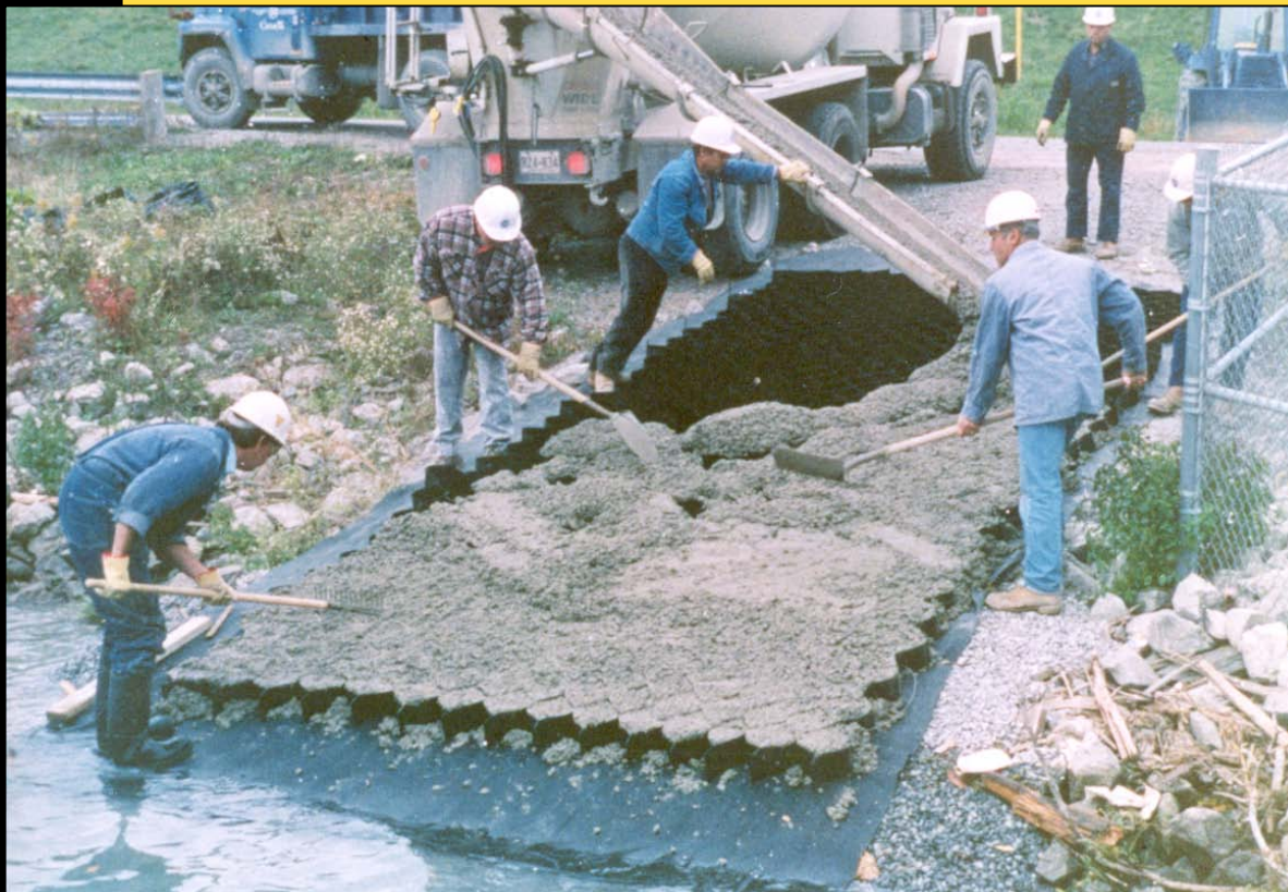
Cellular PCC concrete placement.
