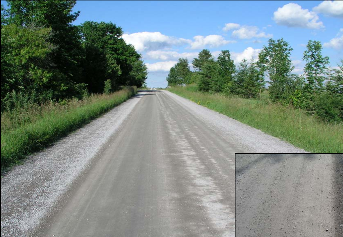
Gravel surfacing treated with CaCl.
