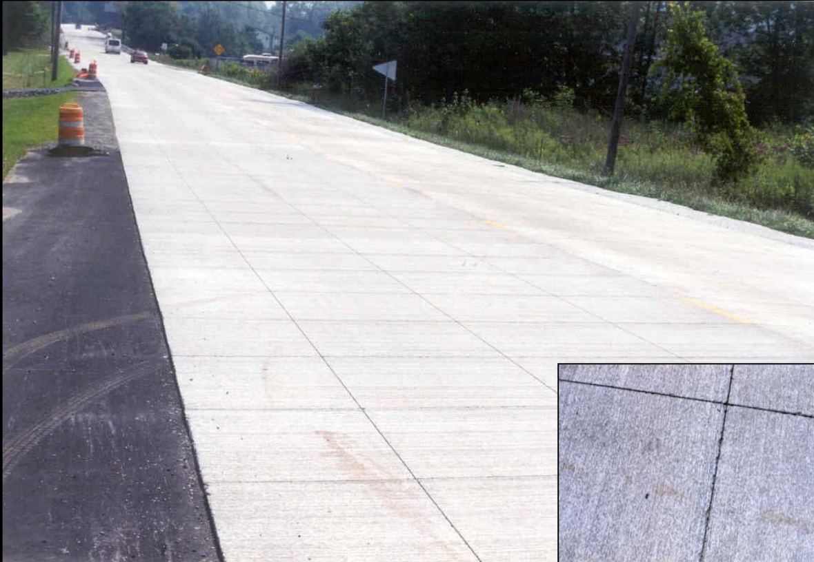
Whitetopping roadway surface.
