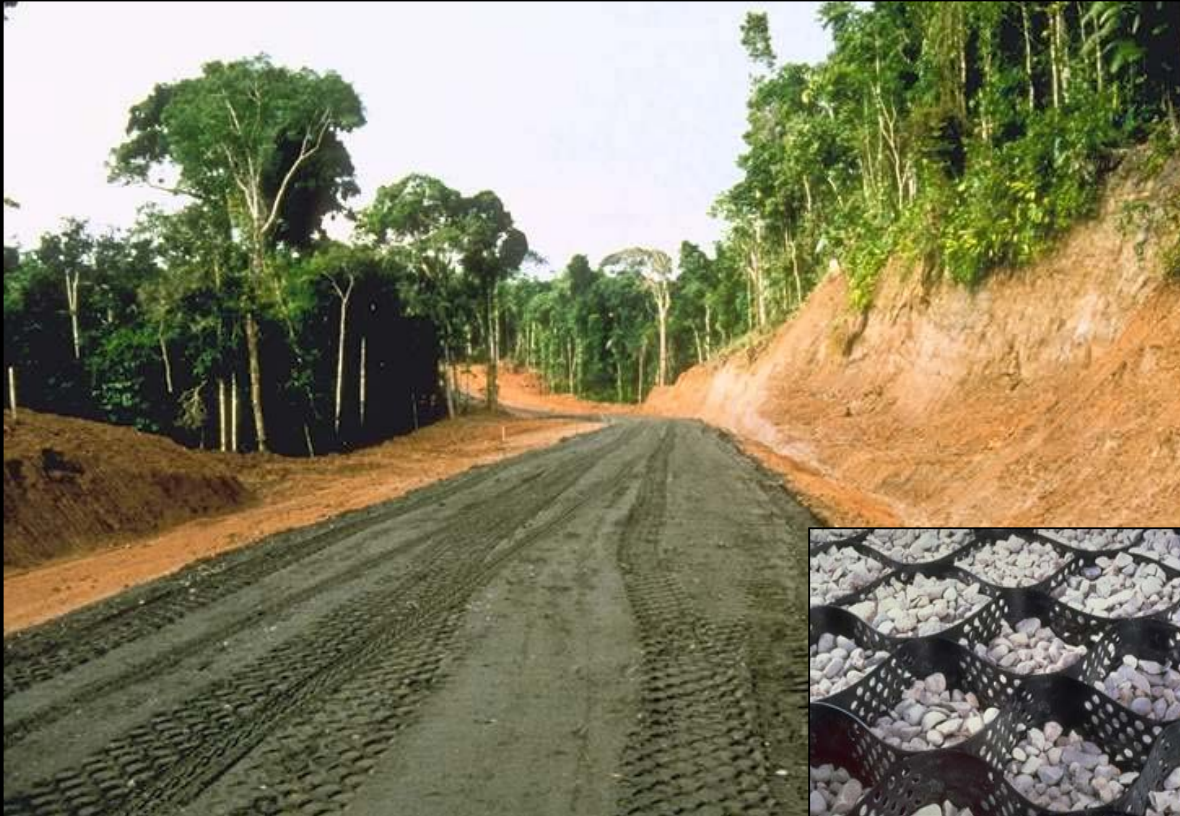
Cellular confined aggregate surfacing.
