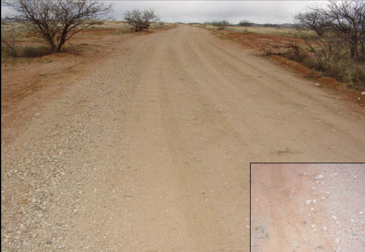
Enzymatic emulsion stabilized surfacing.
