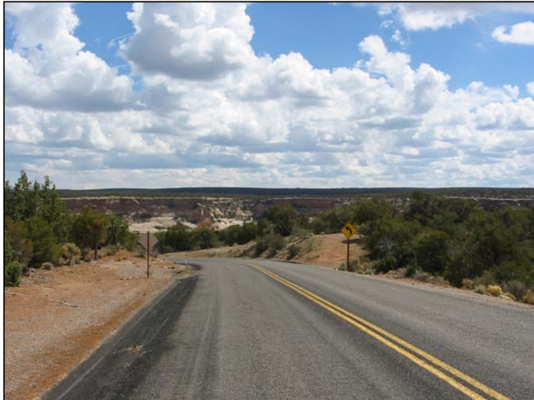
Chip seal surfacing.
