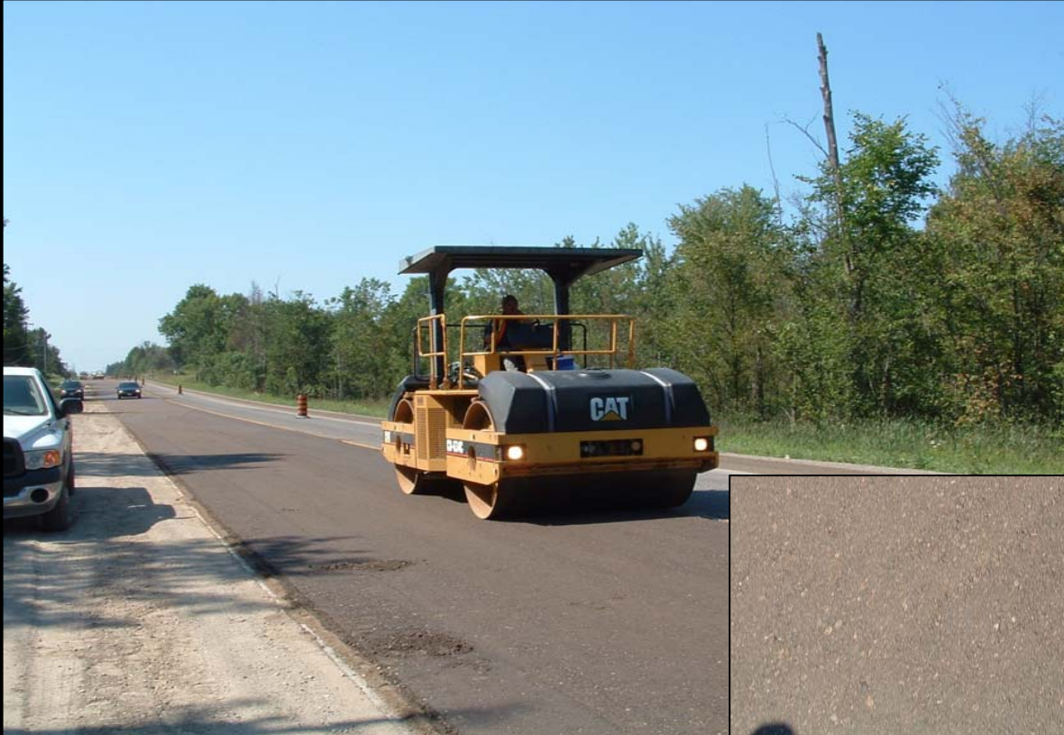
Foamed asphalt base layer.
