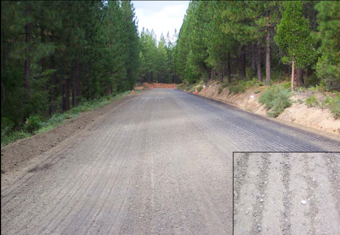
Pulverized roadway material.
