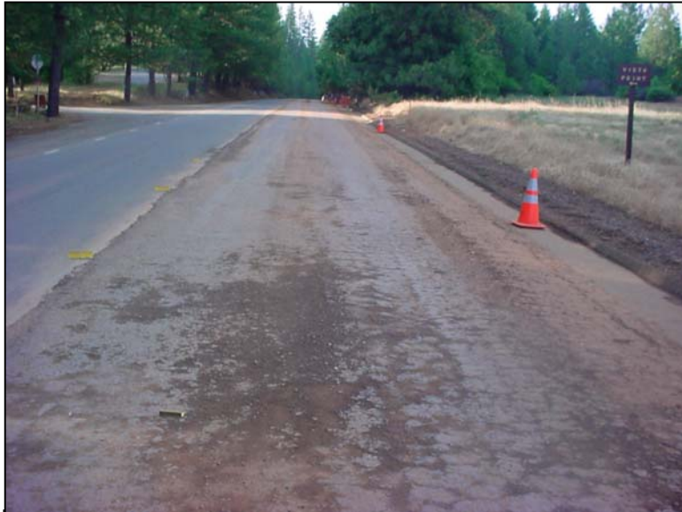
Foamed asphalt material in right lane.
