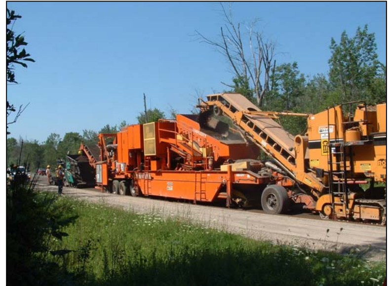
Foamed asphalt equipment train.
