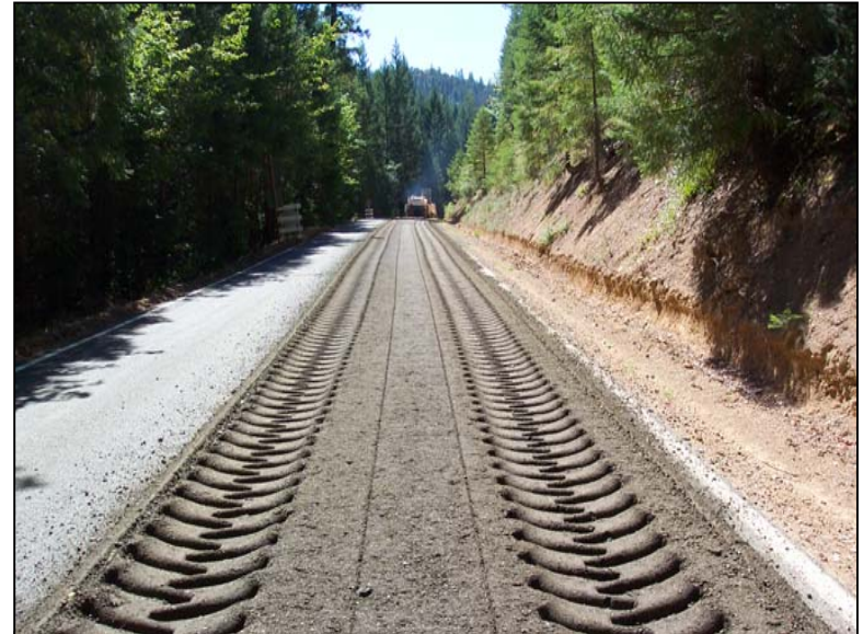
Pulverized material prior to compaction.
