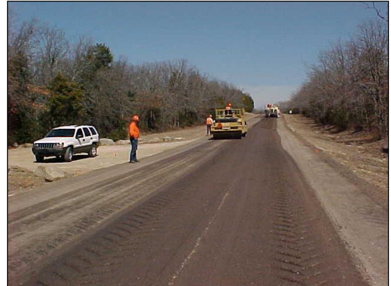
Compaction of FDR-emulsified asphalt material.
