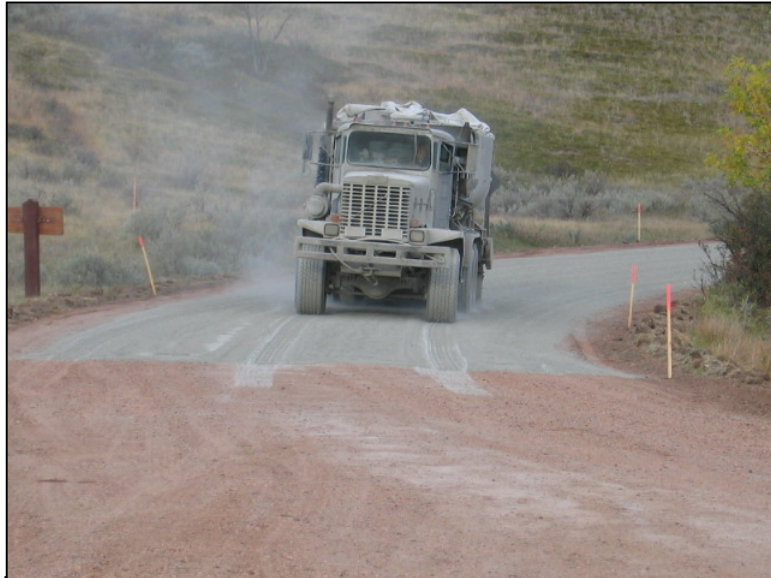
Spreading of cement prior to reclamation process.
