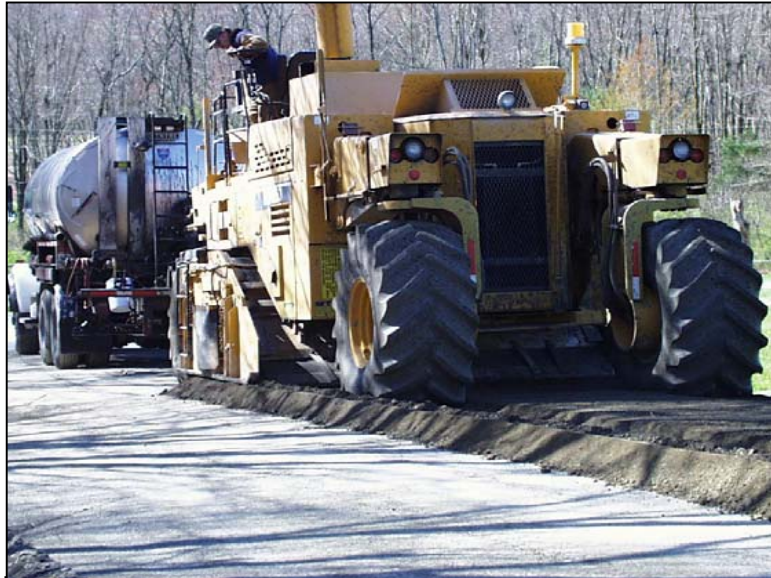
FDR-emulsified asphalt construction.
