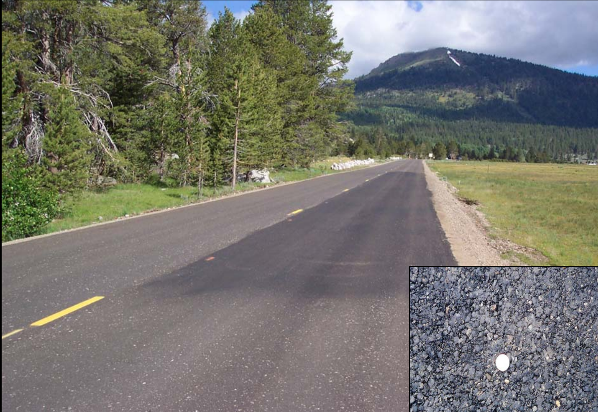
Cold in-place recycled material.
