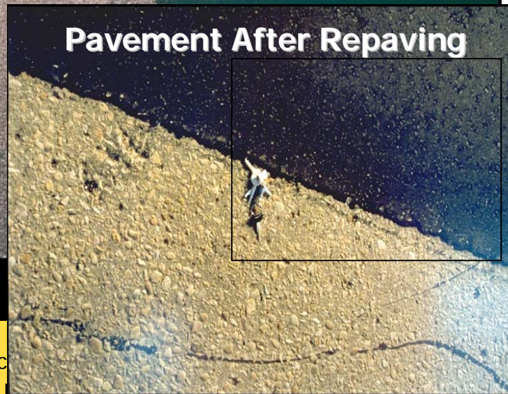
Hot in-place recycled pavement on right.
