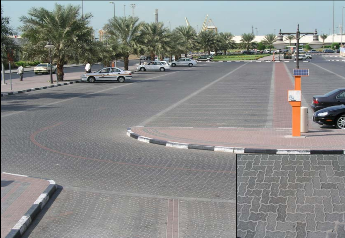
Concrete unit paver surfacing.
