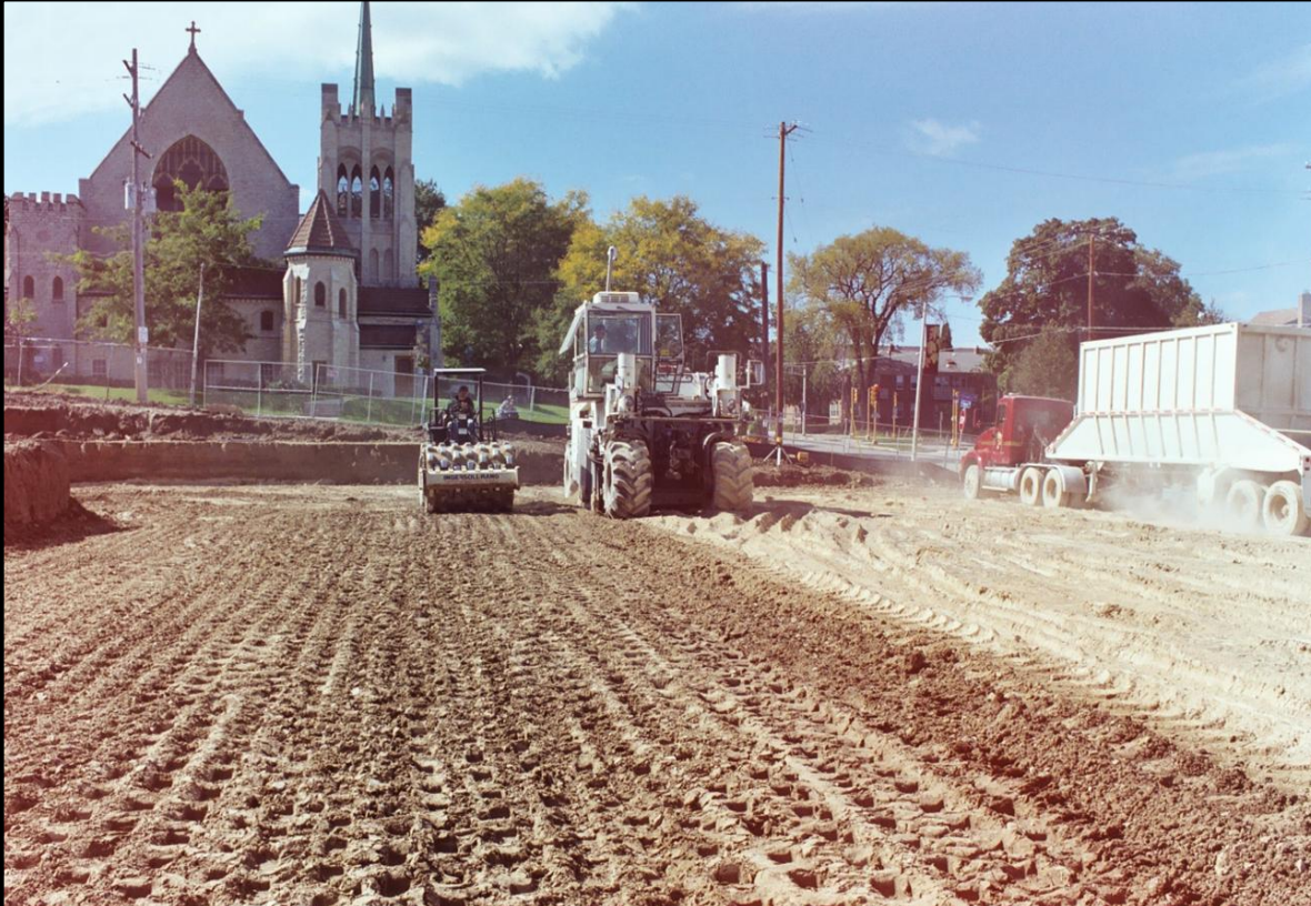
Spreading fly ash for soil treatment.
