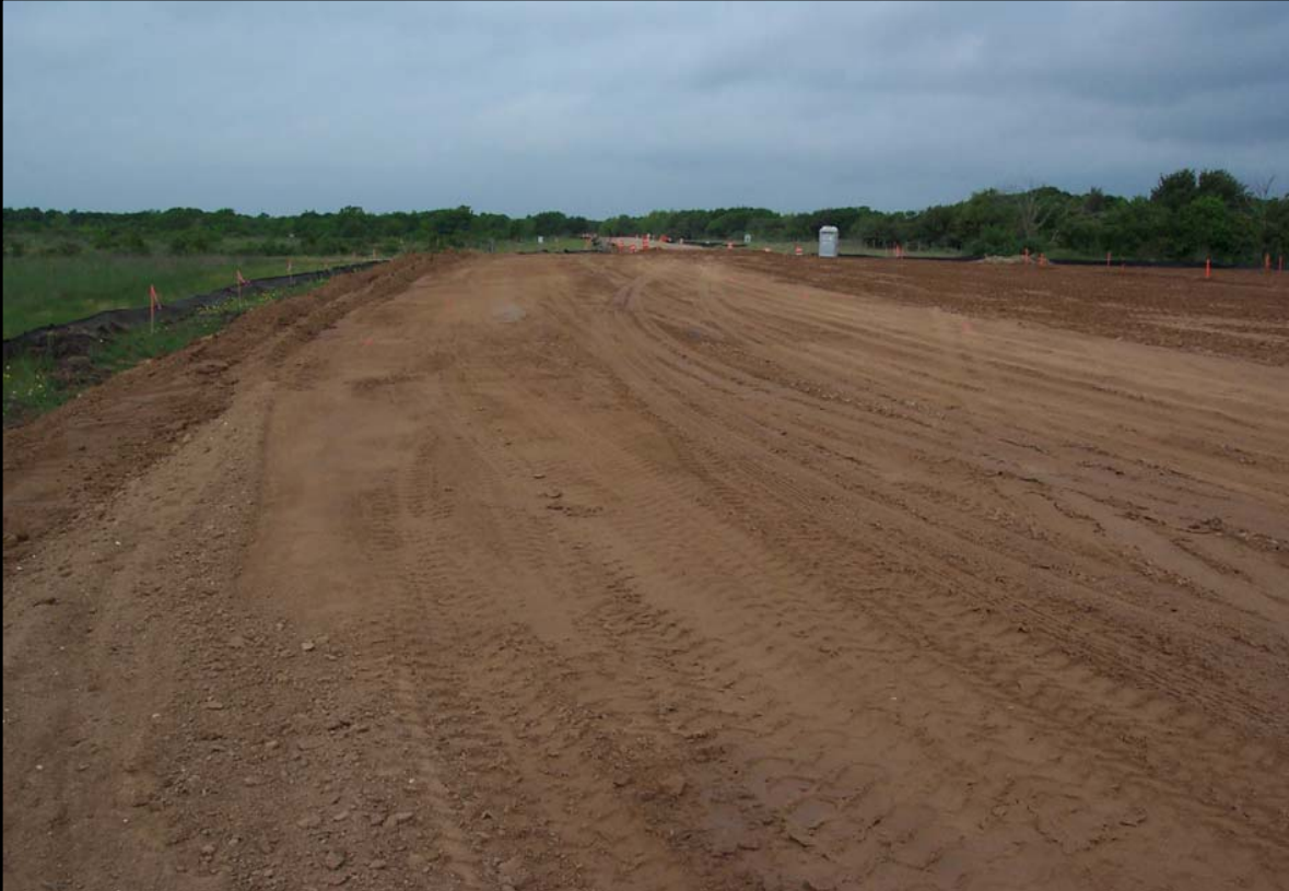
Lime stabilized subgrade material.
