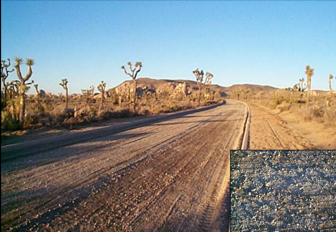
Portland cement stabilized base material.
