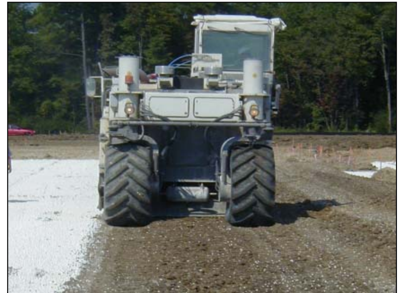
Mixing lime into subgrade material.
