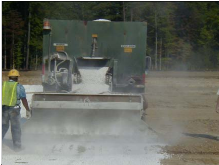
Spreading lime treatment on subgrade.
