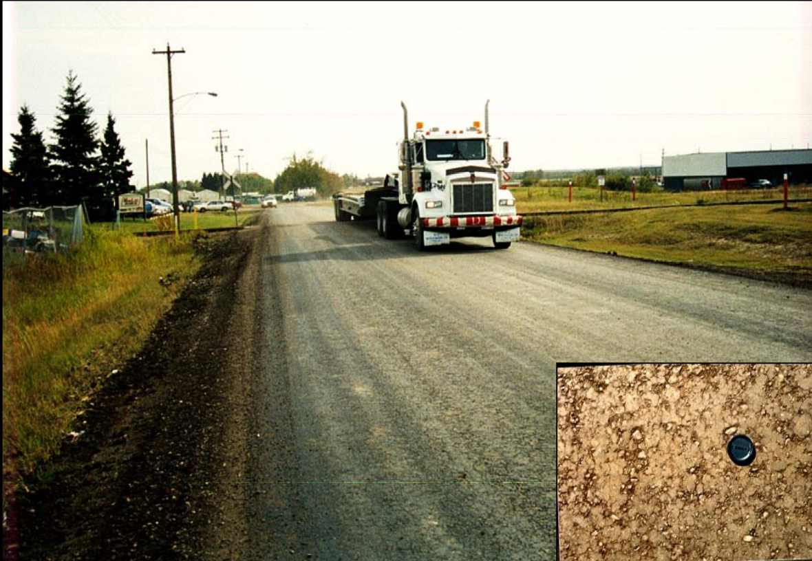
Electrolyte emulsion stabilized surfacing.
