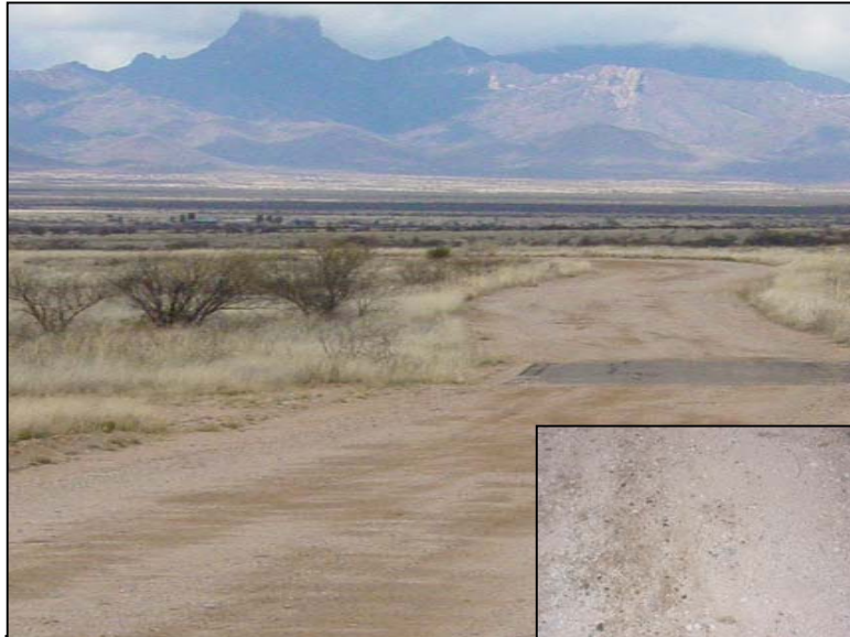
Gravel surfacing treated with MgCl.
