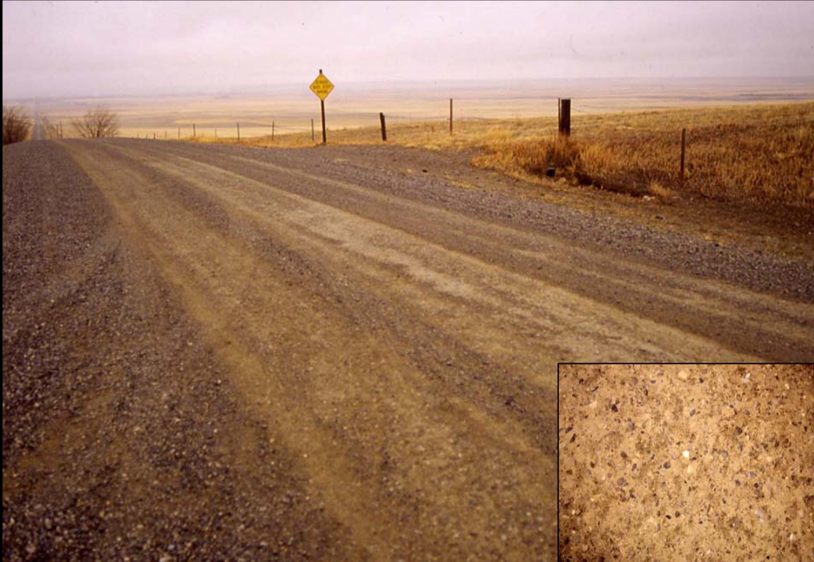
Gravel road stabilized with clay additives.
