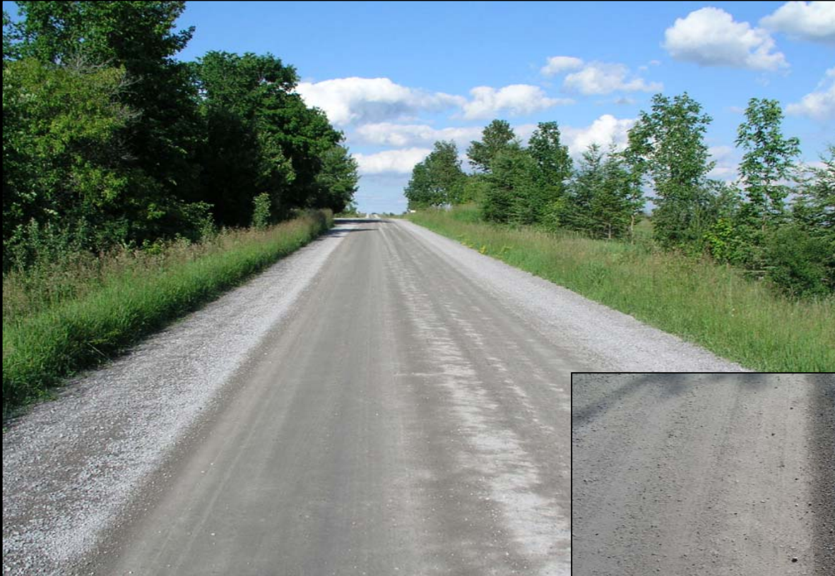
Gravel surfacing treated with CaCl.
