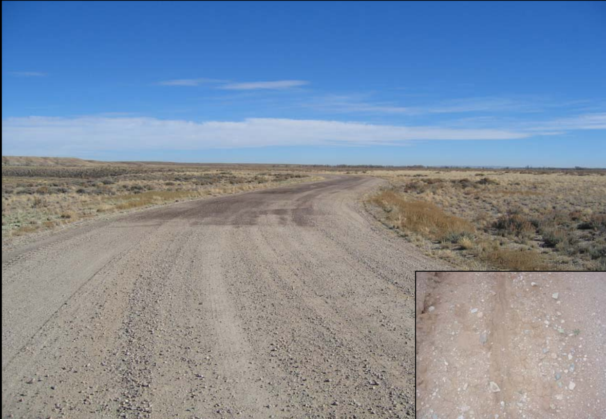
Gravel surfacing treated with lignosulfonates.
