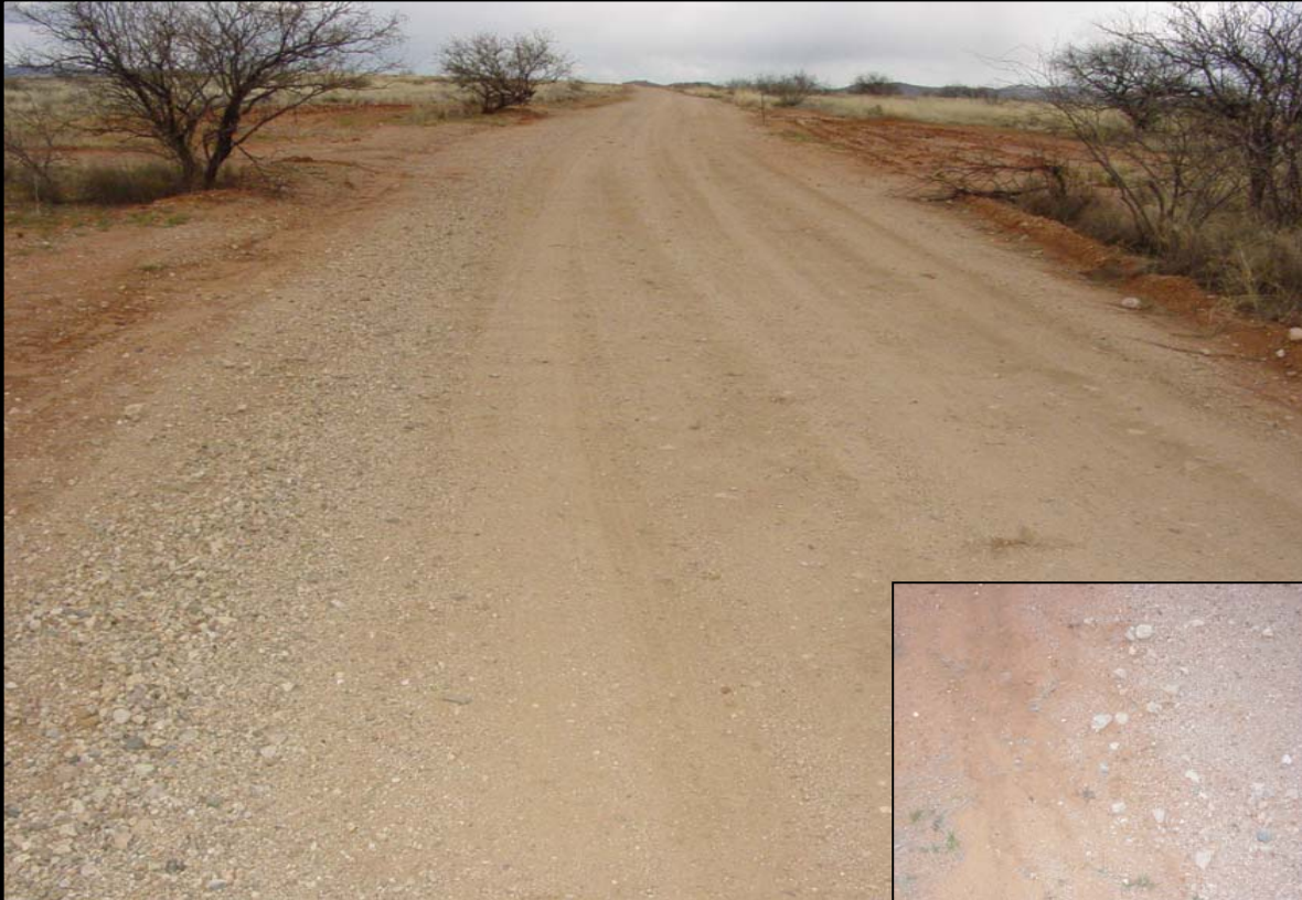
Enzymatic emulsion stabilized surfacing.
