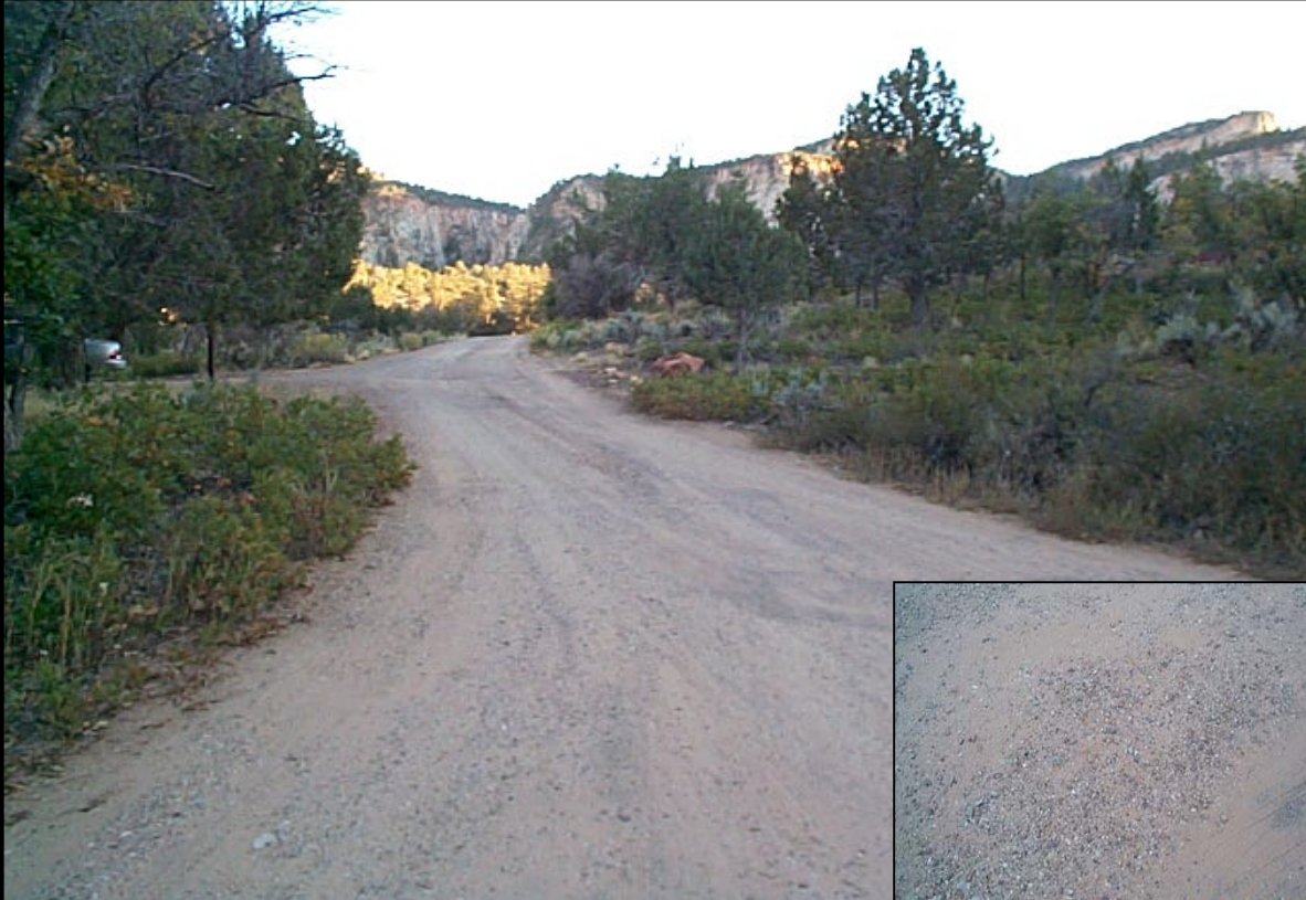
Unbound gravel surfacing.
