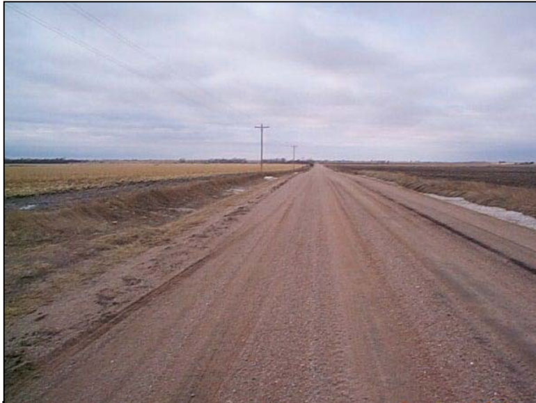
Sand roadway surfacing.
