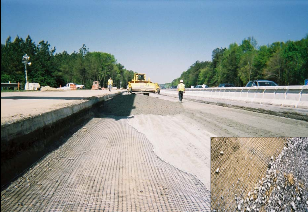
Spreading aggregate base over geogrid layer.
