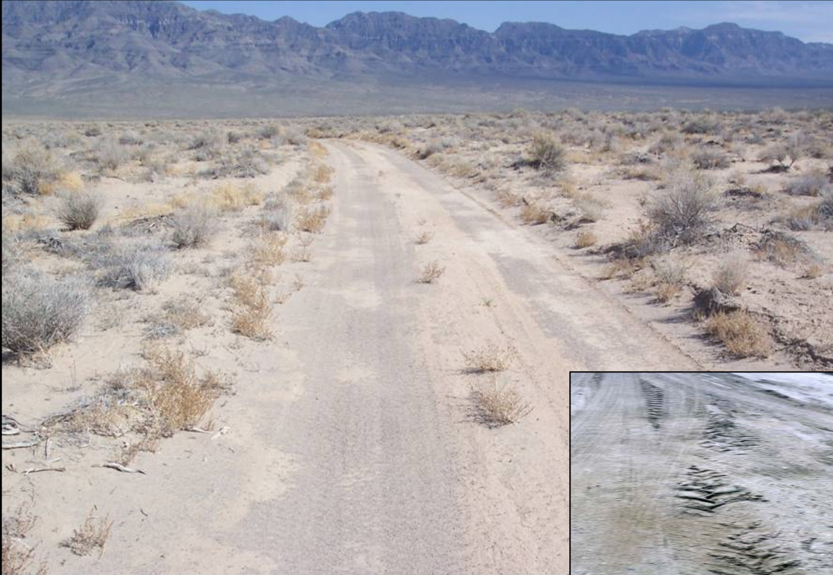
Sand roadway surfacing.
