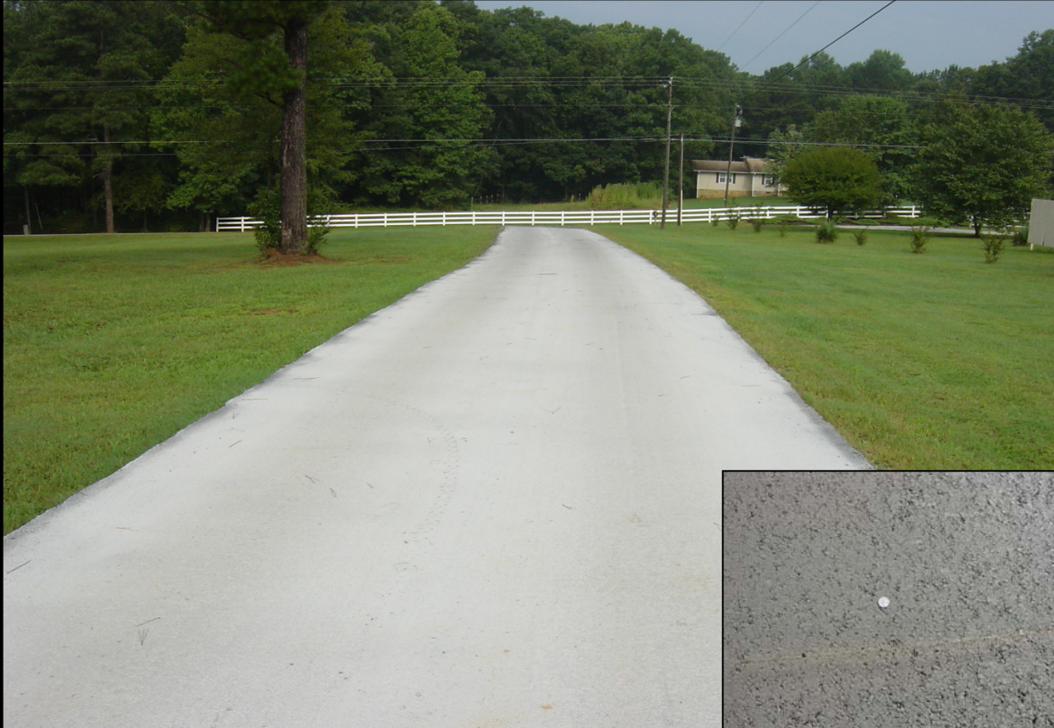
Roller compacted concrete roadway surfacing.
