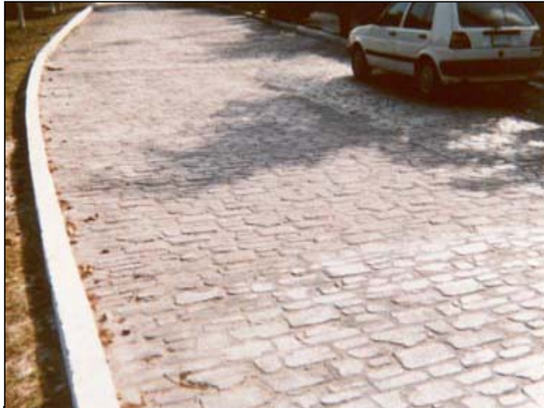
Stamped PCCP surfacing.
