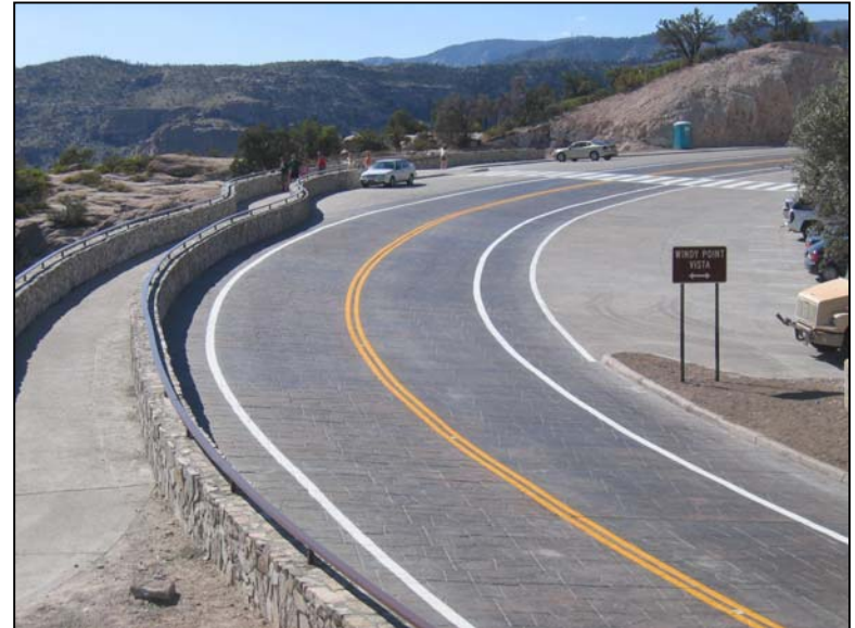
Stamped PCCP surfacing.
