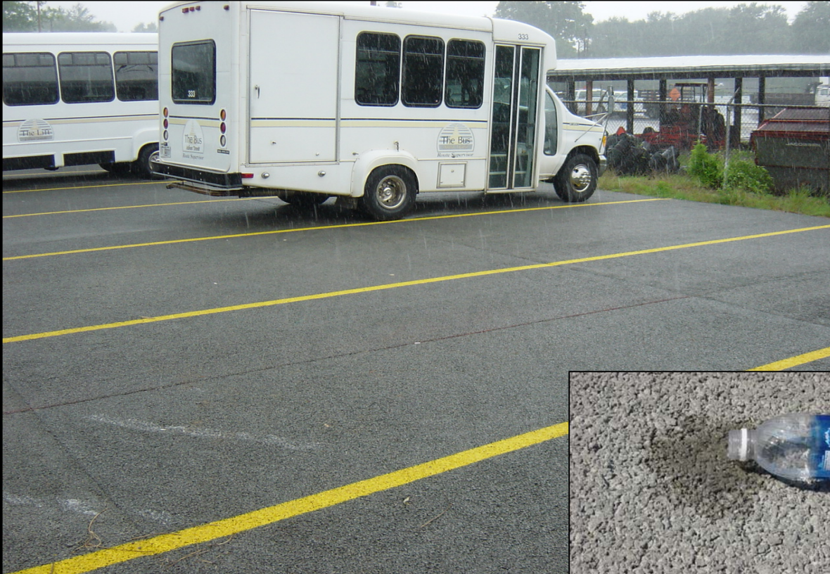
Porous PCCP parking lot.
