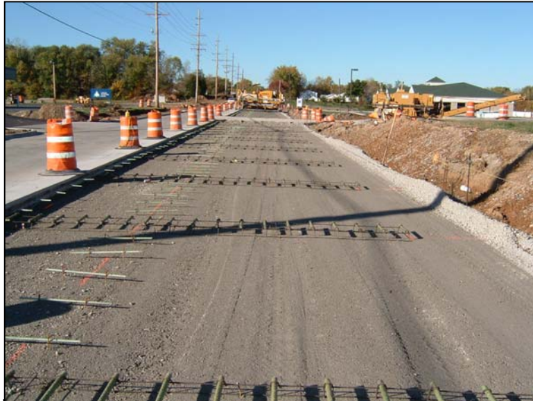
PCCP construction: dowel bar placement.
