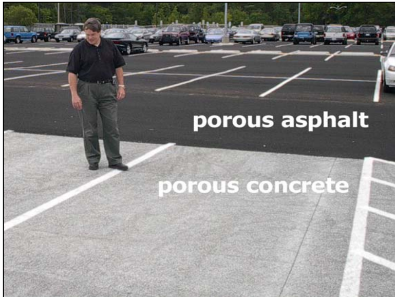
Porous PCCP parking lot.
