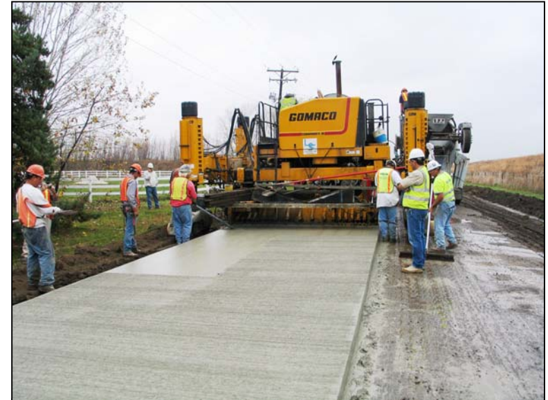
PCCP construction: concrete paving.
