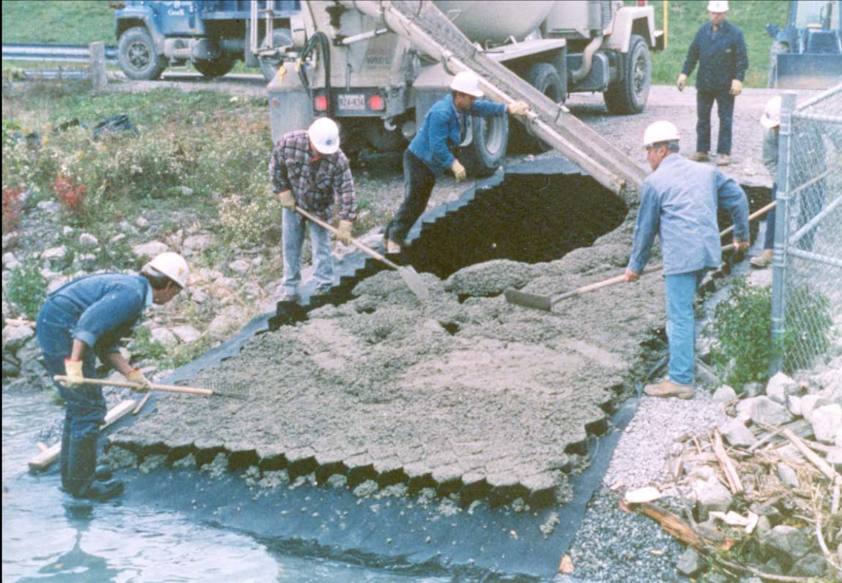
Cellular PCC concrete placement.
