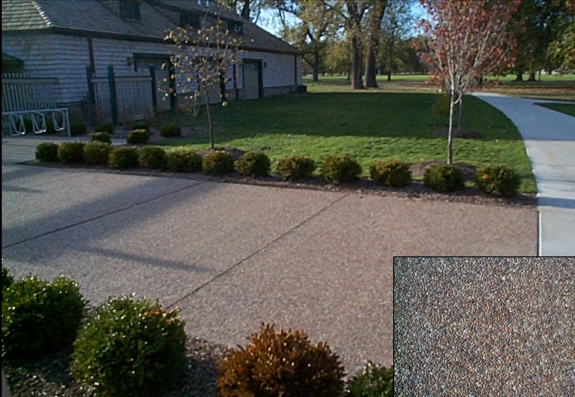
Exposed aggregate PCCP entranceway.
