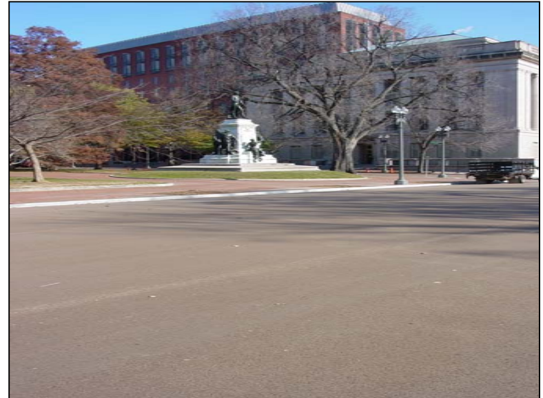
Synthetic binder concrete pavement surfacing
