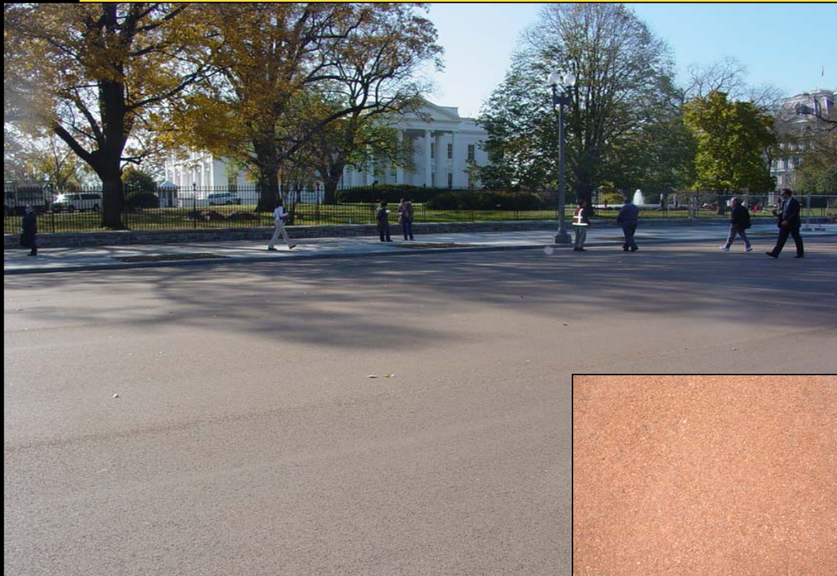
Synthetic binder concrete pavement roadway surfacing.
