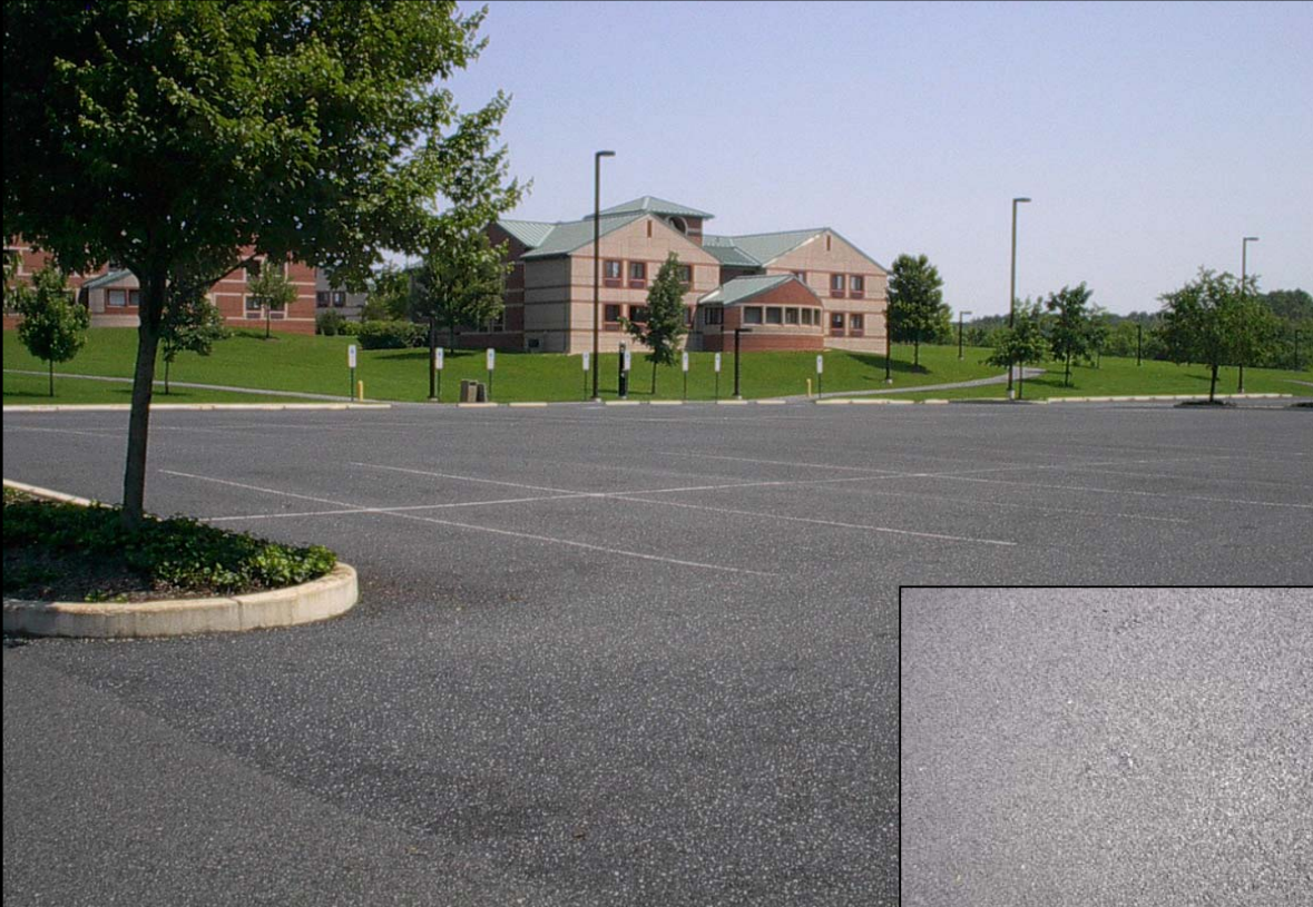
Porous HACP parking lot.
