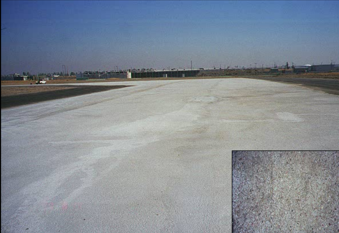
Resin Modified Pavement surfacing.
