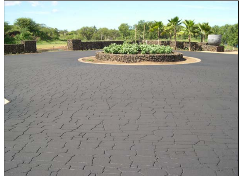
Imprinted HACP surfacing.
