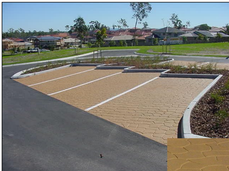
Imprinted HACP parking spaces.
