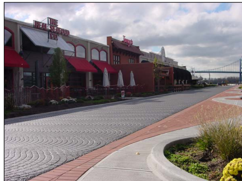
Imprinted HACP surfacing.
