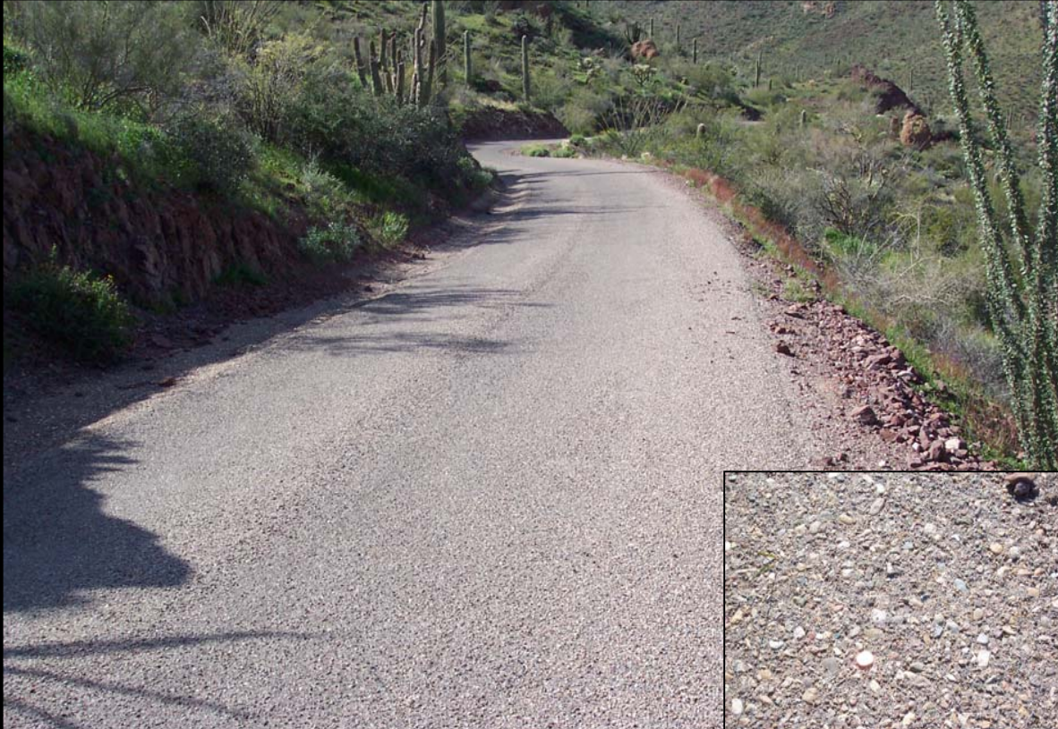
Cold mix asphalt concrete pavement.
