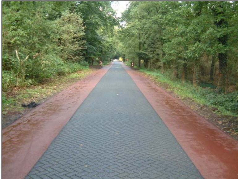
Imprinted HACP surfacing.
