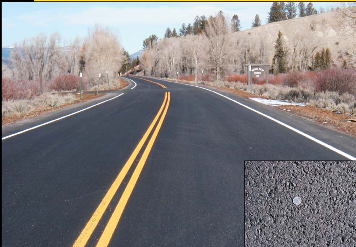
Hot Asphalt Concrete Pavement.
