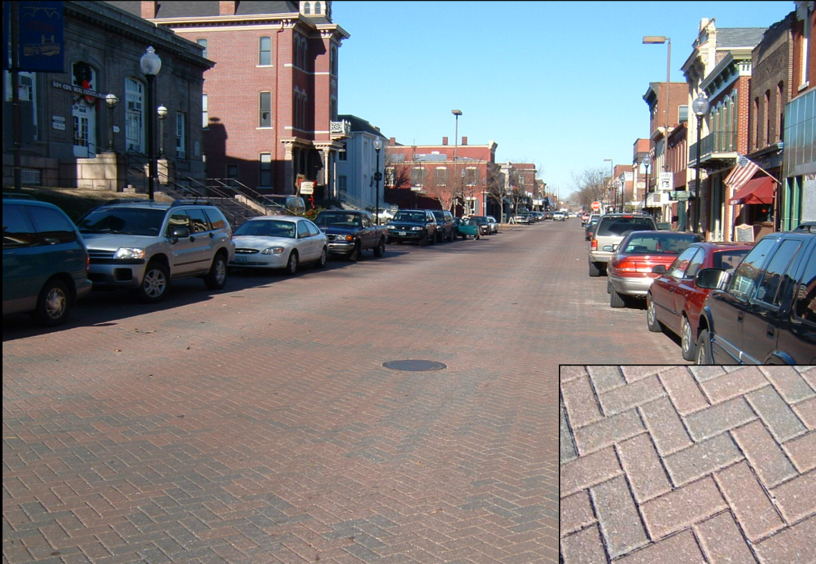
Imprinted HACP street surfacing.
