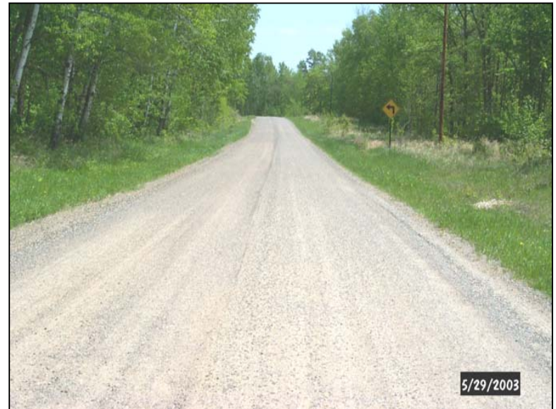
Otta seal surfacing.
