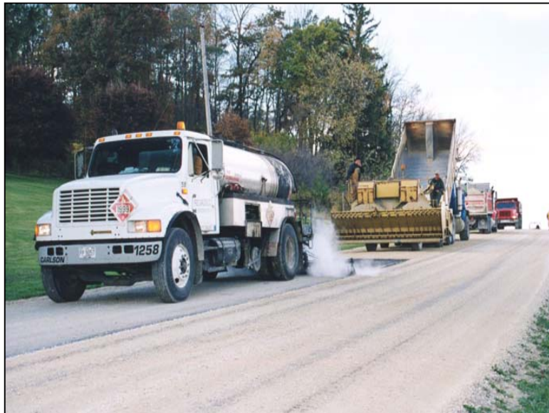
Otta seal construction.
