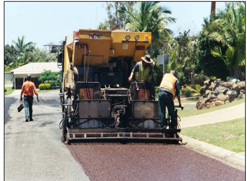
Slurry seal placement.
