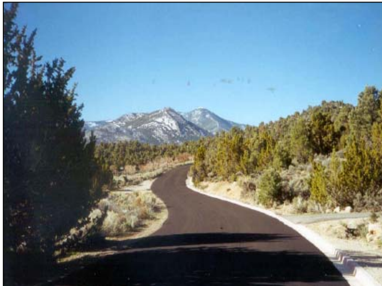
Slurry seal surfacing.
