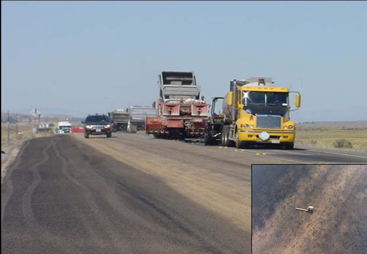
Sand seal construction.
