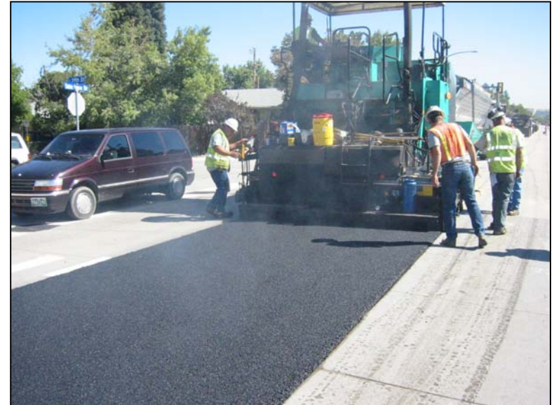
Ultrathin friction course construction.
