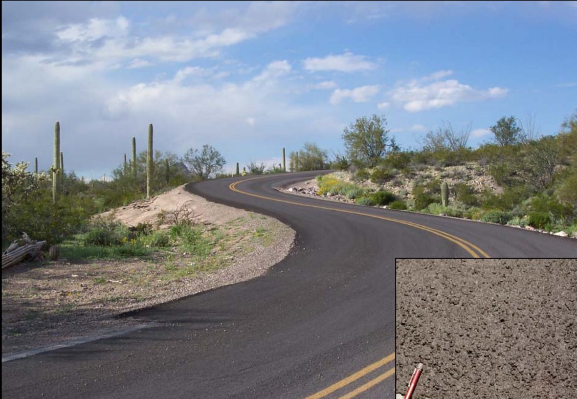
Slurry seal surfacing.
