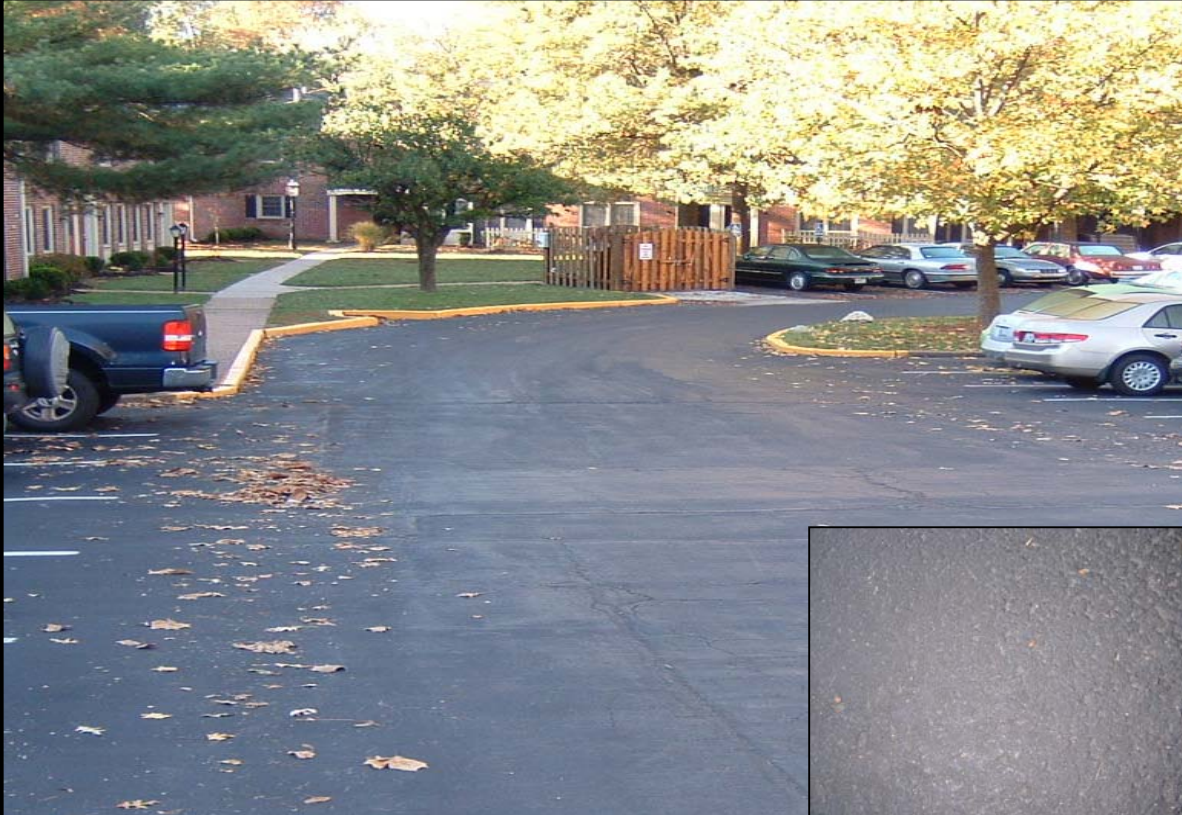
Fog seal surfacing.
