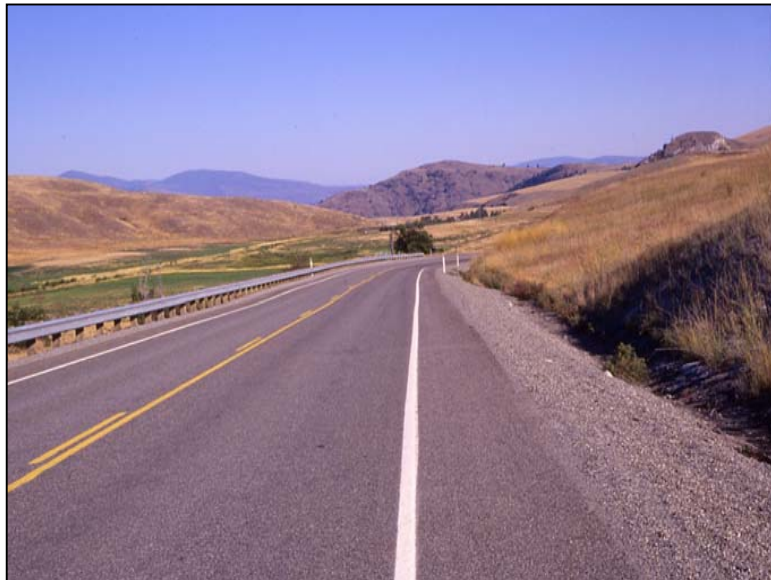
Triple chip seal surfacing.
