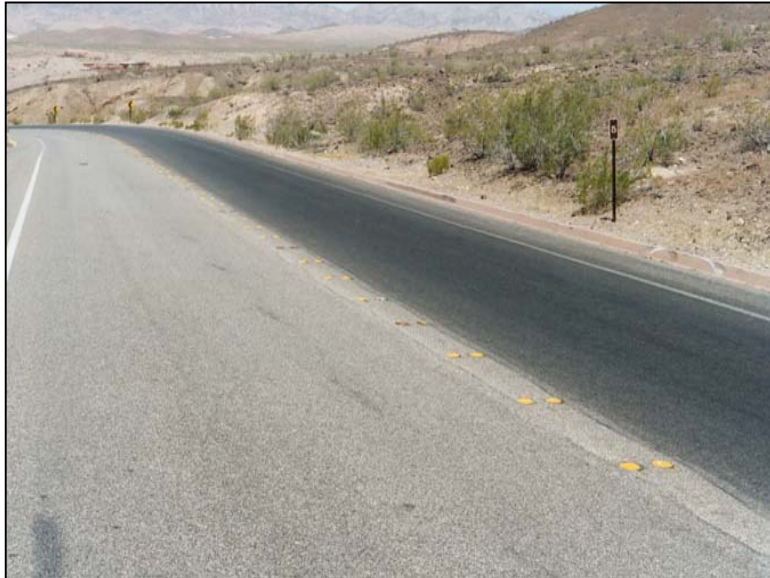
Fog seal on right lane of roadway.
