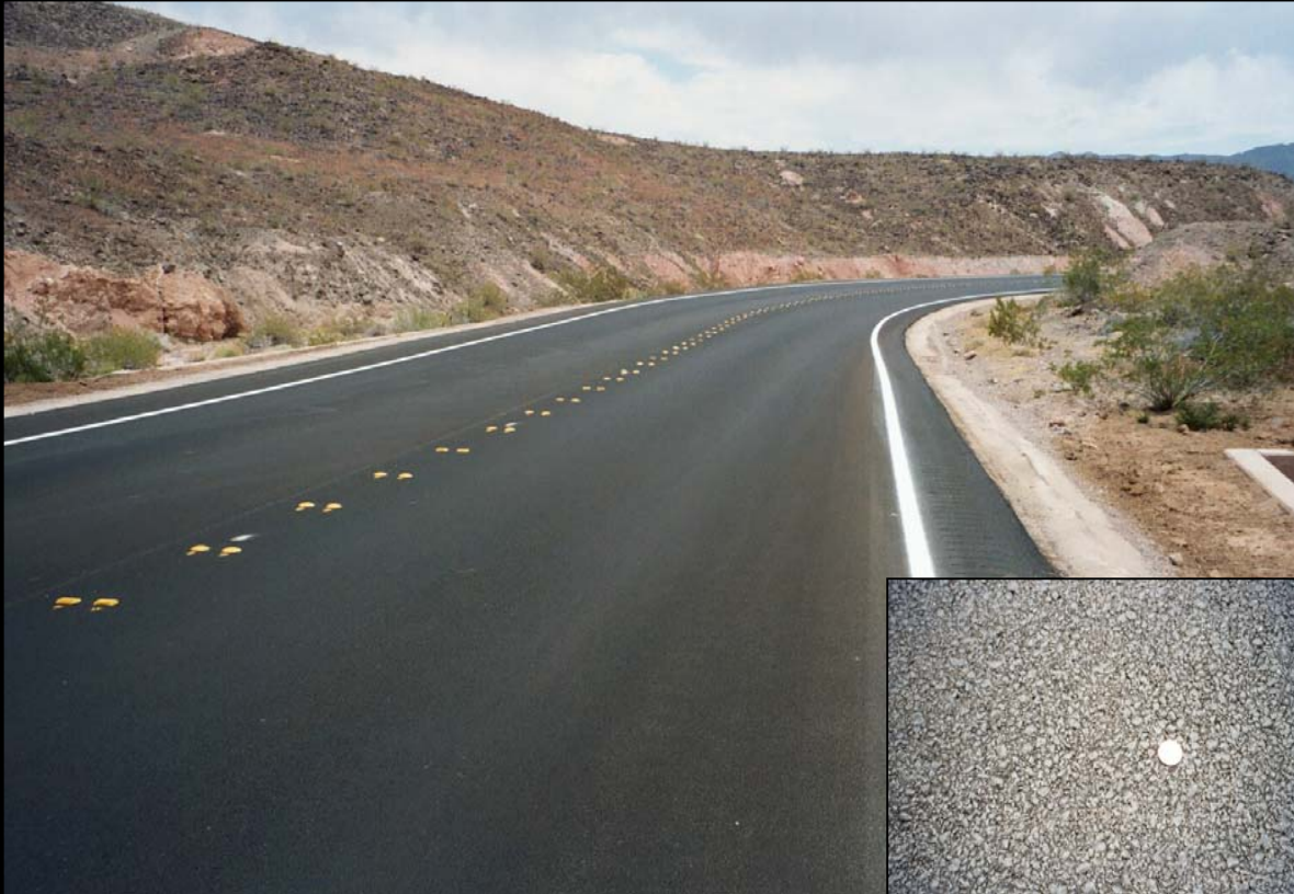
Open graded friction course surfacing.
