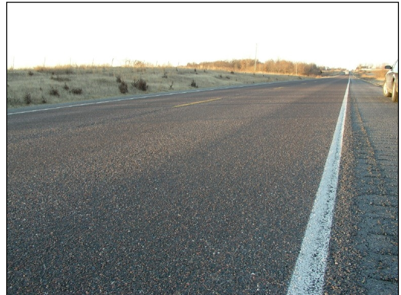
Double chip seal surfacing.
