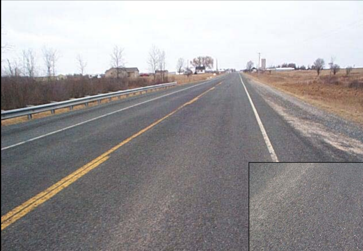
Double chip seal surfacing.
