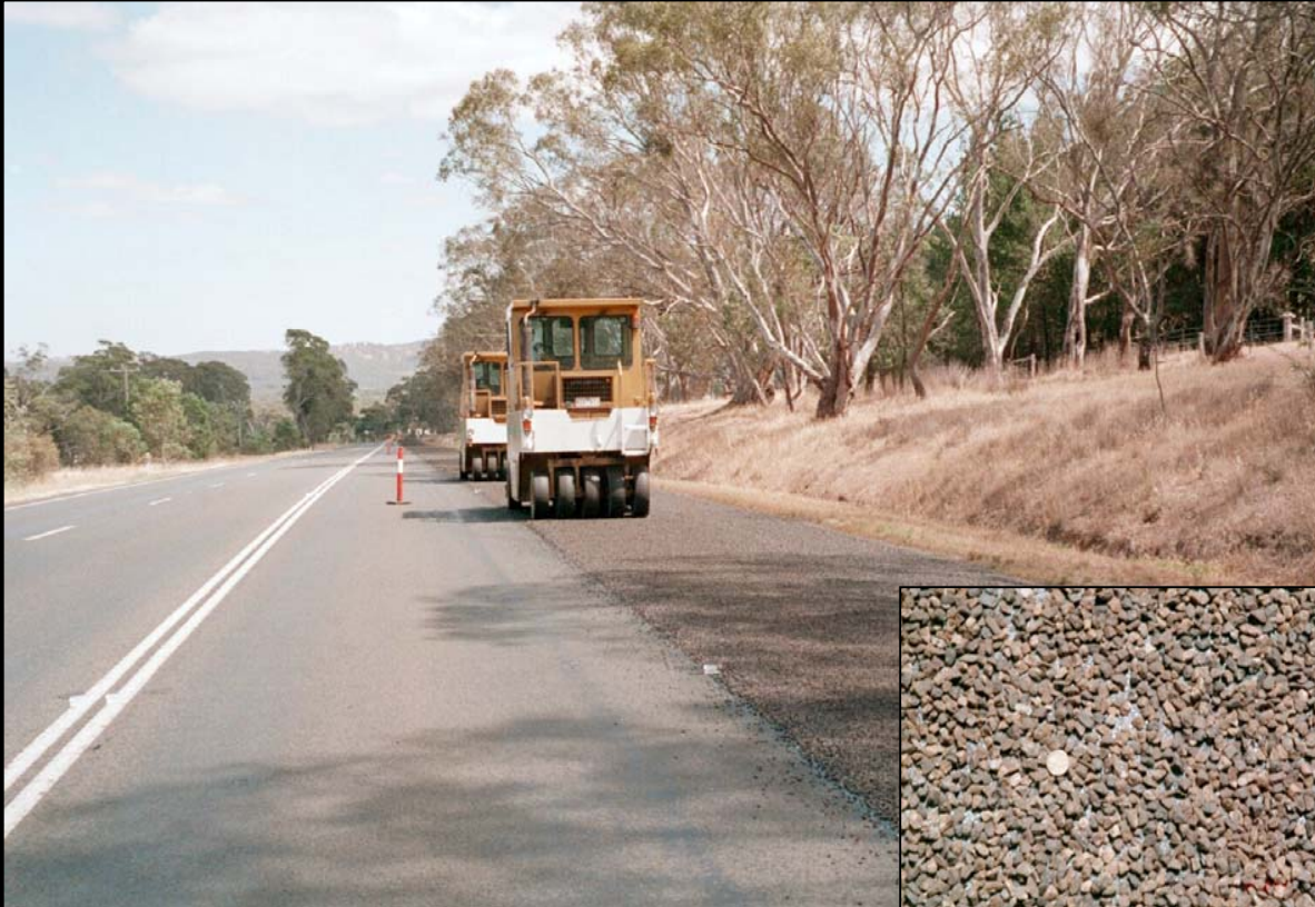
Chip seal over geotextile construction.
