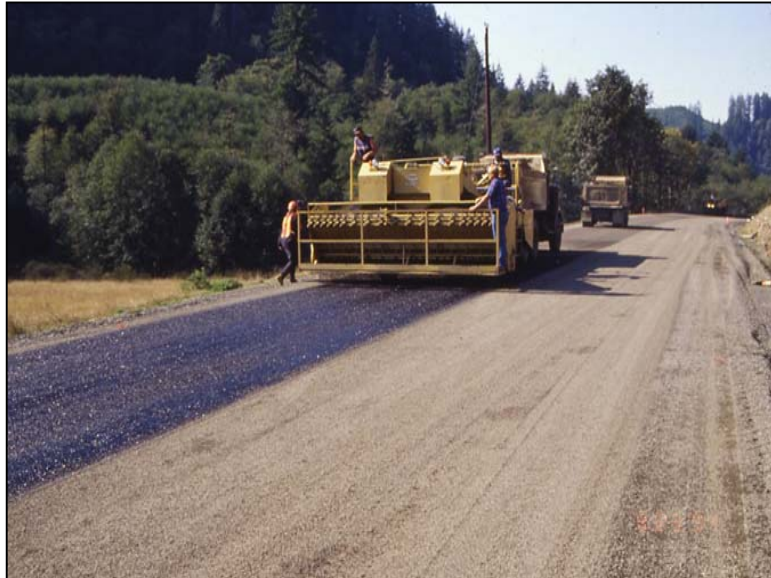
Chip seal construction.
