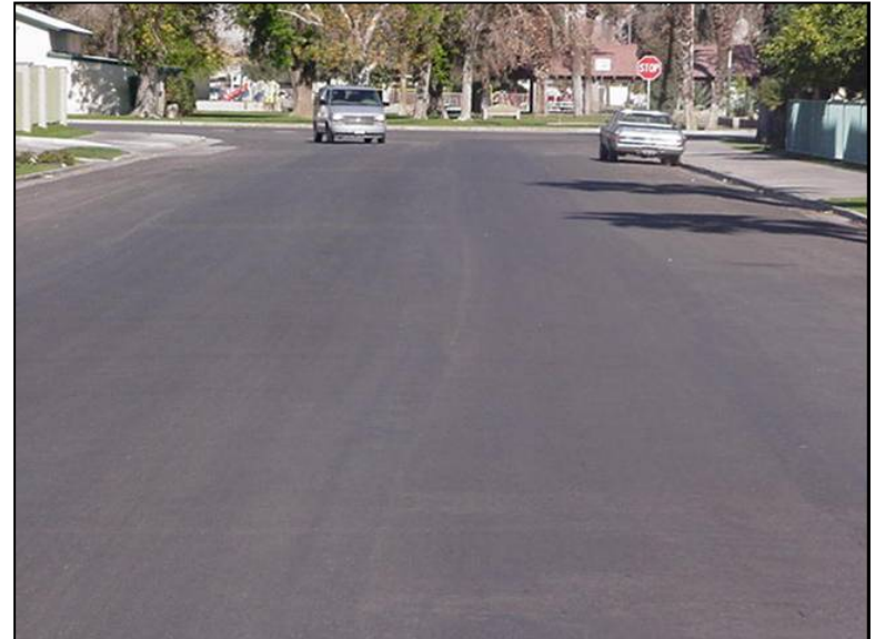
Cape seal surfacing.
