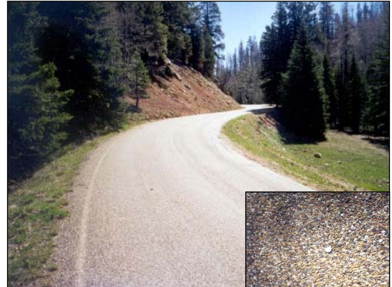
Chip seal surfacing.
