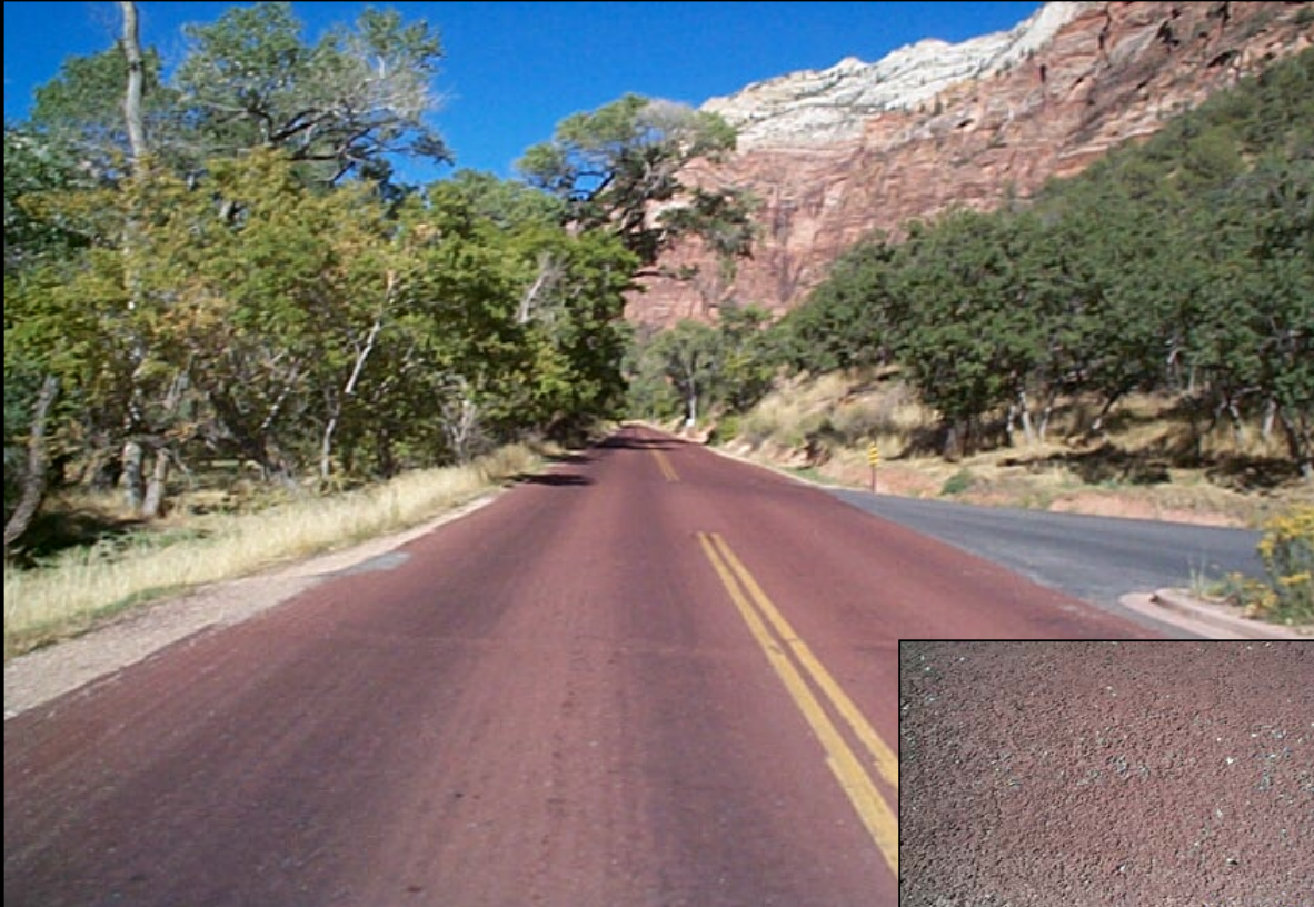
Chip seal surfacing with red aggregate chips.
