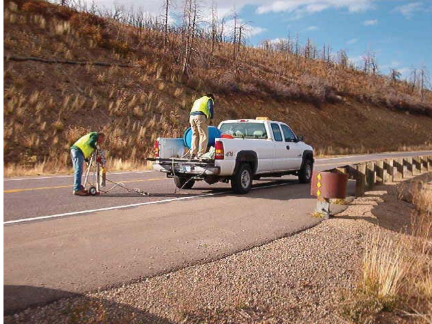
Figure 45. Photo. Coring at Site 4.
