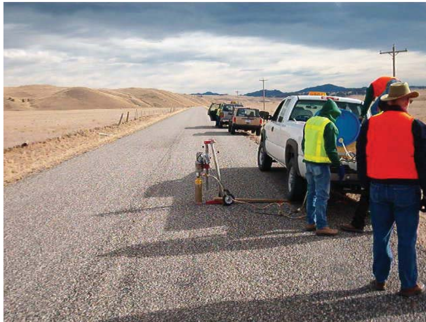
Figure 34. Photo. Coring at Site 1.
