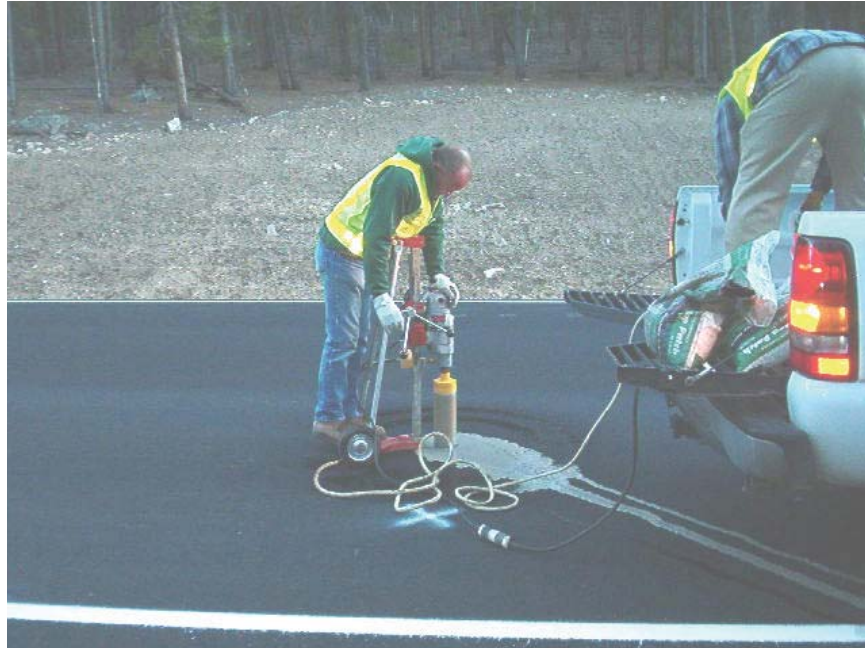
Figure 41. Photo. Coring at Site 3.
