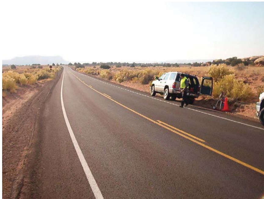
Figure 48. Photo. View of Site 5.
