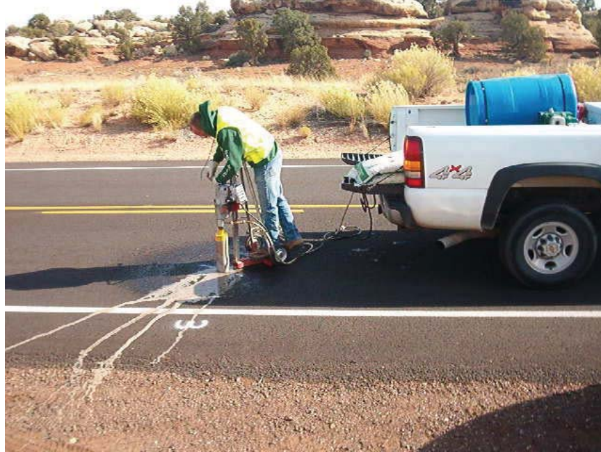
Figure 49. Photo. Coring at Site 5.
