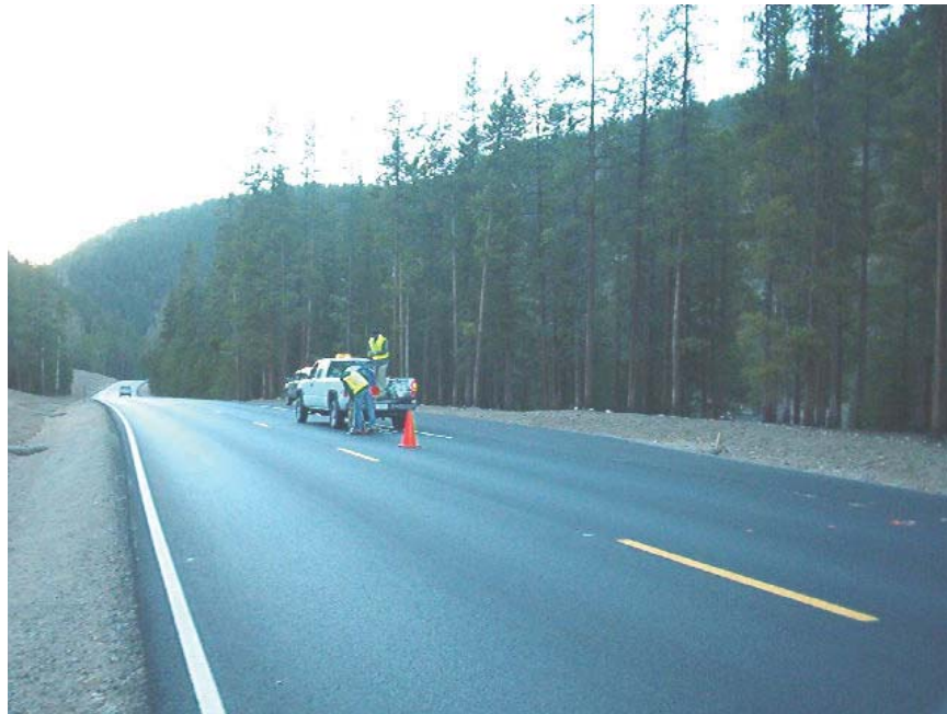
Figure 40. Photo. View of Site 3.
