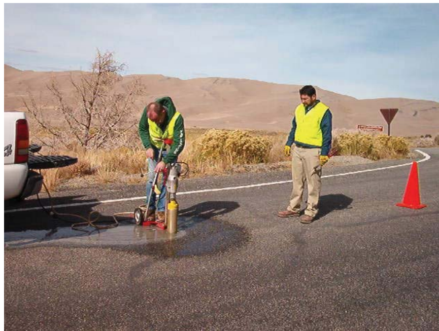
Figure 36. Photo. Coring at Site 2.
