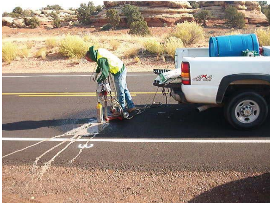
Figure 49. Photo. Coring at Site 5.
