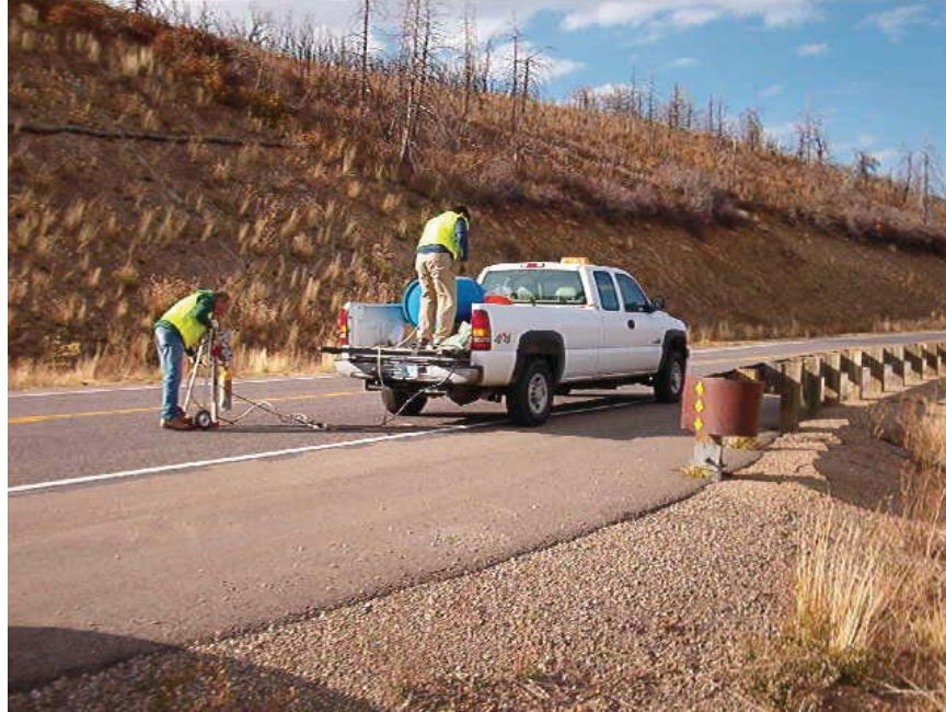
Figure 45. Photo. Coring at Site 4.
