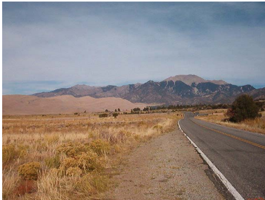
Figure 38. Photo. View of Site 2.
