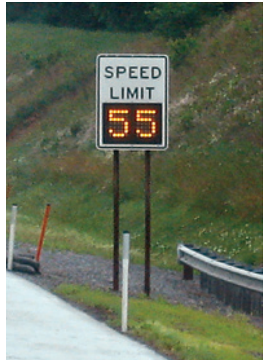
Figure 1: VSL Sign Installation in Pennsylvania (Source: Bryan Katz)
