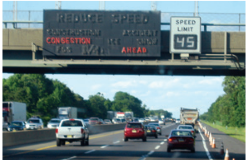
Figure 6: Variable Speed Limit System on the New Jersey Turnpike (Source: Bryan Katz)
