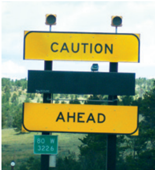
Figure 7: Changeable Message Sign in Wyoming Used to Communicate Speed Reduction Warning (Source: Bryan Katz)
