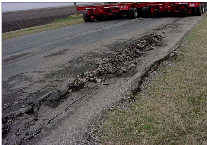
Figure 1. Pavement Damage Caused by Heavy Vehicles
