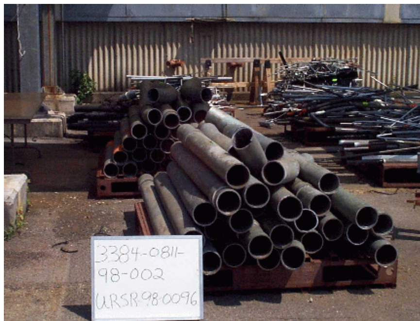
Figure 4.6: Large-bore piping that has been sectioned to permit release surveys
