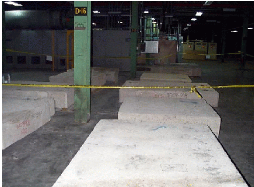
Figure 4.1: Concrete slabs staged for clearance surveys
