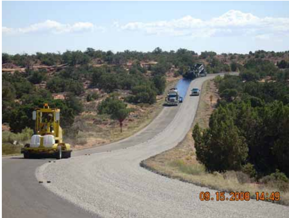
Figure 38. Photo. Utah Parks Project—Canyonlands NP Chip Seal Construction.
