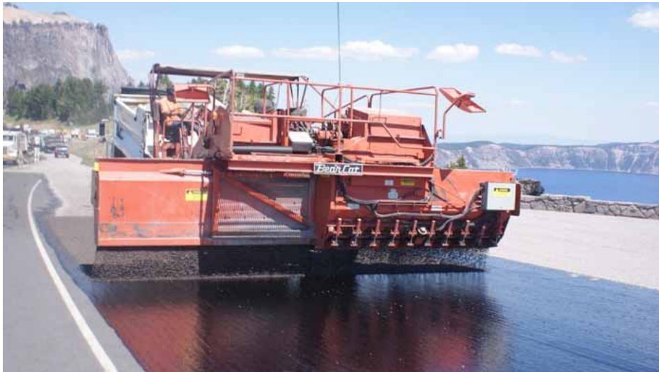
Figure 46. Photo. Crater Lake Project Chip Seal Application.
