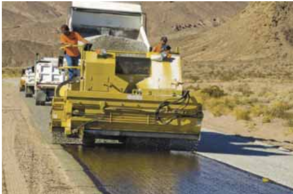
Figure 43. Photo. Death Valley Project—Chip Seal Aggregate Application.
