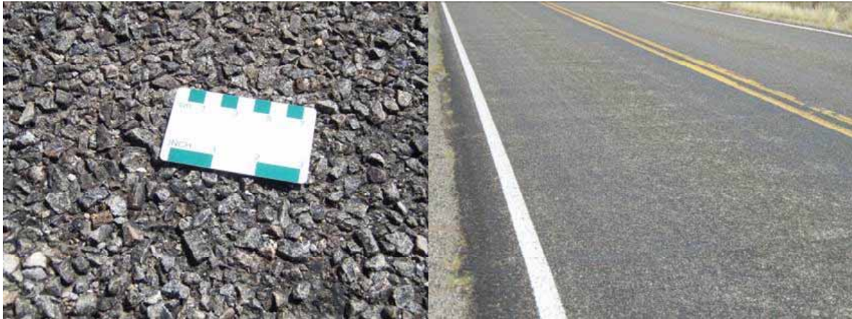
Figure 81. Photo. Arches National Park Chip Seal in July 2009.
