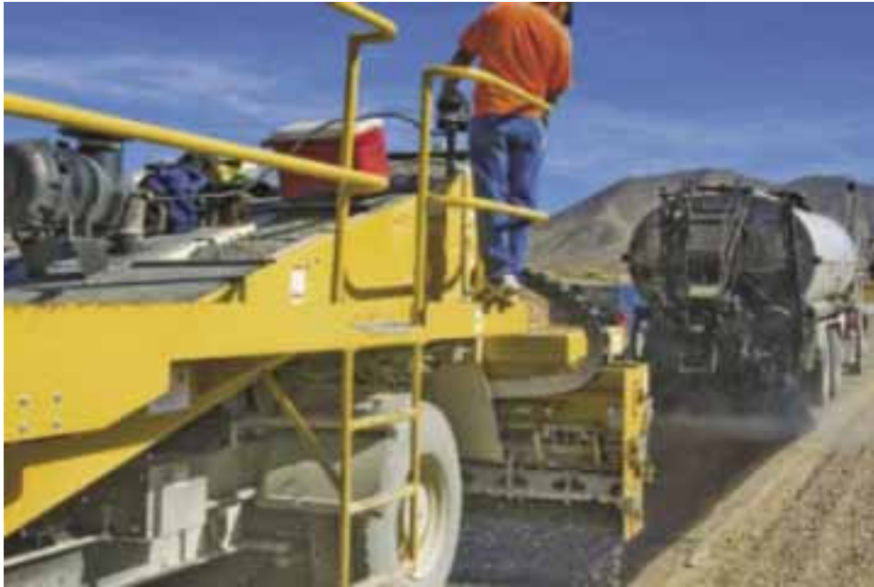
Figure 44. Photo. Death Valley Project—Chip Seal Construction.
