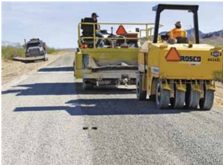
Figure 45. Photo. Death Valley Project—Rolling the Chip Seal.
