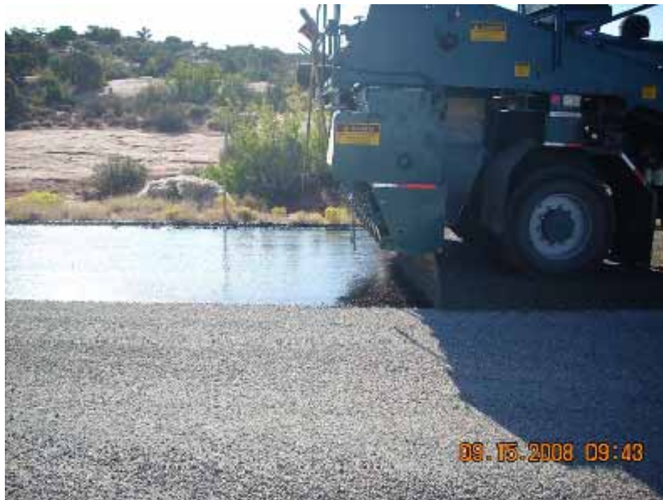
Figure 37. Photo. Utah Parks Project—Canyonlands NP Chip Seal Chip Application.
