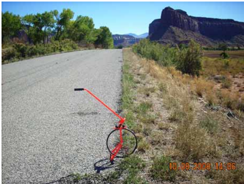
Figure 41. Photo. Utah Parks Project—Natural Bridges National Monument Chip Seal.
