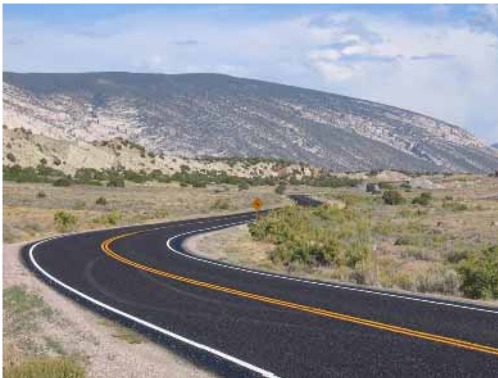
Figure 33. Photo. Dinosaur Project—Route 10 after Completion.
