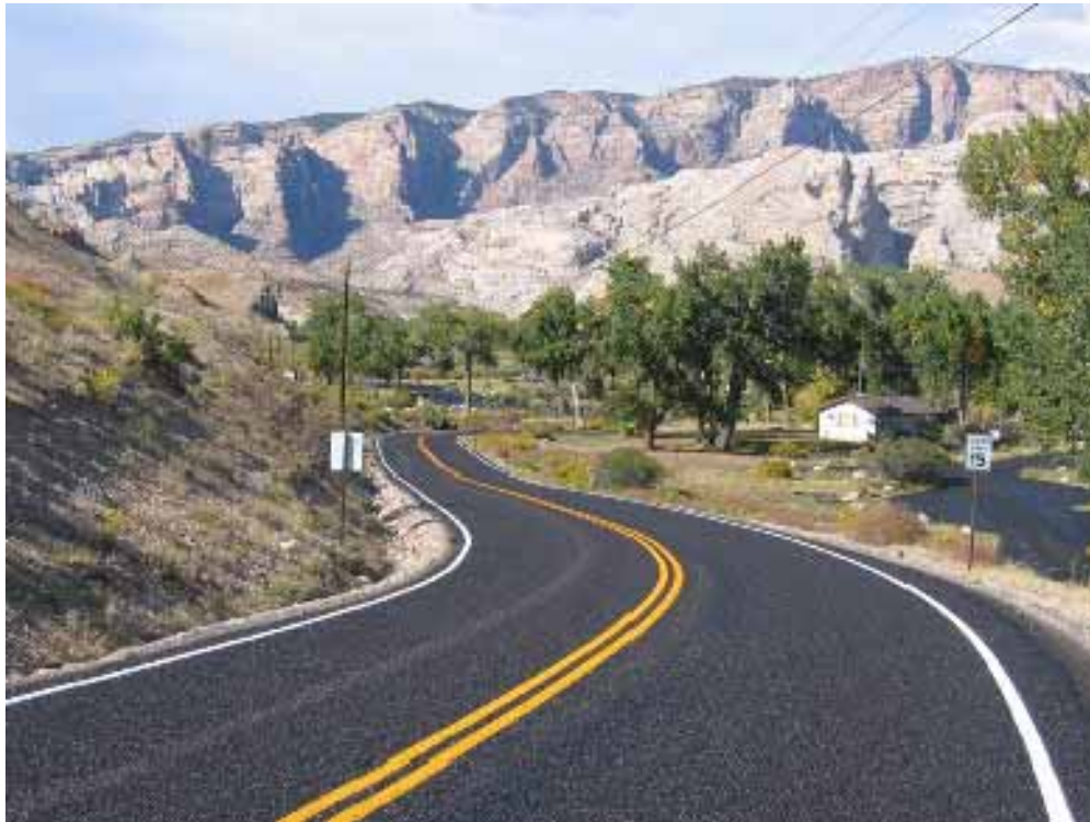
Figure 32. Photo. Dinosaur Project—Green River Access Road after Completion.
