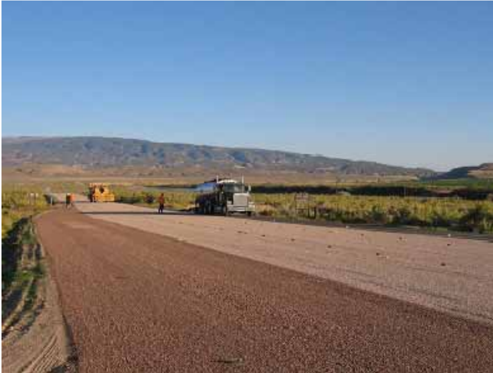
Figure 30. Photo. Dinosaur Project—Pay Station Chipsealing.
