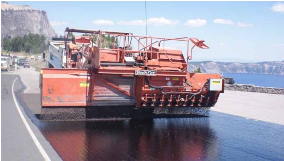
Figure 46. Photo. Crater Lake Project Chip Seal Application.
