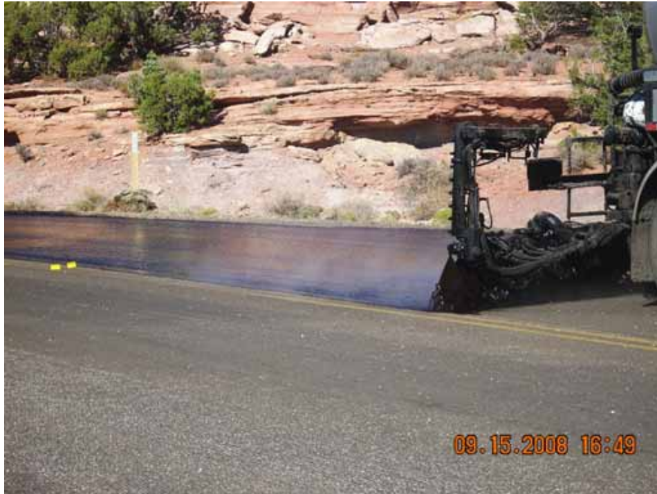
Figure 36. Photo. Utah Parks Project—Canyonlands NP Chip Seal Emulsion Application.
