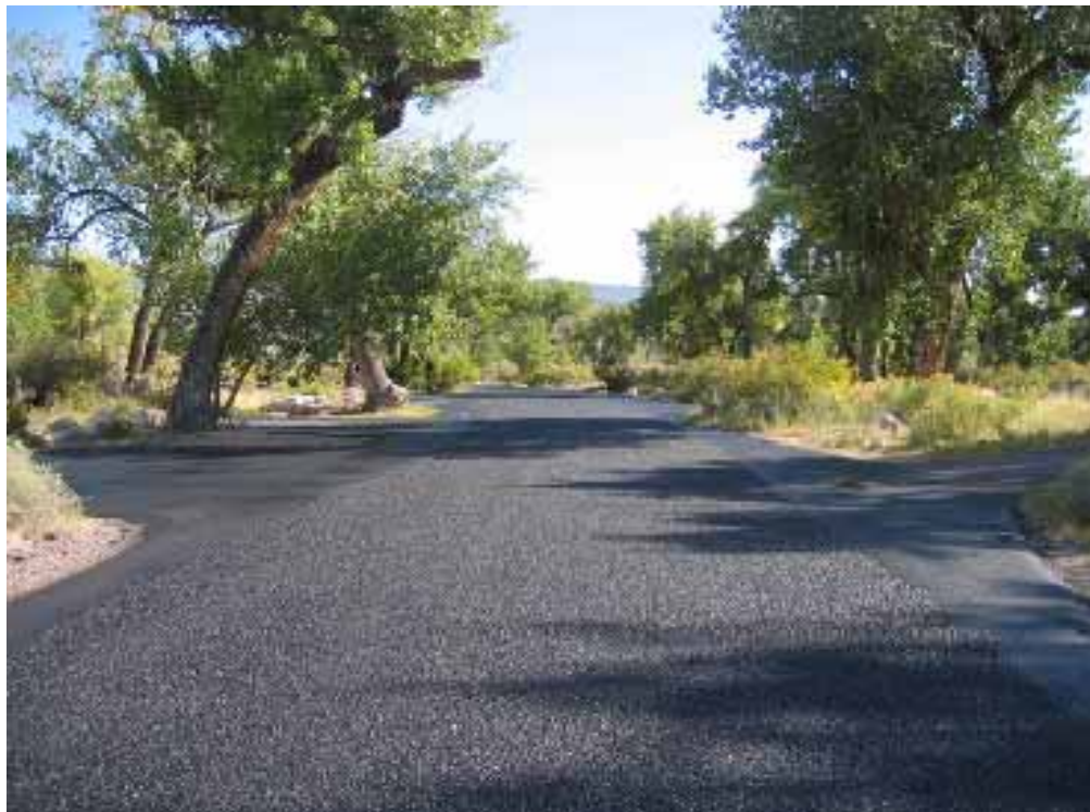
Figure 31. Photo. Dinosaur Project—Loop ‘B’ After Completion.
