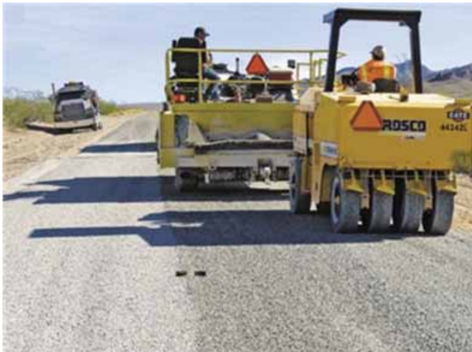
Figure 45. Photo. Death Valley Project—Rolling the Chip Seal.
