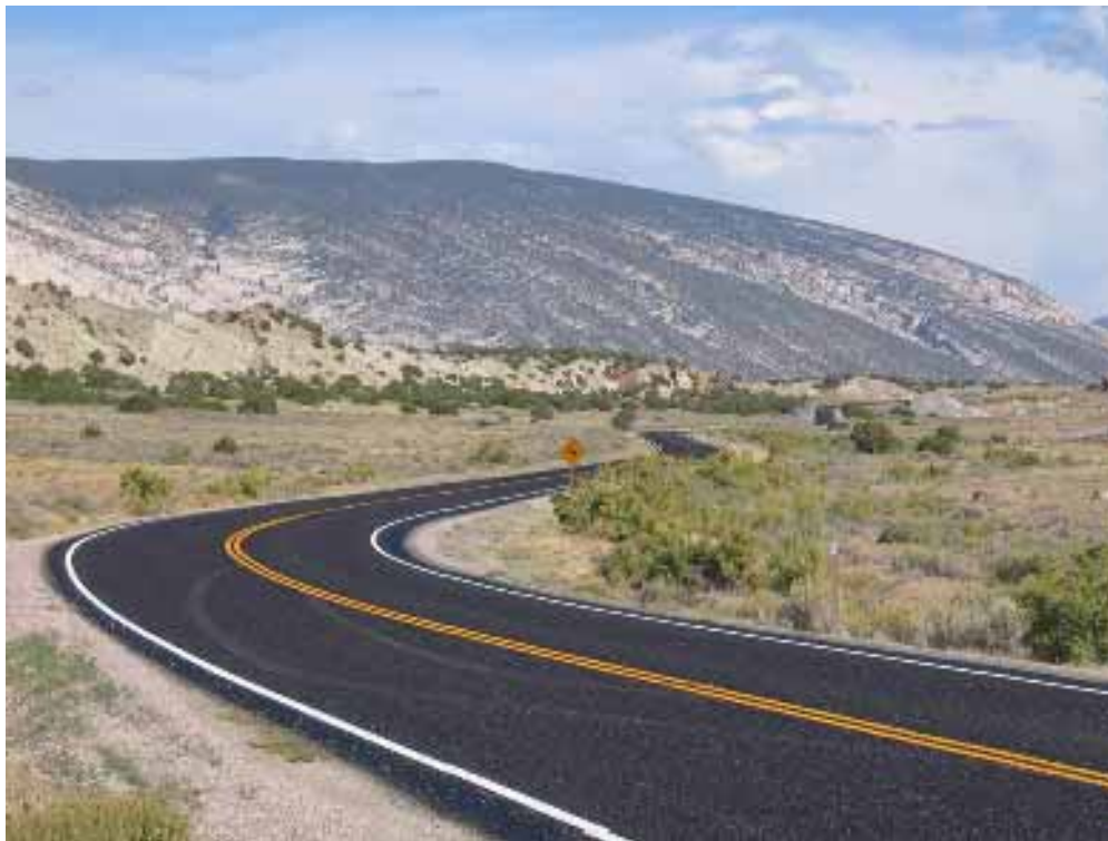
Figure 33. Photo. Dinosaur Project—Route 10 after Completion.
