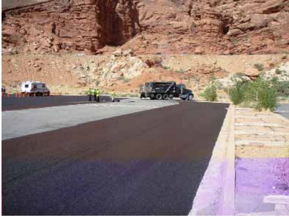
Figure 34. Photo. Utah Parks Project—Micro Surfacing at Arches National Park.
