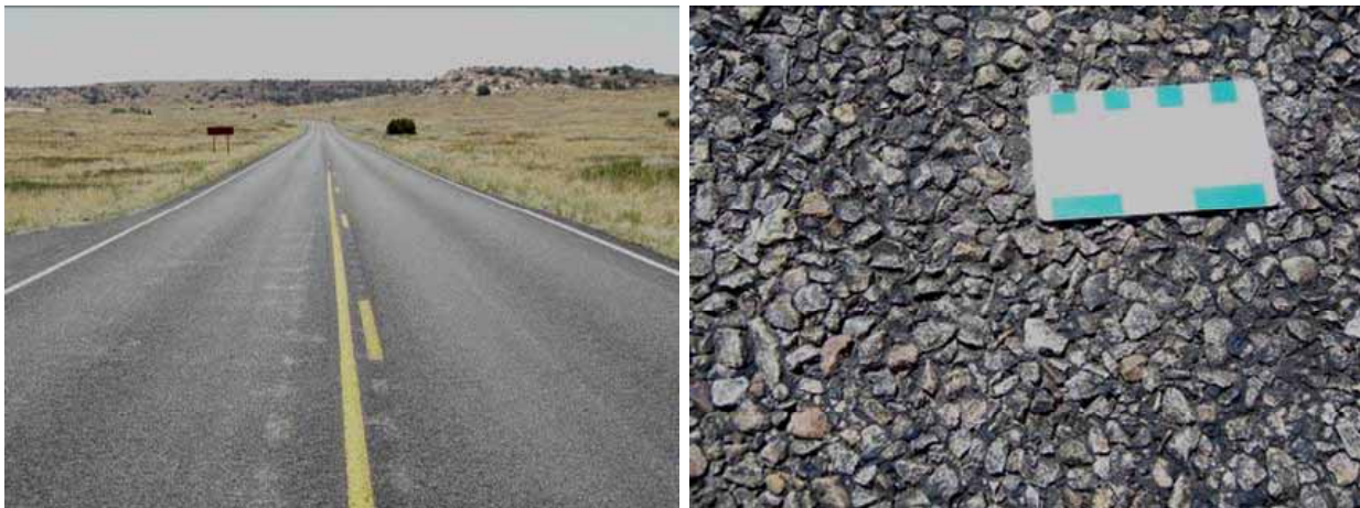
Figure 82. Photo. Canyonlands National Park Chip Seal in July 2009.
