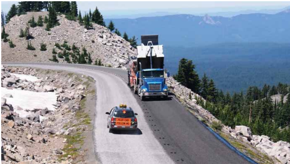
Figure 49. Photo. Crater Lake Project Construction and Traffic Control.
