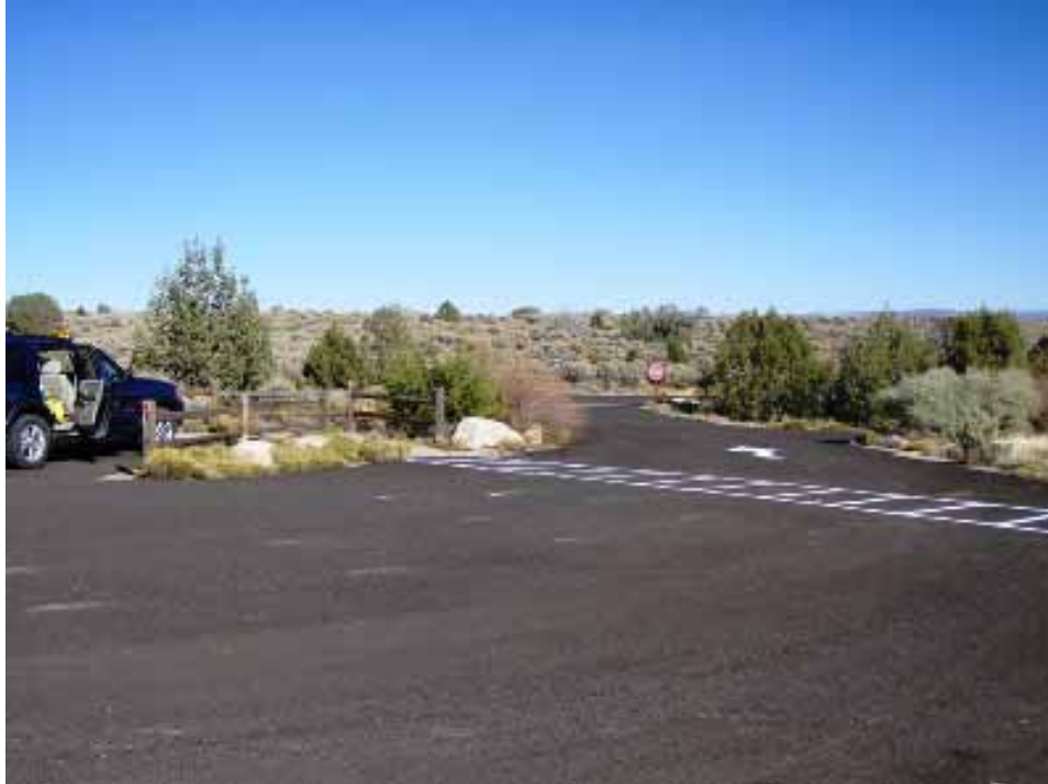
Figure 40. Photo. Utah Parks Project—Hovenweep National Monument Micro Surfacing.
