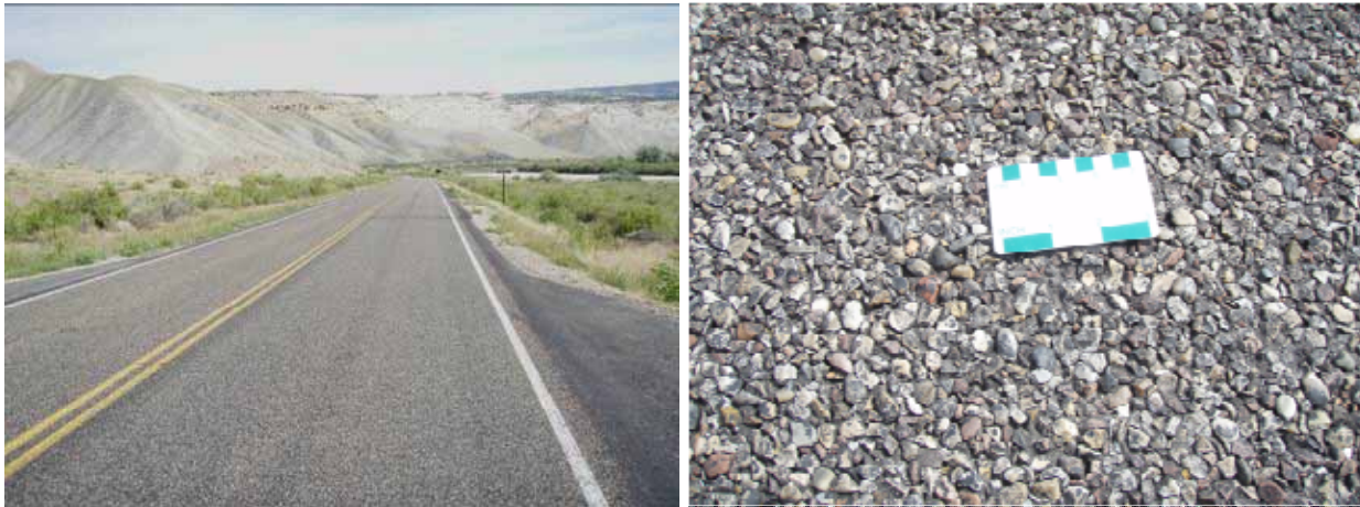
Figure 85. Photo. Dinosaur National Monument PASS Chip Seal in July 2009.
