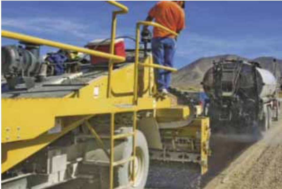
Figure 44. Photo. Death Valley Project—Chip Seal Construction.
