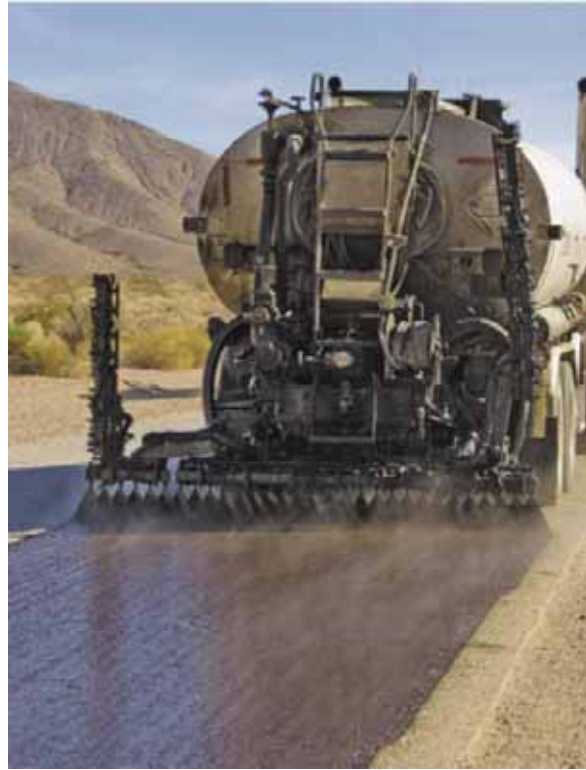
Figure 42. Photo. Death Valley Project—Chip Seal Emulsion Application.
