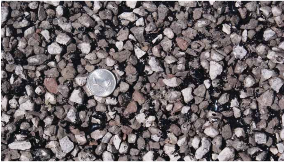
Figure 48. Photo. Crater Lake Project Chip Seal Texture.
