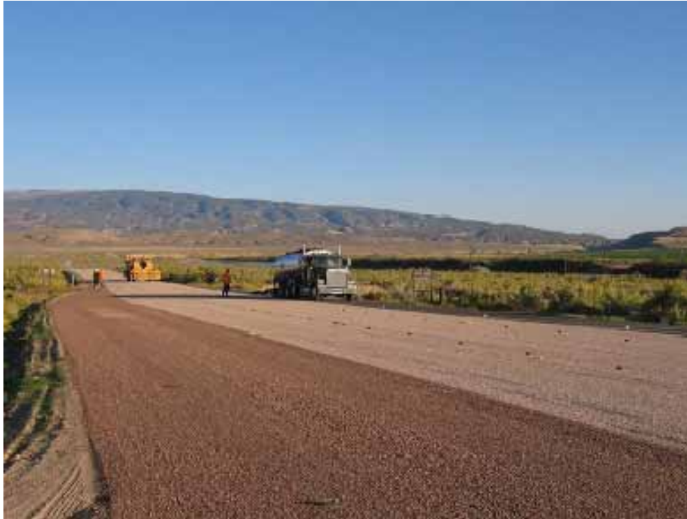
Figure 30. Photo. Dinosaur Project—Pay Station Chipsealing.
