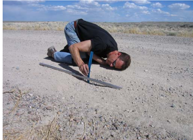
Figure 23. Photo. Measuring Pothole Depth.
