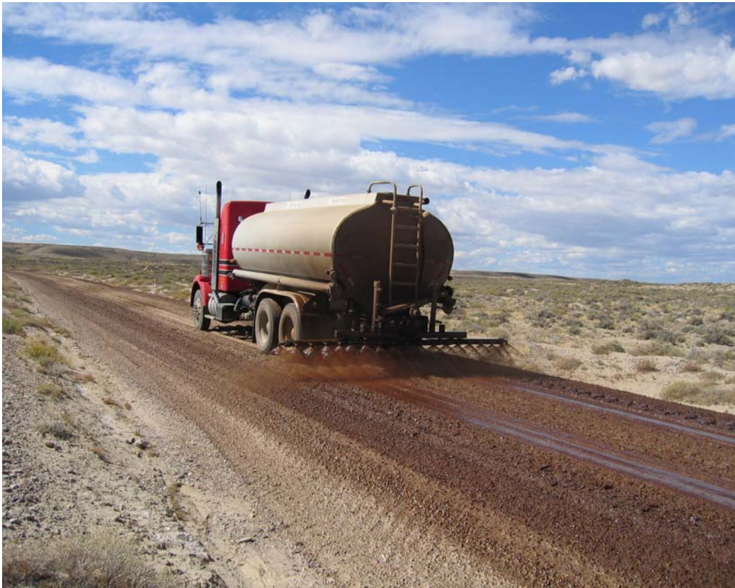
Figure 7. Photo. Distribute truck applying DMC-820 Ligno/Mag to Section VI.
