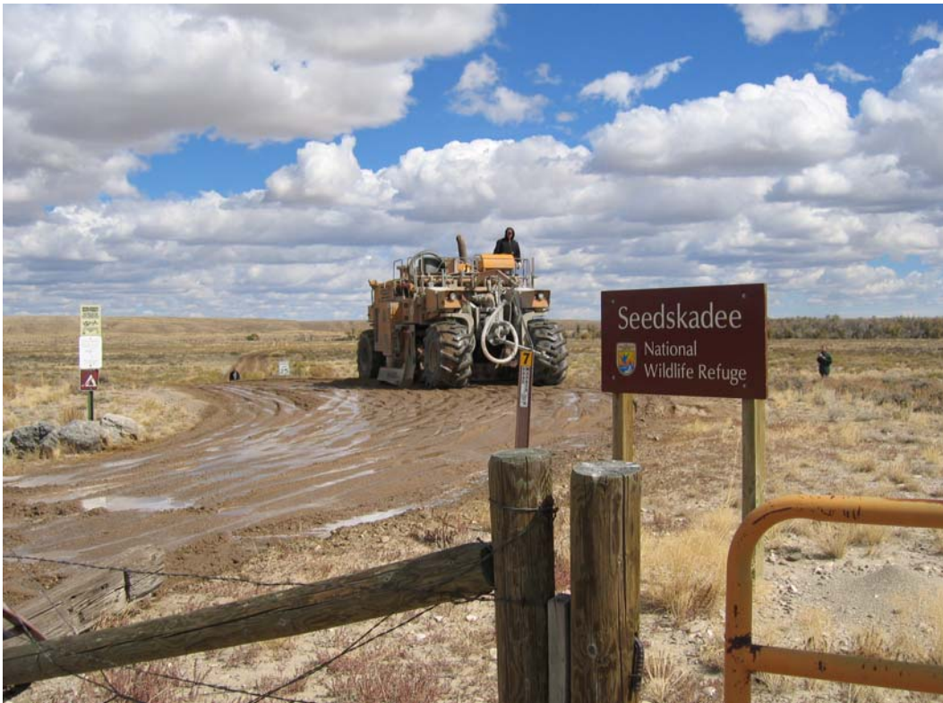
Figure 6. Photo. 650 CMI pulverizer mixing Caliber product into Section V.
