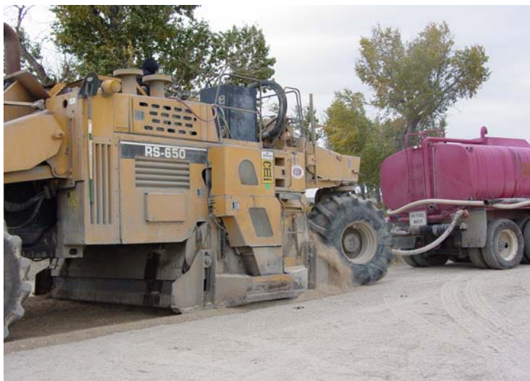
Figure 4. Photo. CMI 650 pulverizer following water truck.
