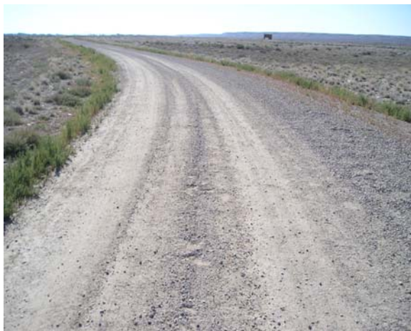
Figure 13. Photo. Raveling.
