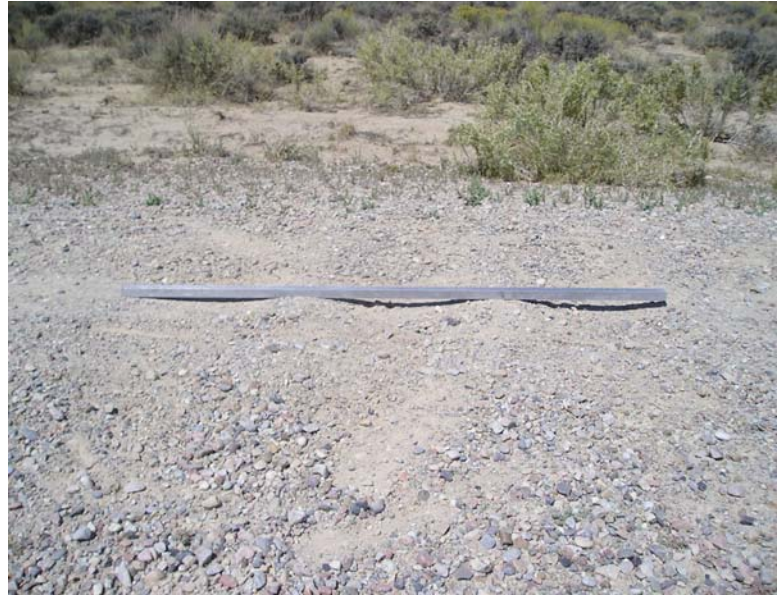
Figure 19. Photo. Measuring washboarding depths.
