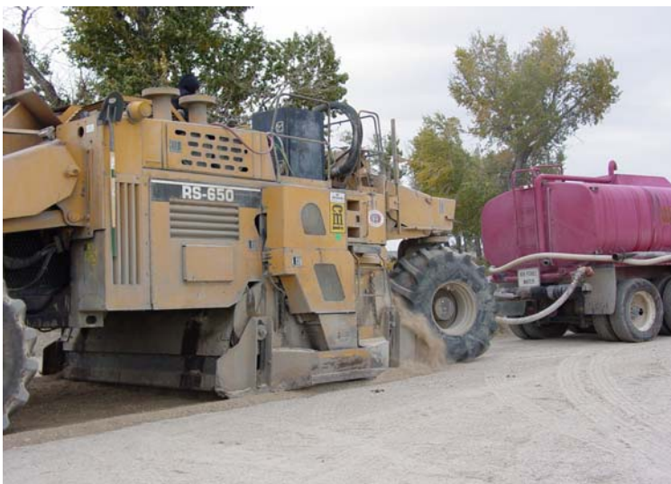
Figure 4. Photo. CMI 650 pulverizer following water truck.
