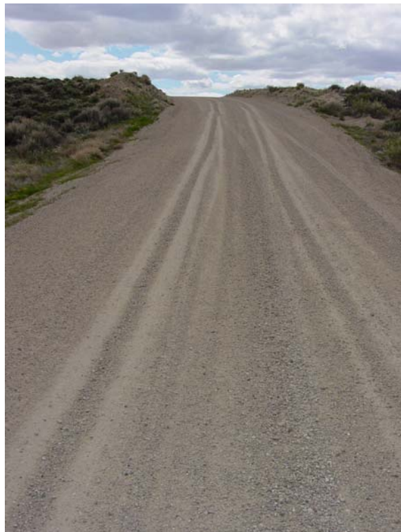
Figure 14. Photo. May 2005 ruts in PermaZyme Section III.
