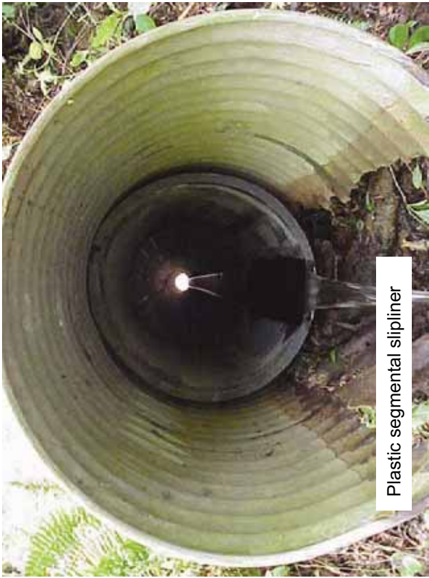
CMP liner in CMP host pipe with grouted annulus
