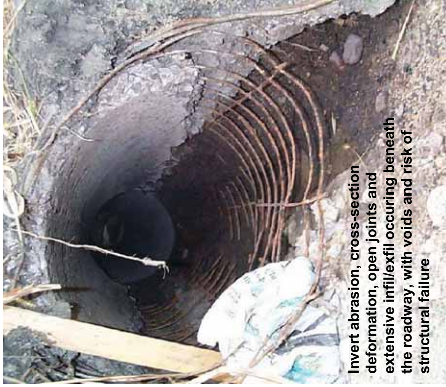
Very poor joint with significant soil infill and sinkholes likely beneath roadway and risk of structural failure
