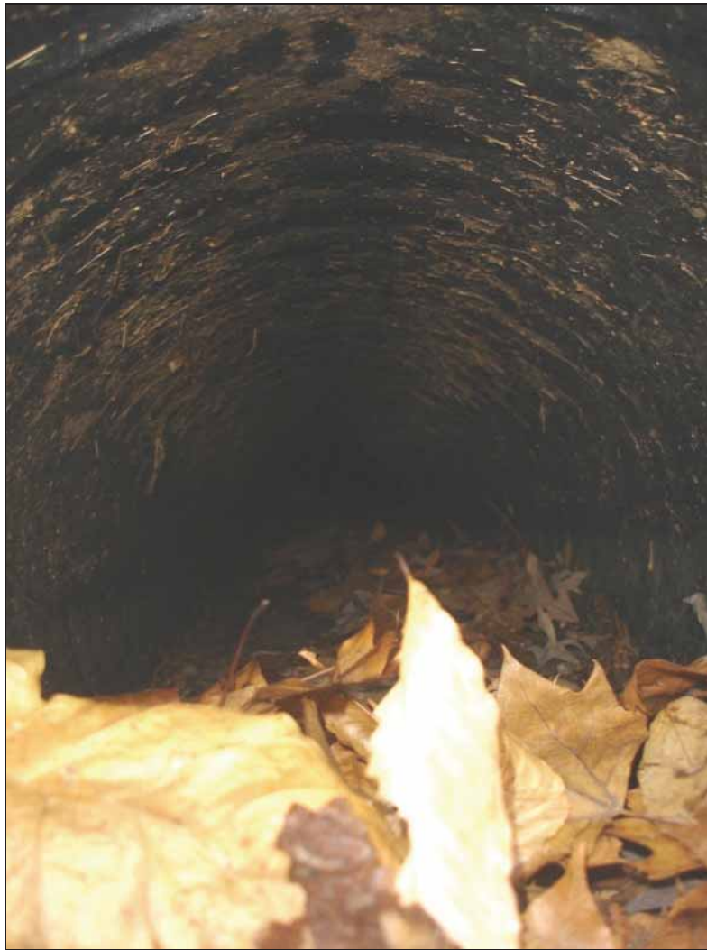
Figure 56. Photo. View of interior of plastic example in Fountainhead Park showing clogging.
