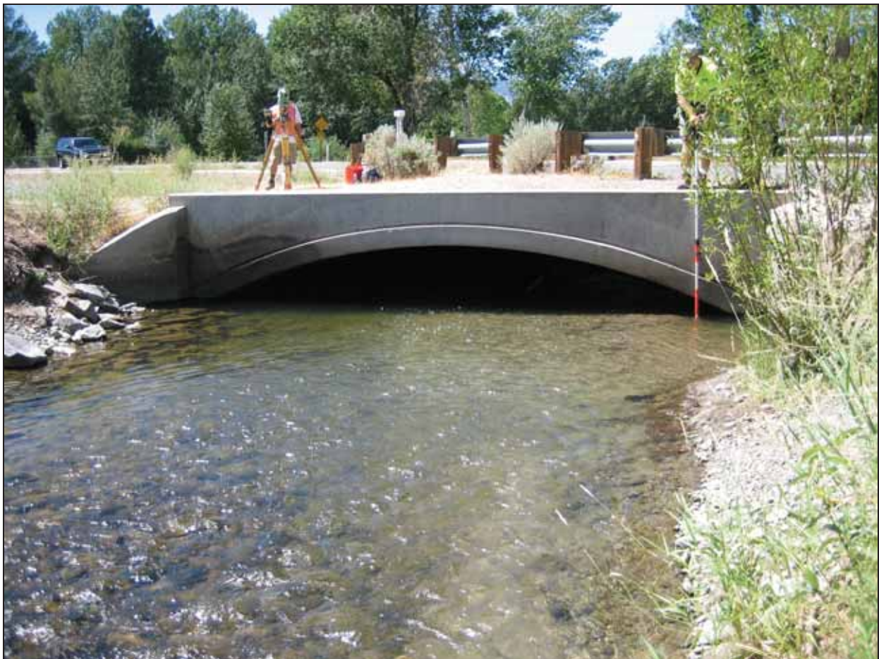
Figure 15. Photo. Example of an open-bottom culvert.
