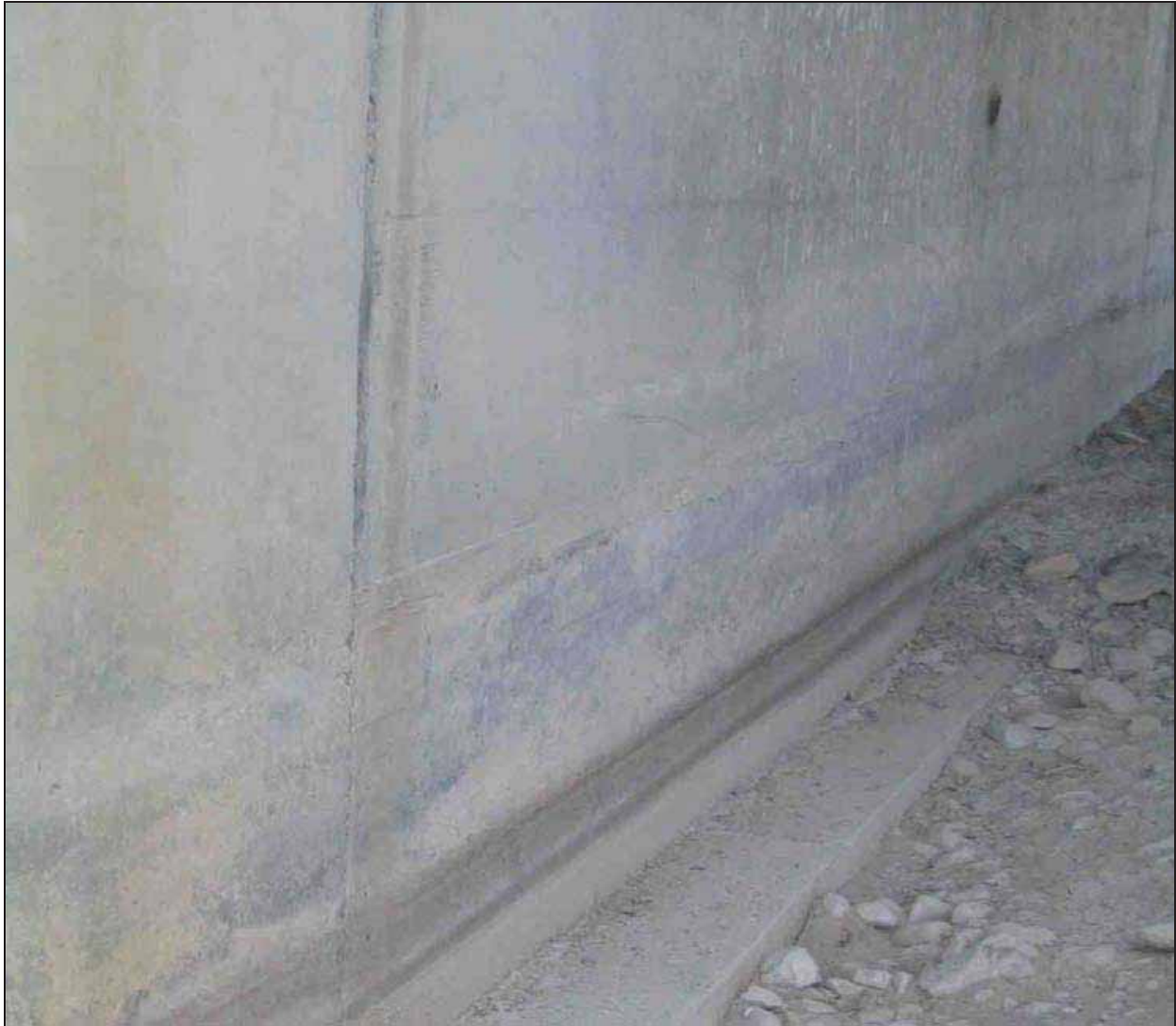
Figure 16. Photo. Exposed spread footing condition possible in an open-bottom culvert.
