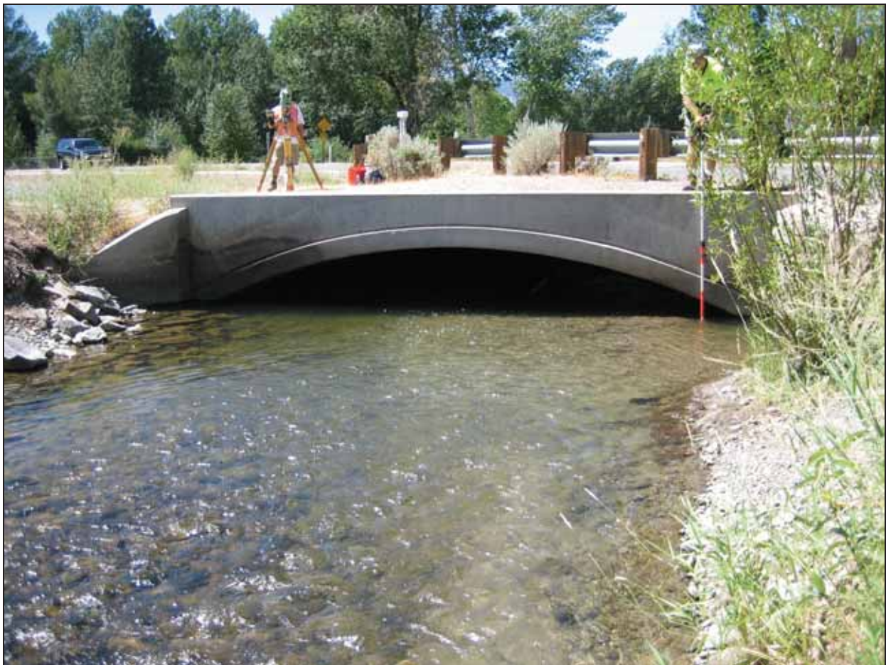
Figure 15. Photo. Example of an open-bottom culvert.
