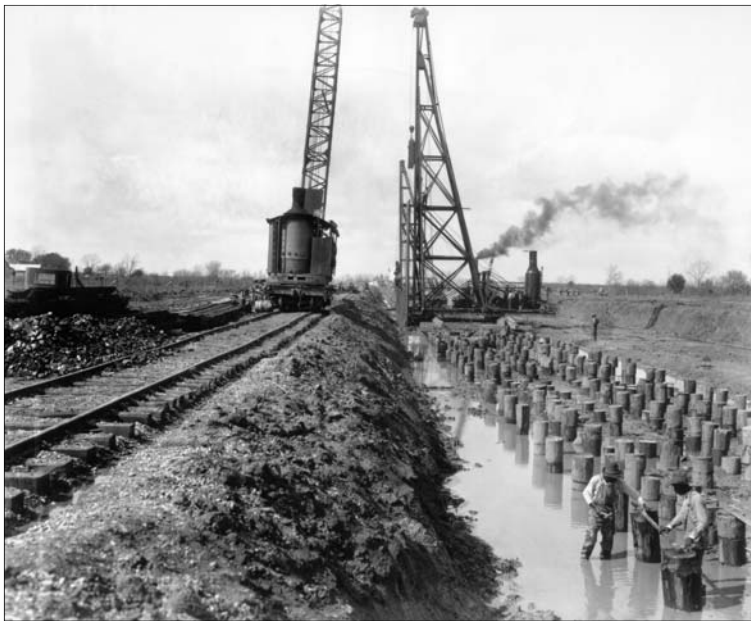
Construction of the Bonnet Carré Spillway, 1929
