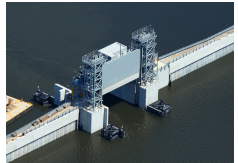
Above: View of the 56-foot-wide vertical lift gate at Bayou Bienvenue. (USACE photograph)
