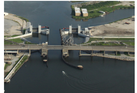
Above: Aerial image of the completed Seabrook Floodgate Complex. (USACE photograph)
