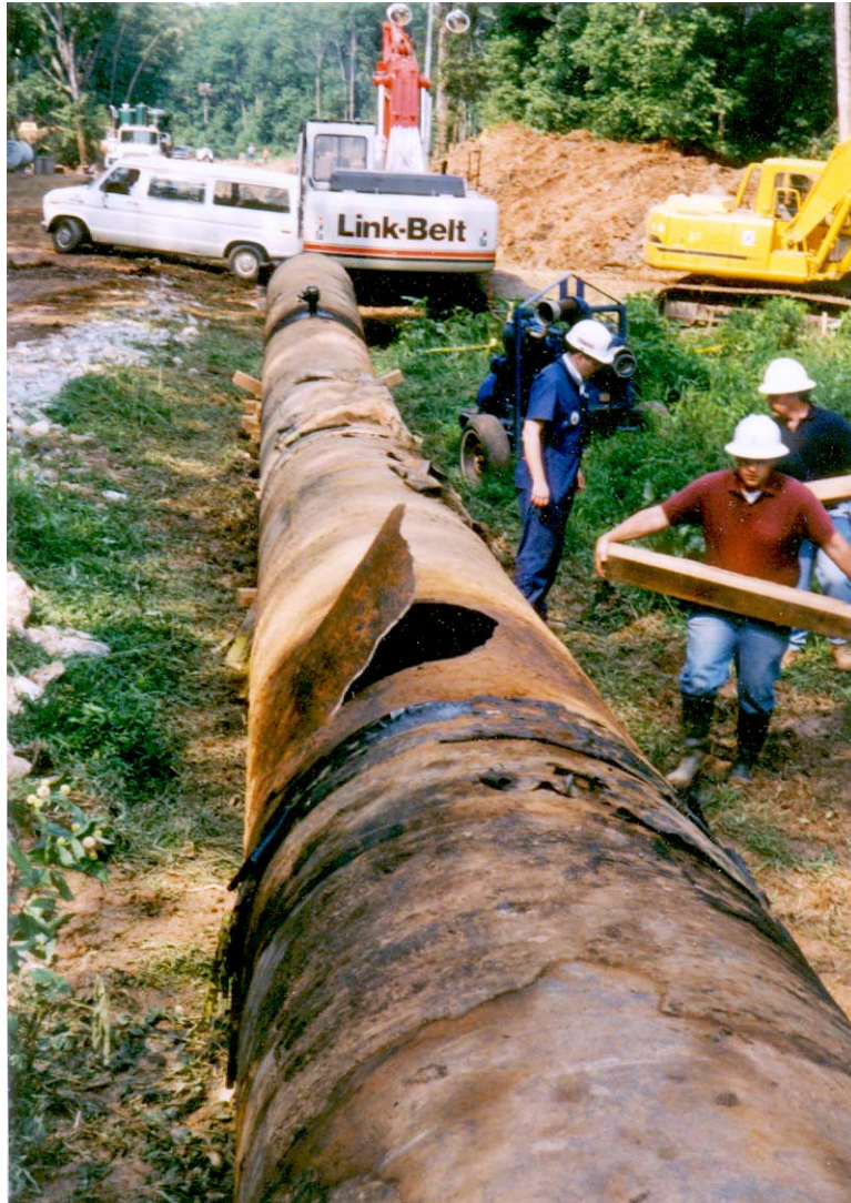
Figure 2. Ruptured pipe after removal from Reedy River
