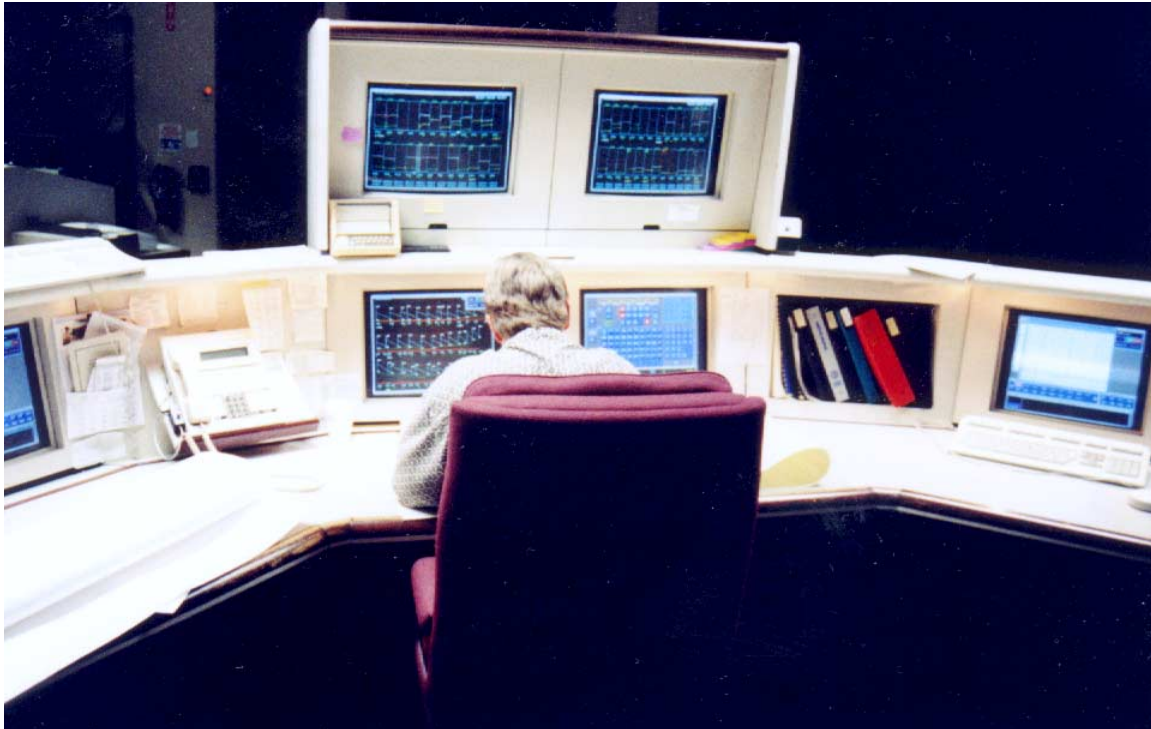
Figure 3. Work station from which controllers monitored and operated line No. 2
