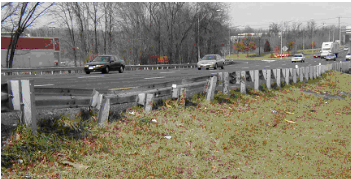
Figure 12. Backside of the southbound guardrail.
