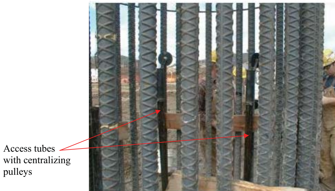
Figure 3. Photo. Rebar Cage and CSL Tubes of Completed Drilled Shaft.
