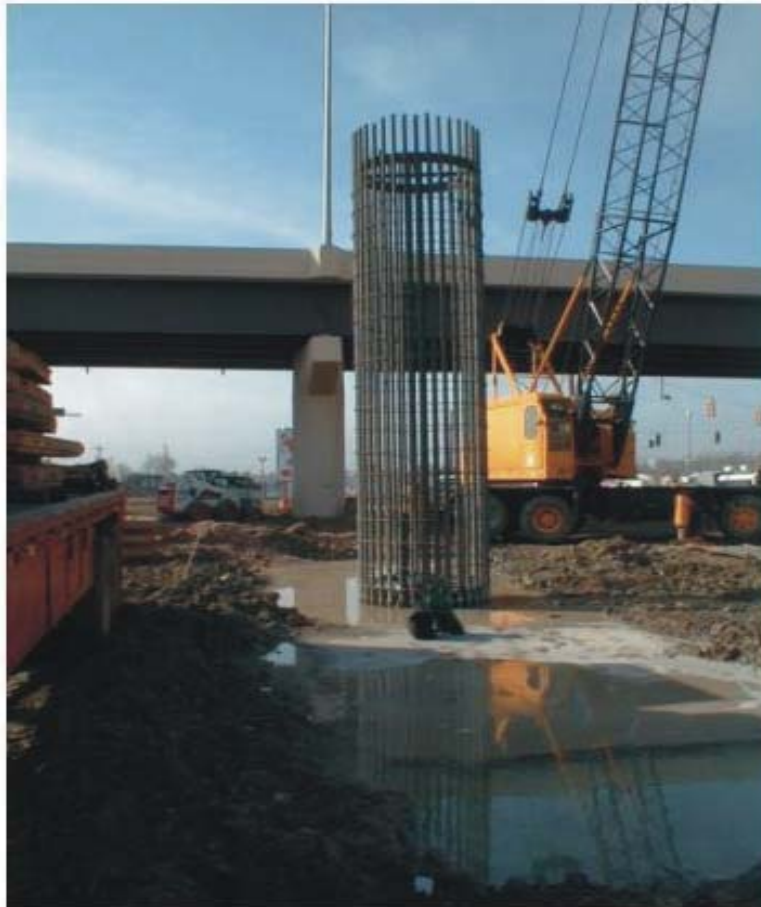
Figure 2. Photo. Drilled Shaft Construction.
