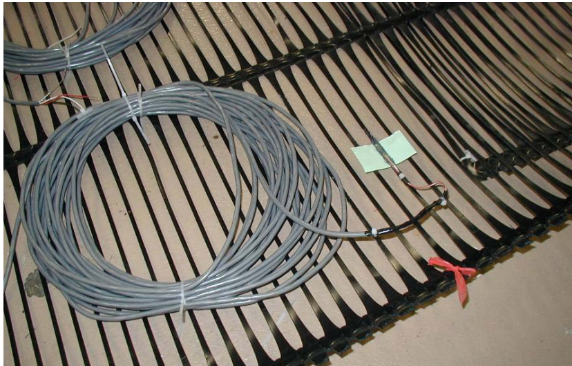
Figure 52. Photo. Strain gage installed on uniaxial geogrid.
