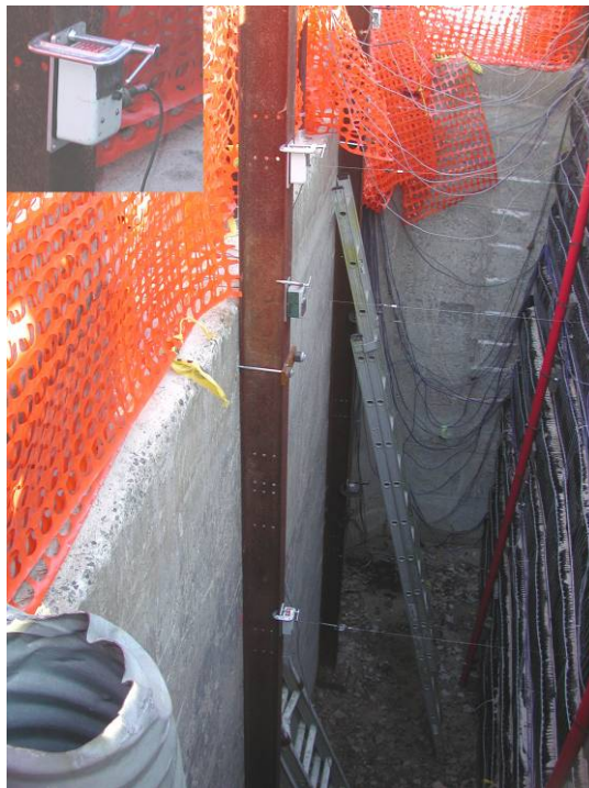
Figure 57. Photo. Potentiometer installation showing connection to vertical reference.
