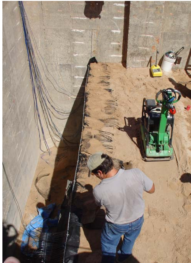
Figure 45. Photo. Reinforced fill compaction and retained fill placement.
