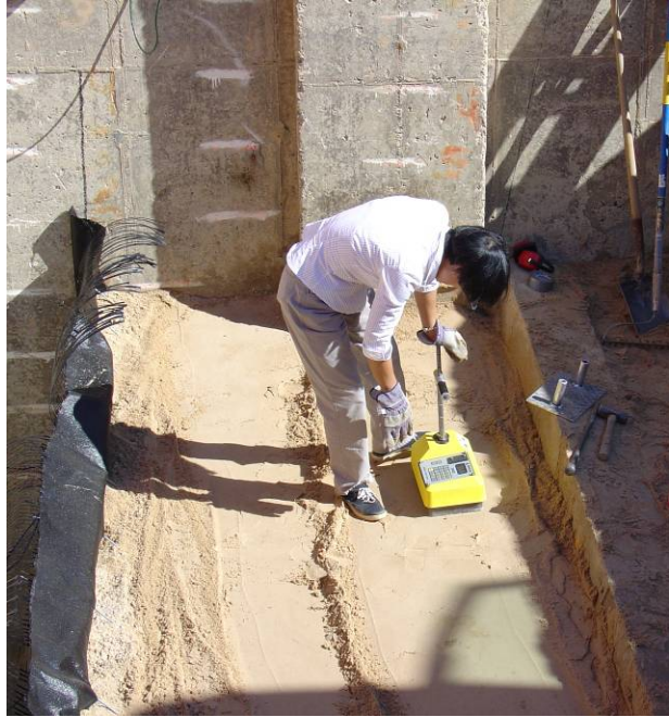
Figure 46. Photo. Nuclear density gage testing of reinforced fill zone.
