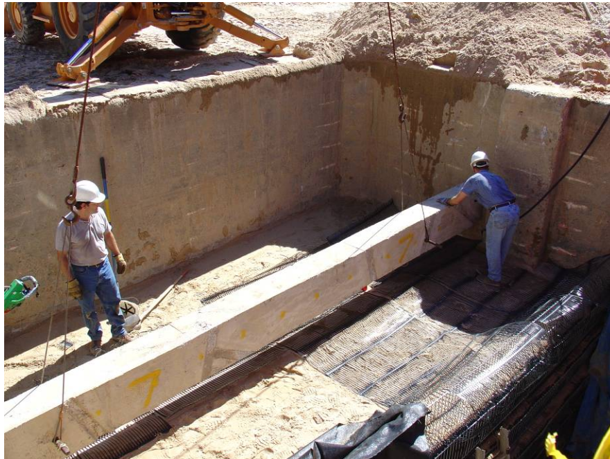
Figure 48. Photo. Installation of shoring beam.
