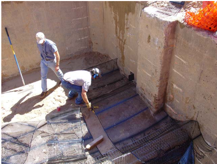
Figure 50. Photo. Geogrid installation.
