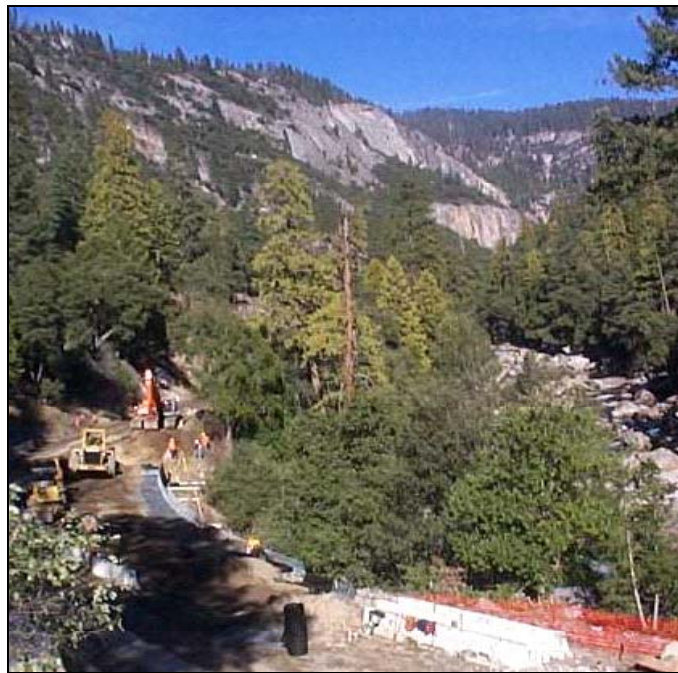
Figure 3. Photo. El Portal Road re-construction.
