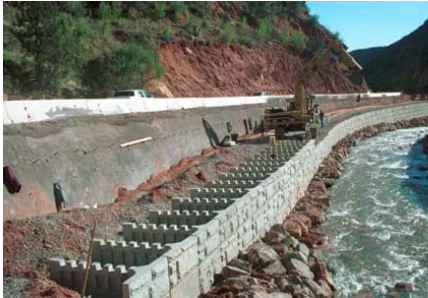
Figure 4. Photo. Compound wall construction at Zion National Park.
