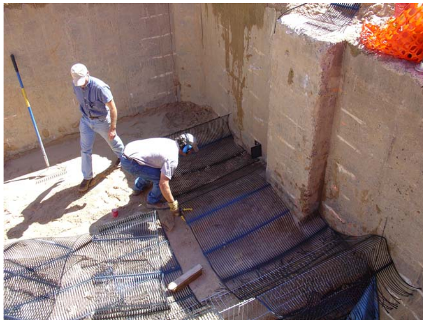
Figure 50. Photo. Geogrid installation.
