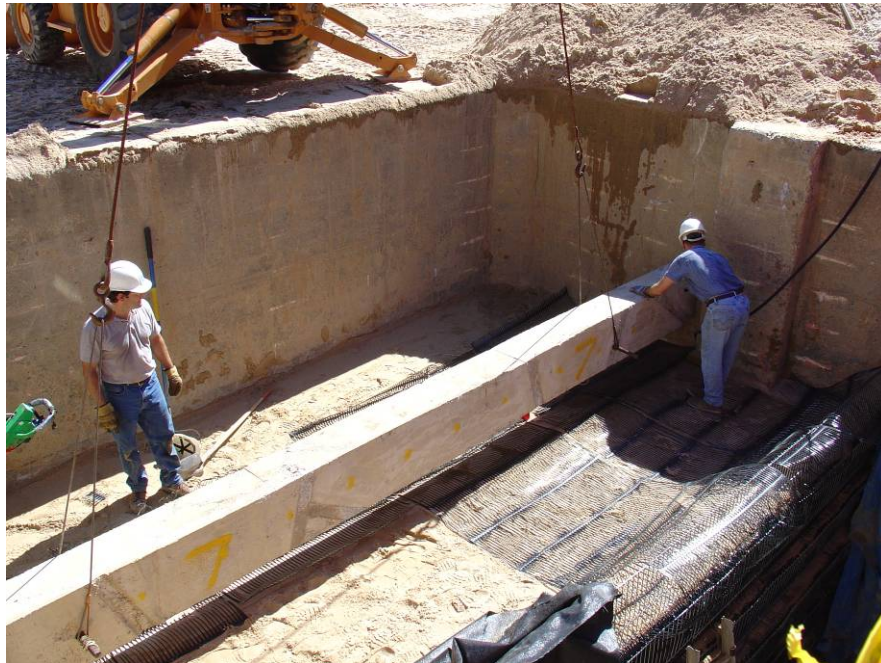
Figure 48. Photo. Installation of shoring beam.
