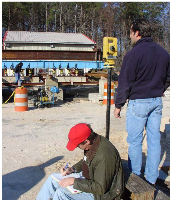
Figure 55. Photo. Total station surveying of footing deflection.
