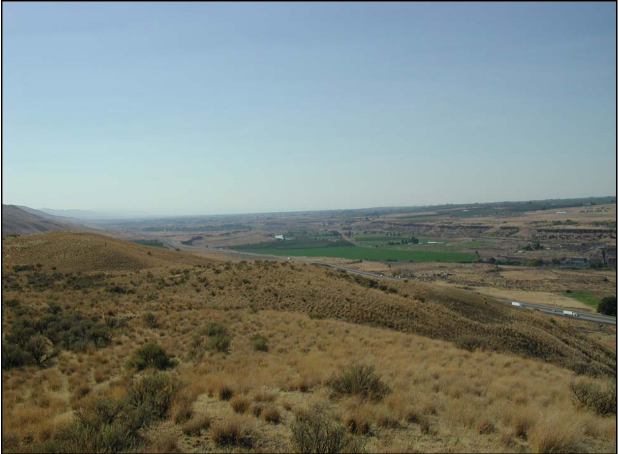
Figure 11. Photo. Site of historical road deformation along Interstate-82 near Benton City.
