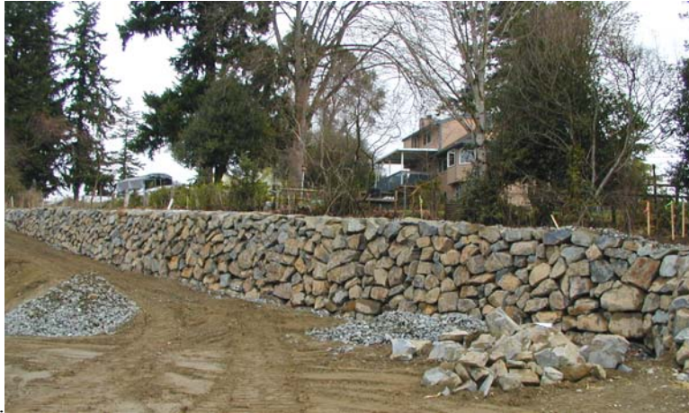
Figure 11. Photograph. Single-tier, 3-m (10-ft) rockery, Military Road at Enchanted Parkway, Federal Way, Washington (Site 1).
