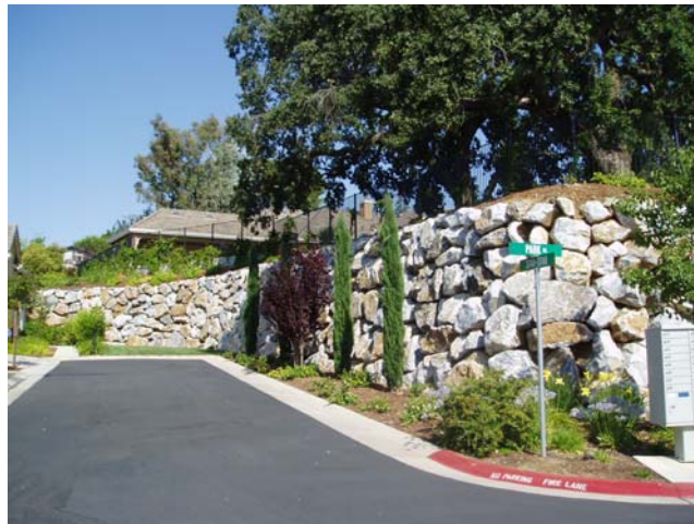
Figure 19. Photograph. Single-tier rockery constructed in cut condition, El Dorado Hills, California (2001).
