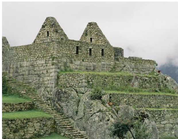
Figure 4. Photograph. Rockery construction at Machu Picchu, Peru.
