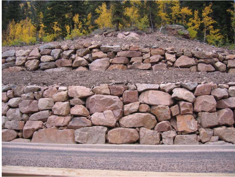
Figure 8. Photograph. Completed rockery for Guanella Pass Road, Colorado, 2005.
