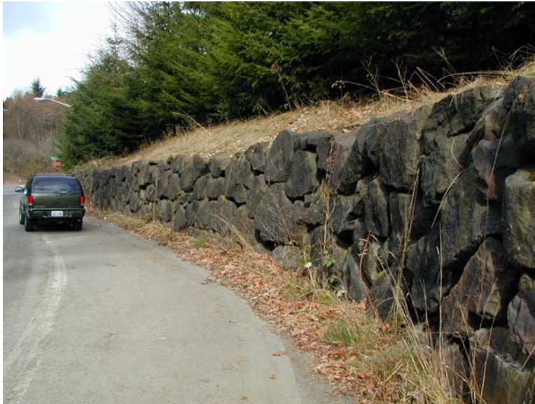
Figure 14. Photograph. Single-tier, 2.4-m (8-ft) rockery, Nisqually National Wildlife Refuge, Washington (Site 4).
