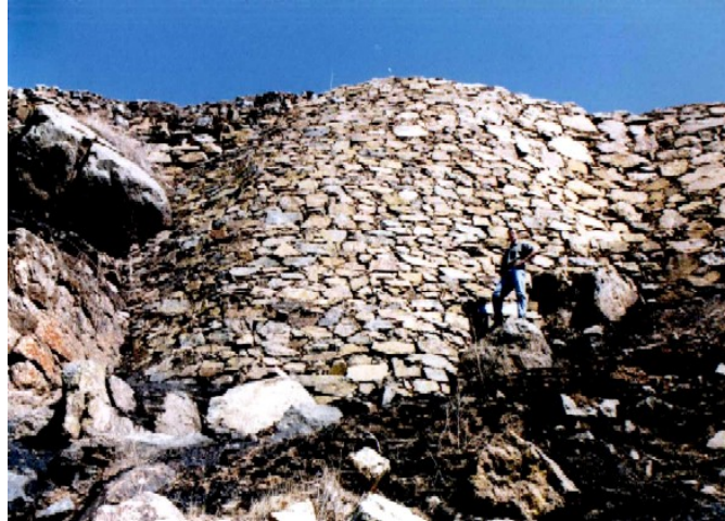
Figure 5. Photograph. Approximately 9.1-m-tall (30-ft-tall) rockery outside La Grange, California, dating from the late 1800s.
